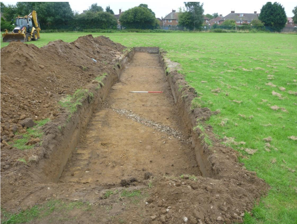
Plate 6 Trench 6 facing south east 1.0m scale
