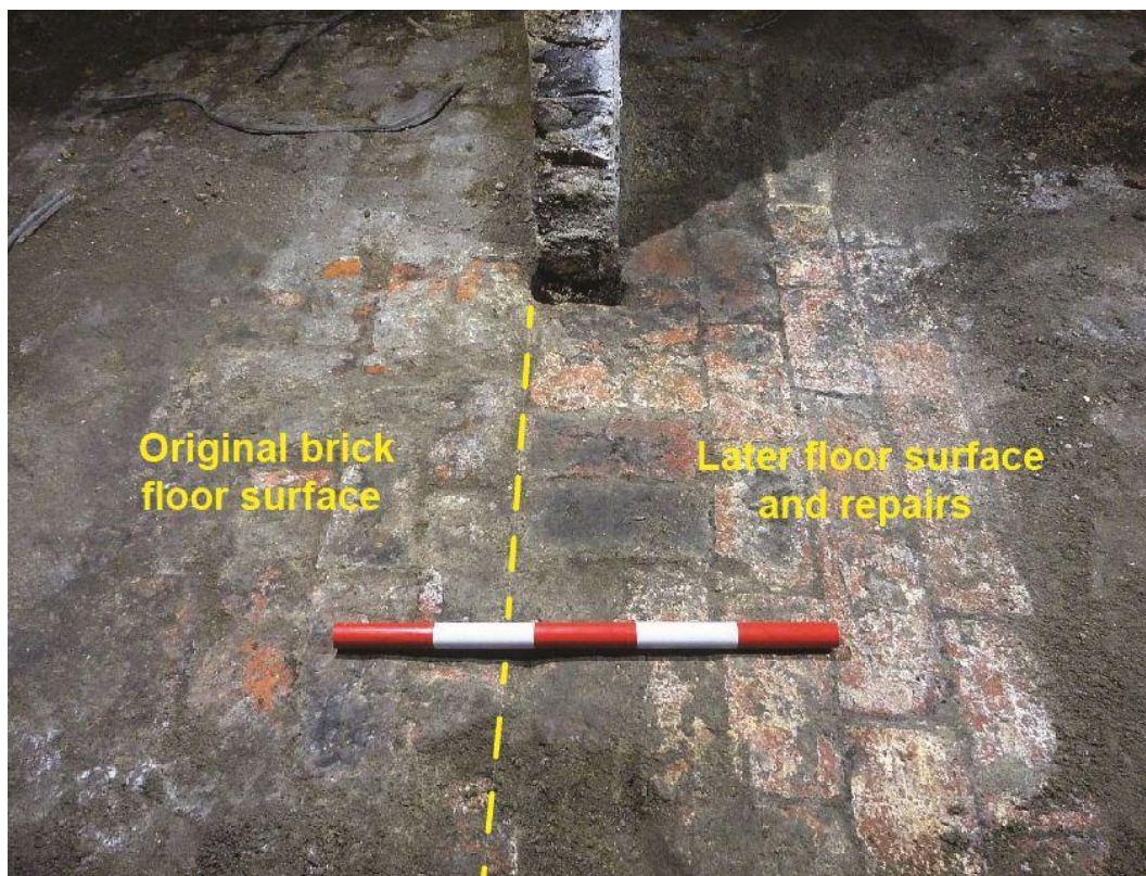
Plate 4 Pre-excitation of brick floors of cellar, view southeast, scale unit: 100mm
