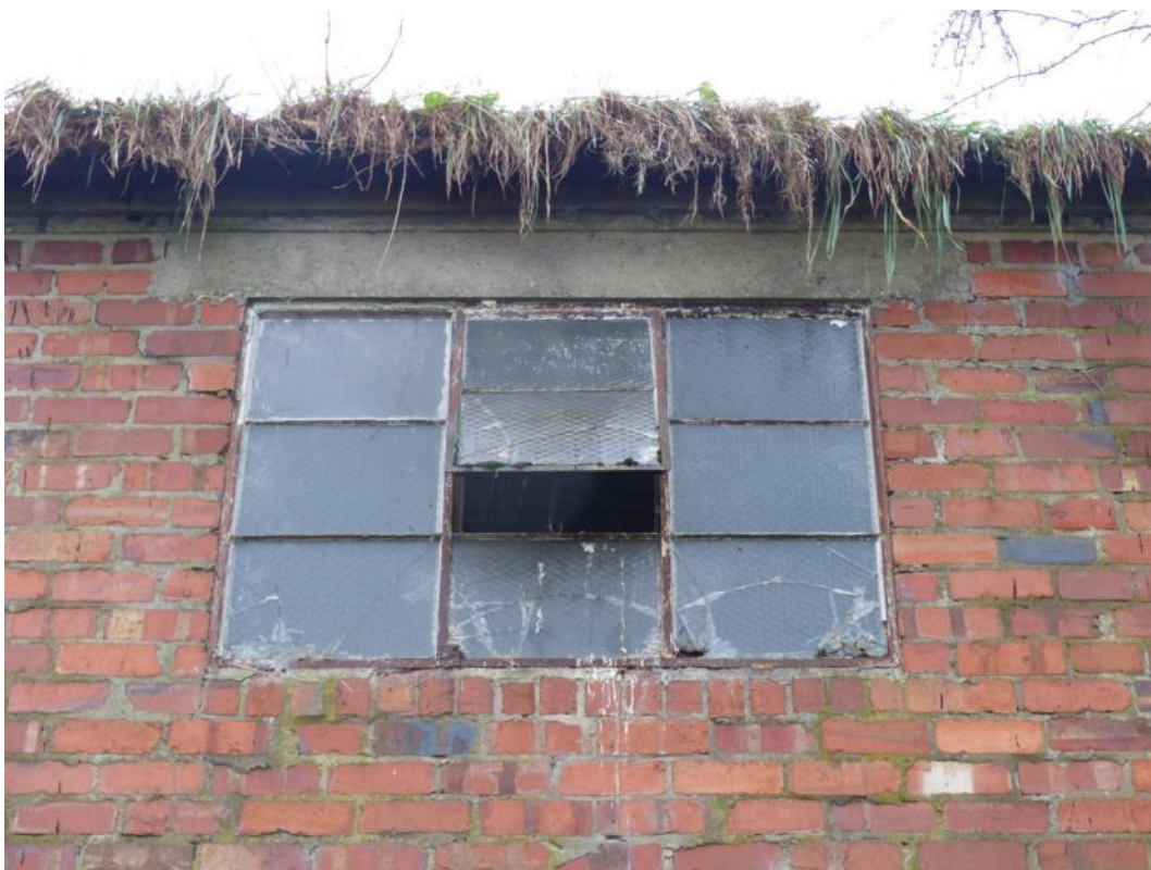
Plate 2: Detail of a window in the former munitions store, looking west
