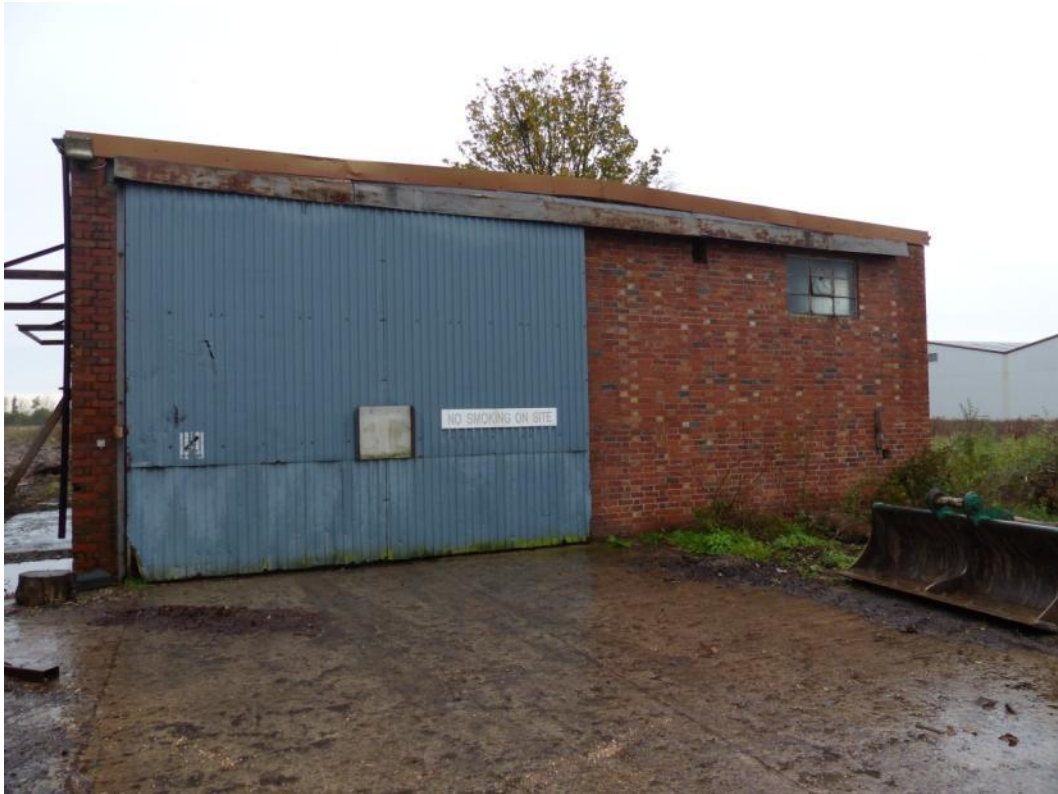
Plate 3: The south elevation of the munitons store, looking northeast
