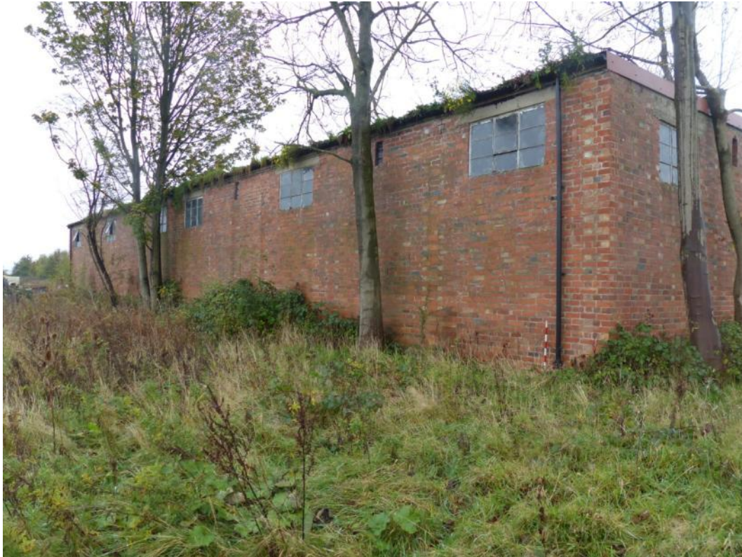
Plate 7: The side (east) elevation of the munitions store, looking southwest
