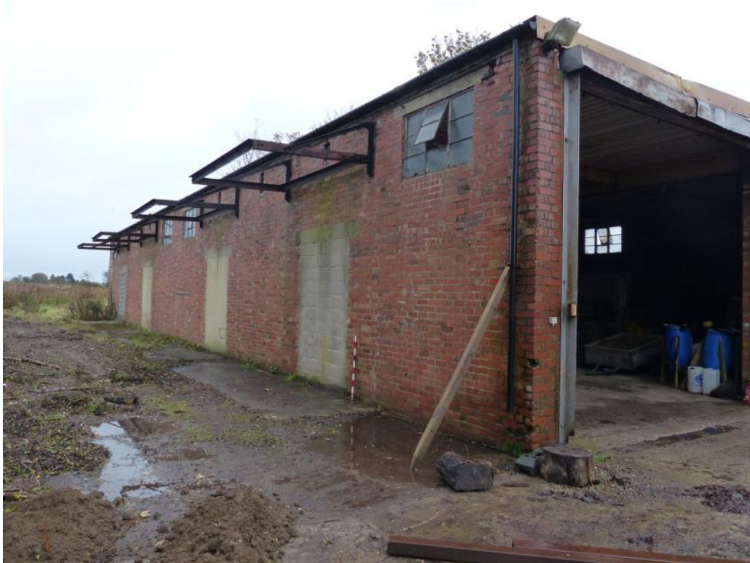
Plate 5: The side (west) elevation of the munitions store, looking northeast
