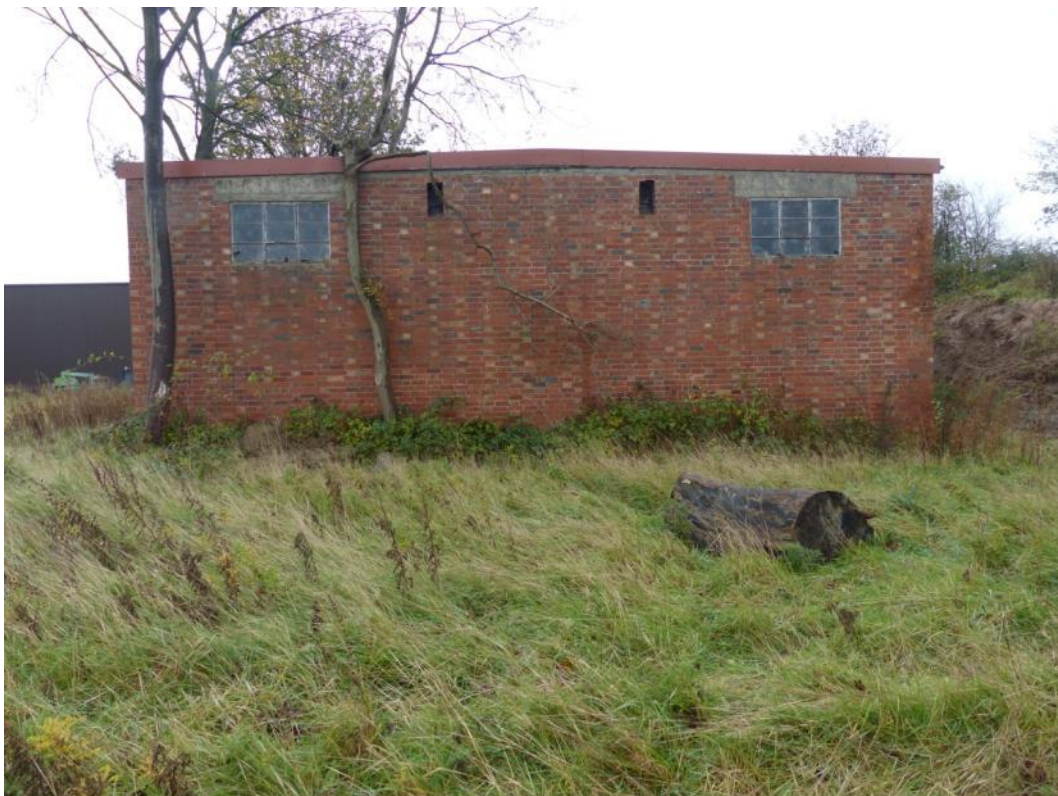
Plate 6: The rear (north) elevation of the munitions store, looking south
