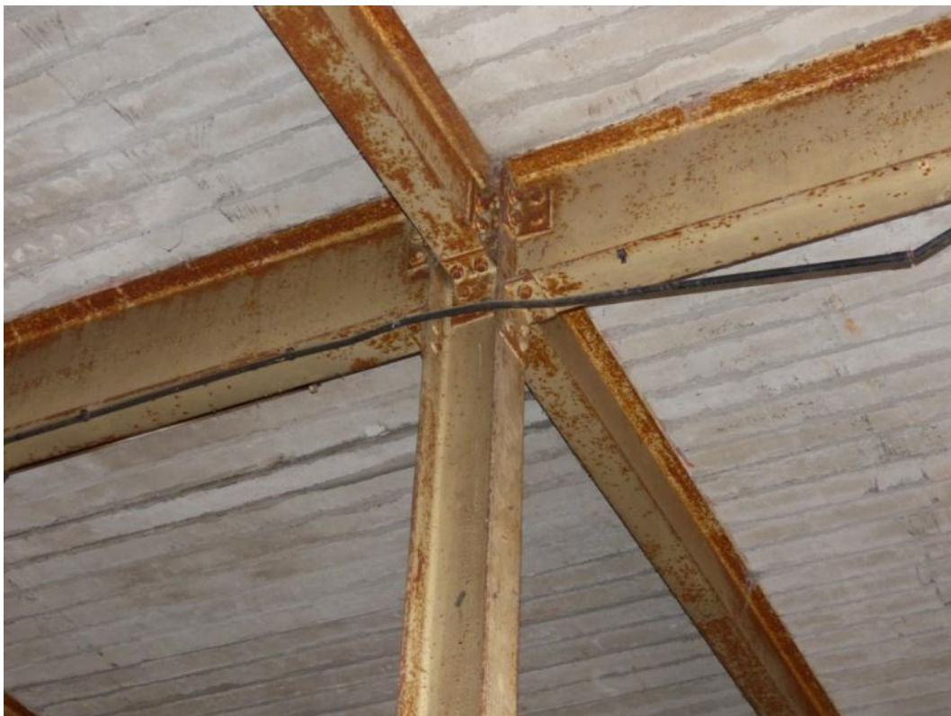
Plate 12: The steel I-beams showing the details of their connections, looking northeast
