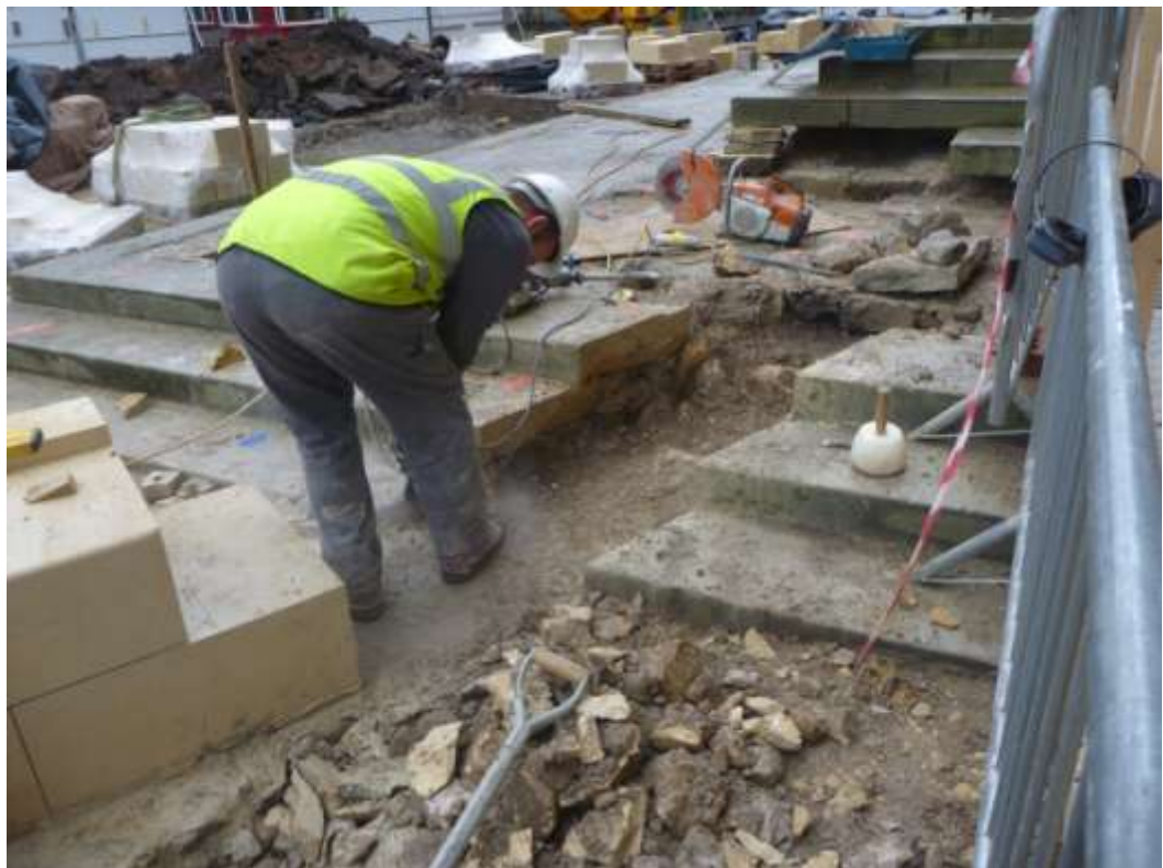
Plate 14 Construction of new ramp wall into 1848 steps, looking south west
