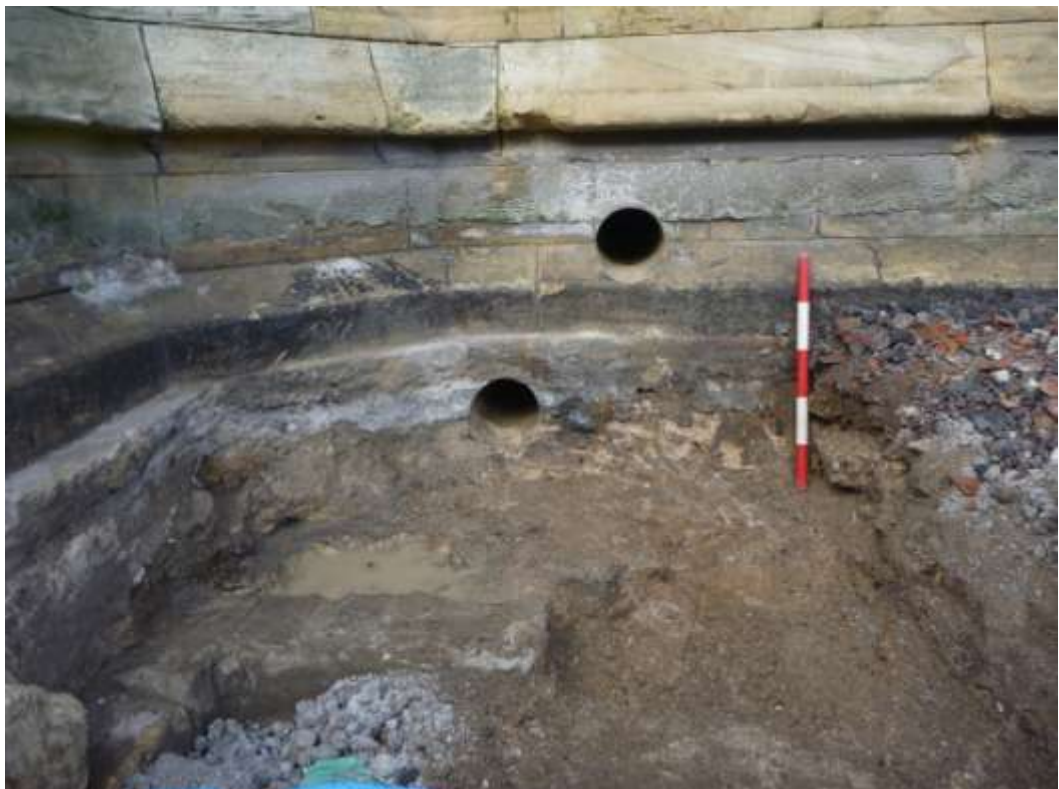
Plate 32 Holes in South Transept south wall for drain in Trench H, looking north
