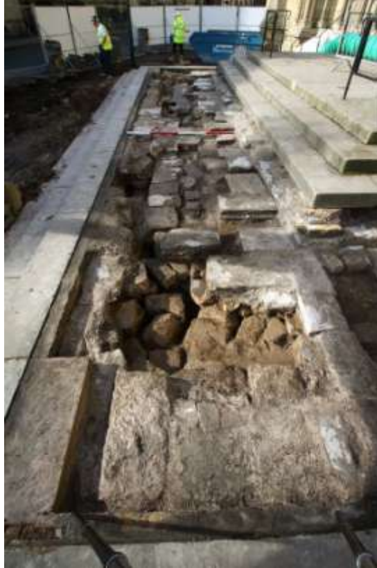
Plate 3 Exposed steps 5006 looking west
