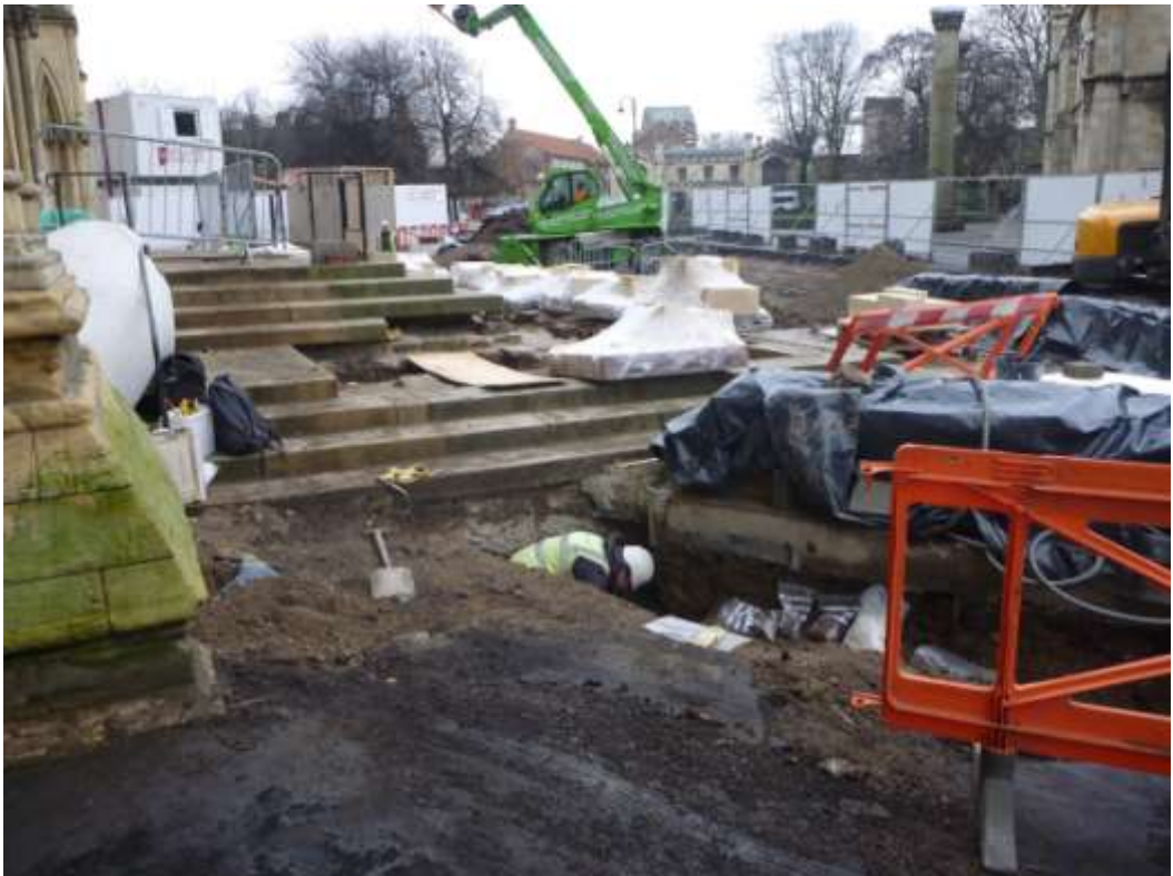
Plate 20 View of Trench A northern end, looking south east
