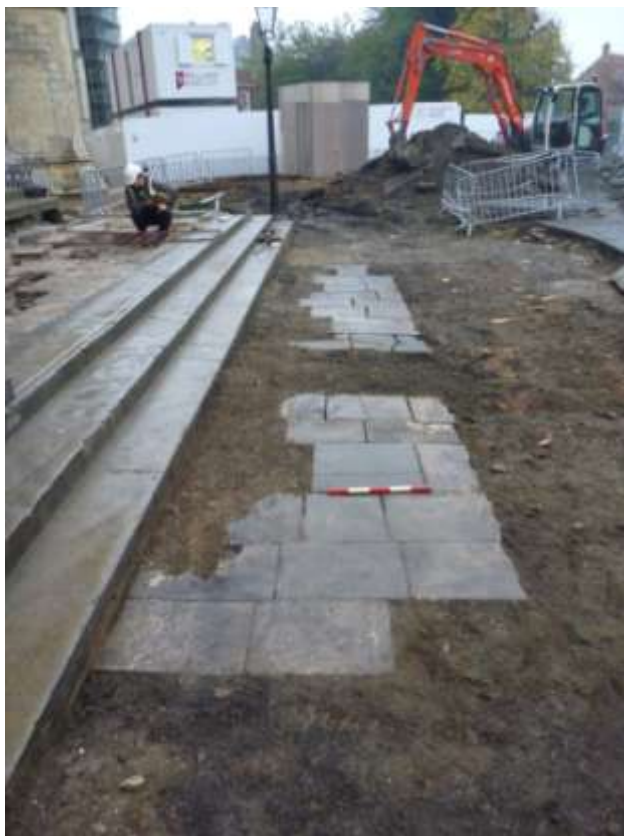
Plate 37 Paving 5052, looking east
