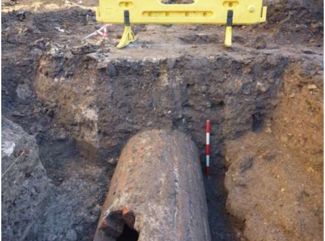
Plate 19 Trench F south-west facing section
