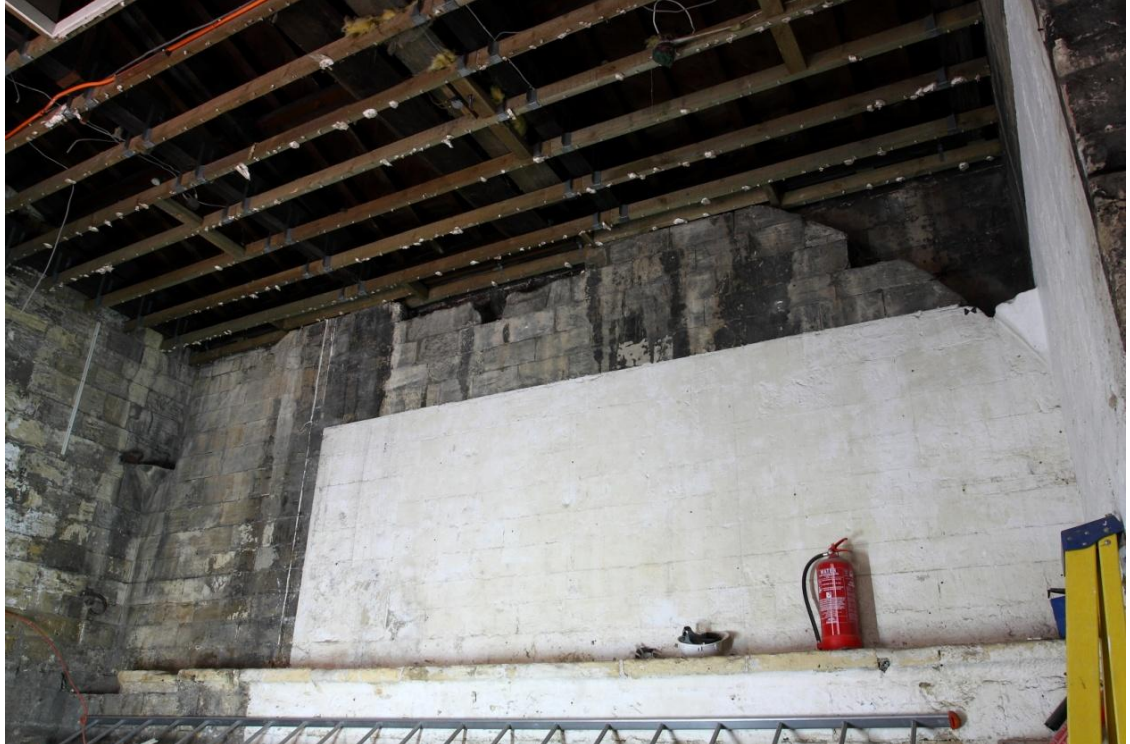
Plate 3 Elements of former range to west of doorways. Note springing corbels, looking SE
