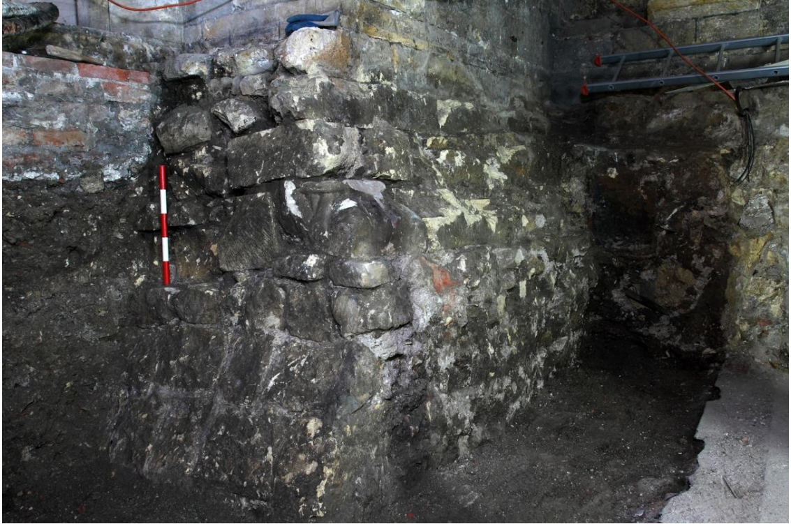
Plate 5 15 th century buttress footing, looking south-east
