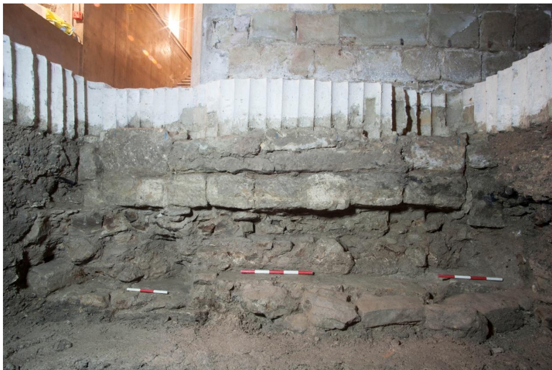
Plate 22 Elevation 2 (west facing) after removing the lower stones of 1067 (Image taken by Stuart Harrison)
