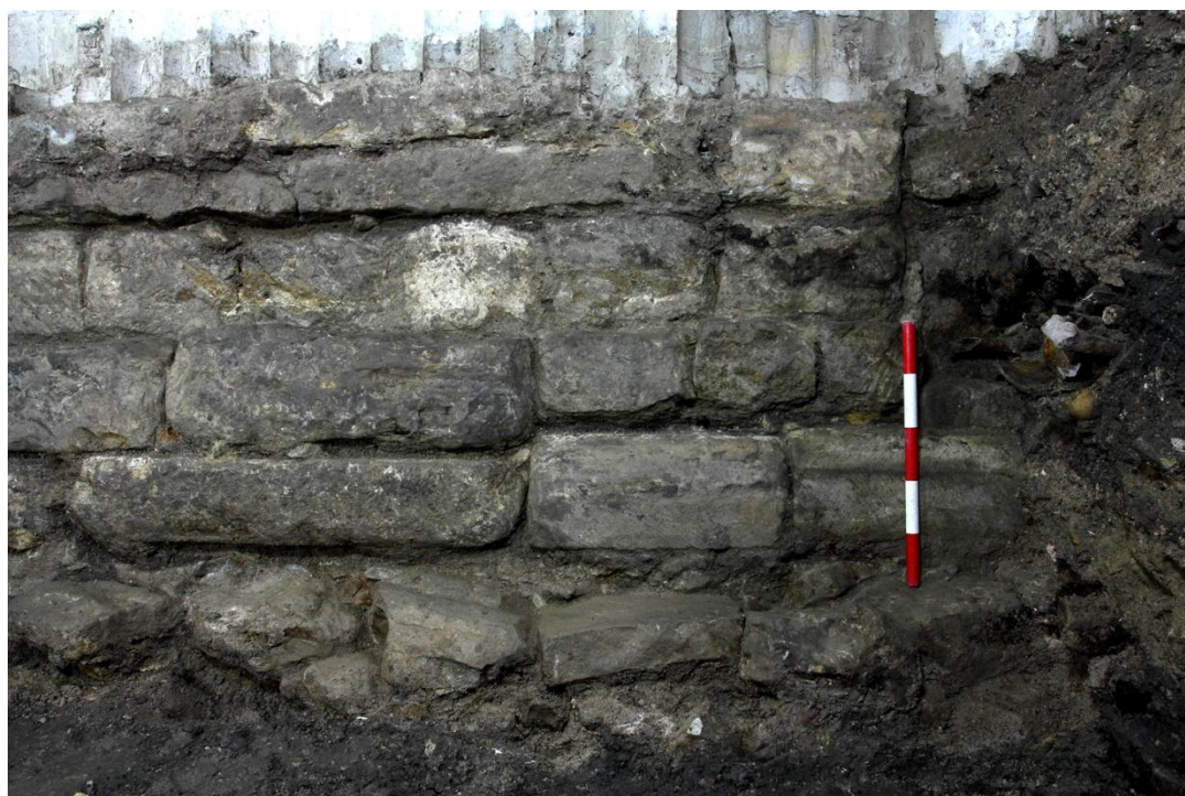
Plate 17 Southern end of elevation 2 (west facing) prior to removal of the projecting part of 1067, looking east
