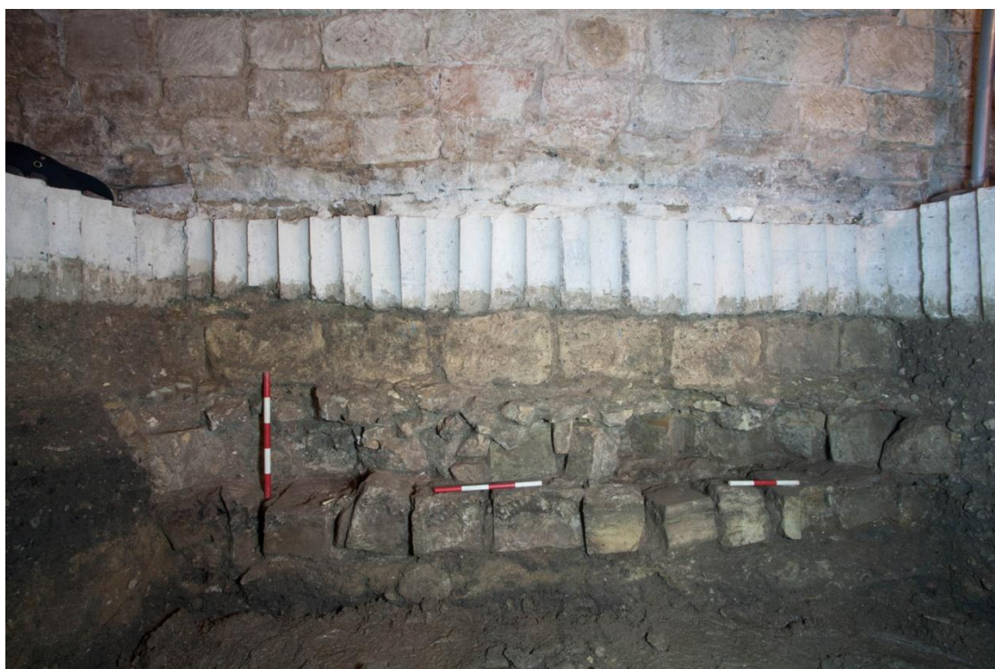
Plate 21 Elevation 4 (east facing) after removing the upper stones of 1043 (Image taken by Stuart Harrison)
