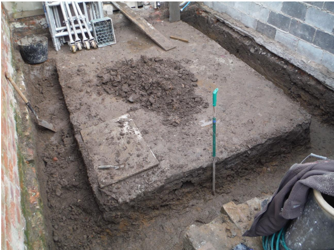
Plate 1 North East facing view showing U-shaped foundation trench.
