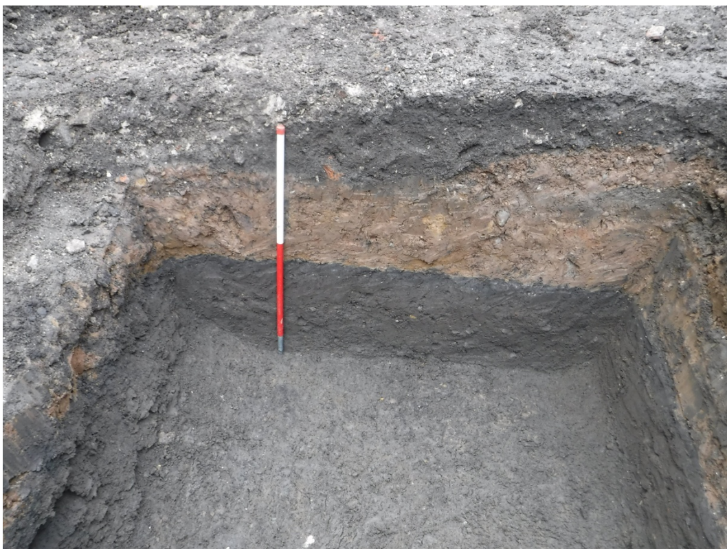
Plate 2 Section 2 showing made ground 1001, redeposited clay 1002 and horticultural soil 1003. Base of the trench is plough soil 1004. View west.
