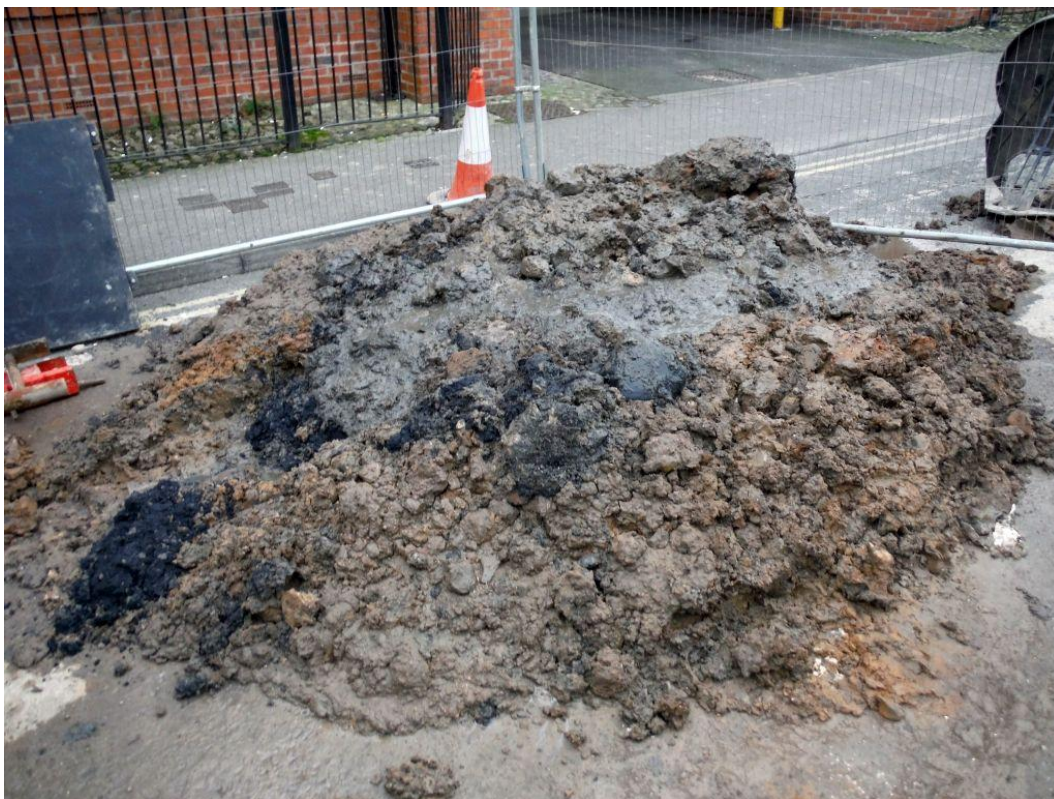
Plate 5 Typical deposits removed from contaminated part of works
