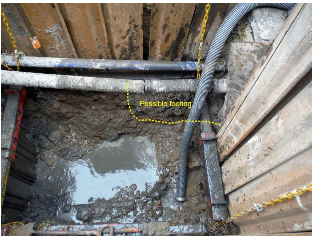
Plate 6 Possible footing (1008), facing northwest
