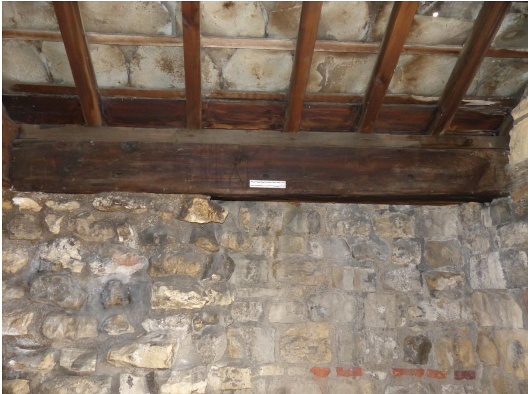
Plate 3 View of additional wall plate beam, looking west
