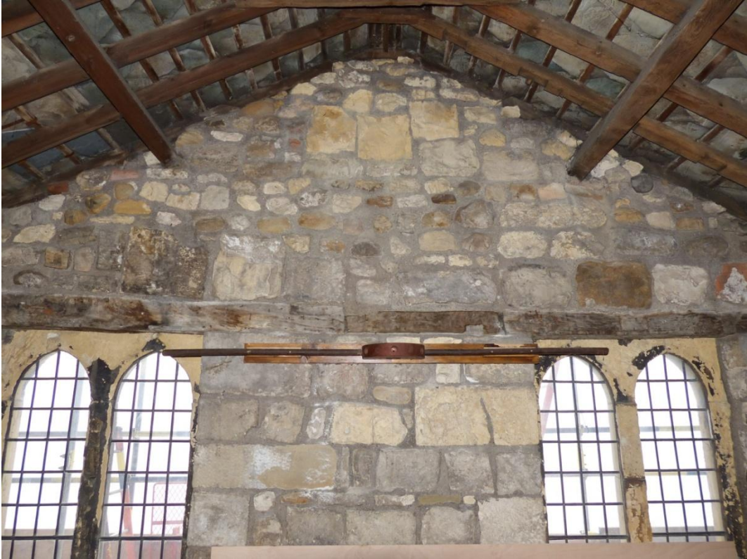
Plate 19 View of the north gable end incorporating reused timbers.
