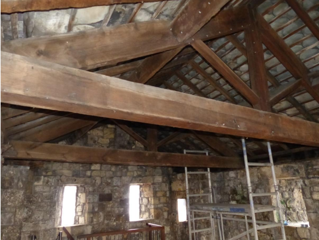
Plate 1 General view of the roof, looking northeast
