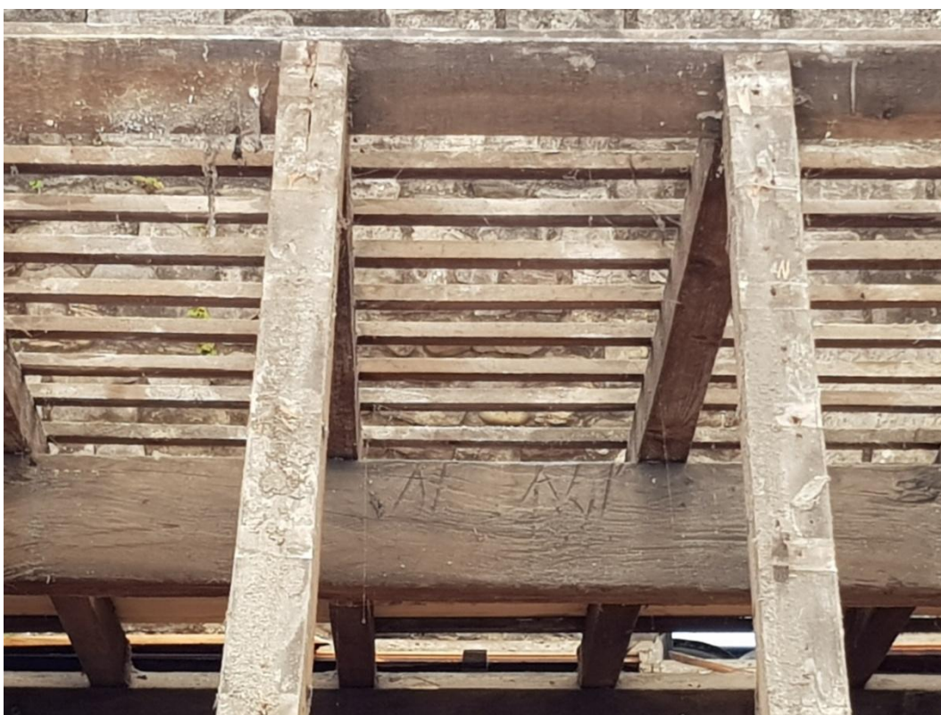
Plate 16 Detail view Baltic timber marks on the west purlin in the central bay
