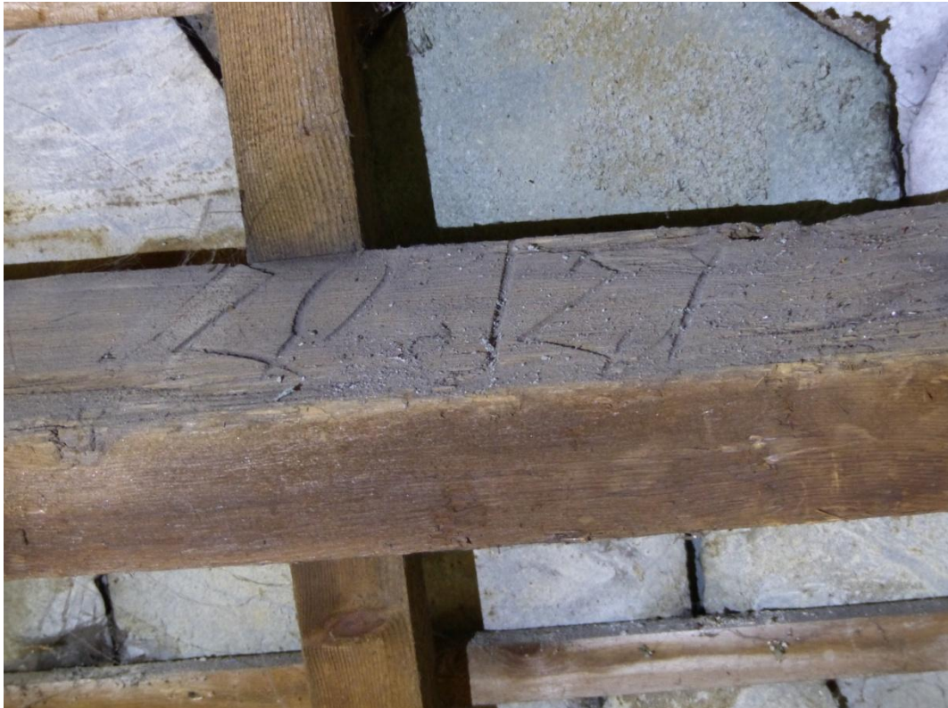
Plate 17 Detail view Baltic timber marks on the east purlin in the central bay
