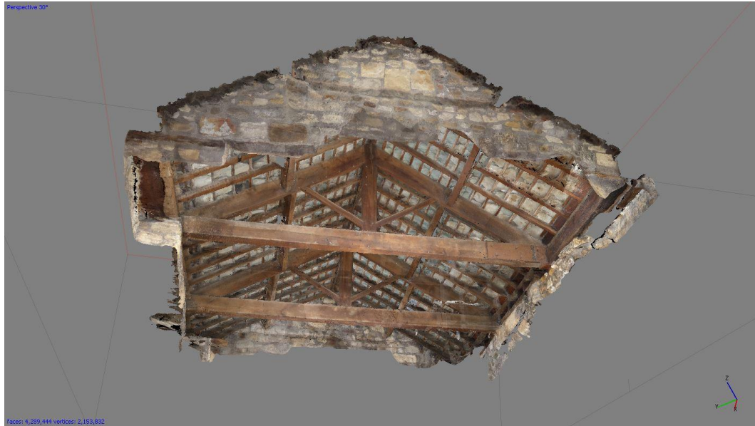
Figure 2: 3D model of internal roof space, looking north
