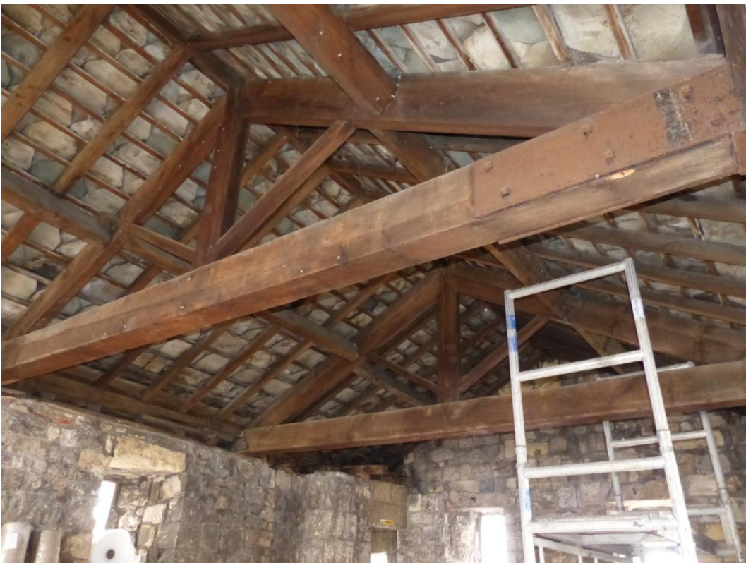
Plate 2 General view of the roof, looking northwest
