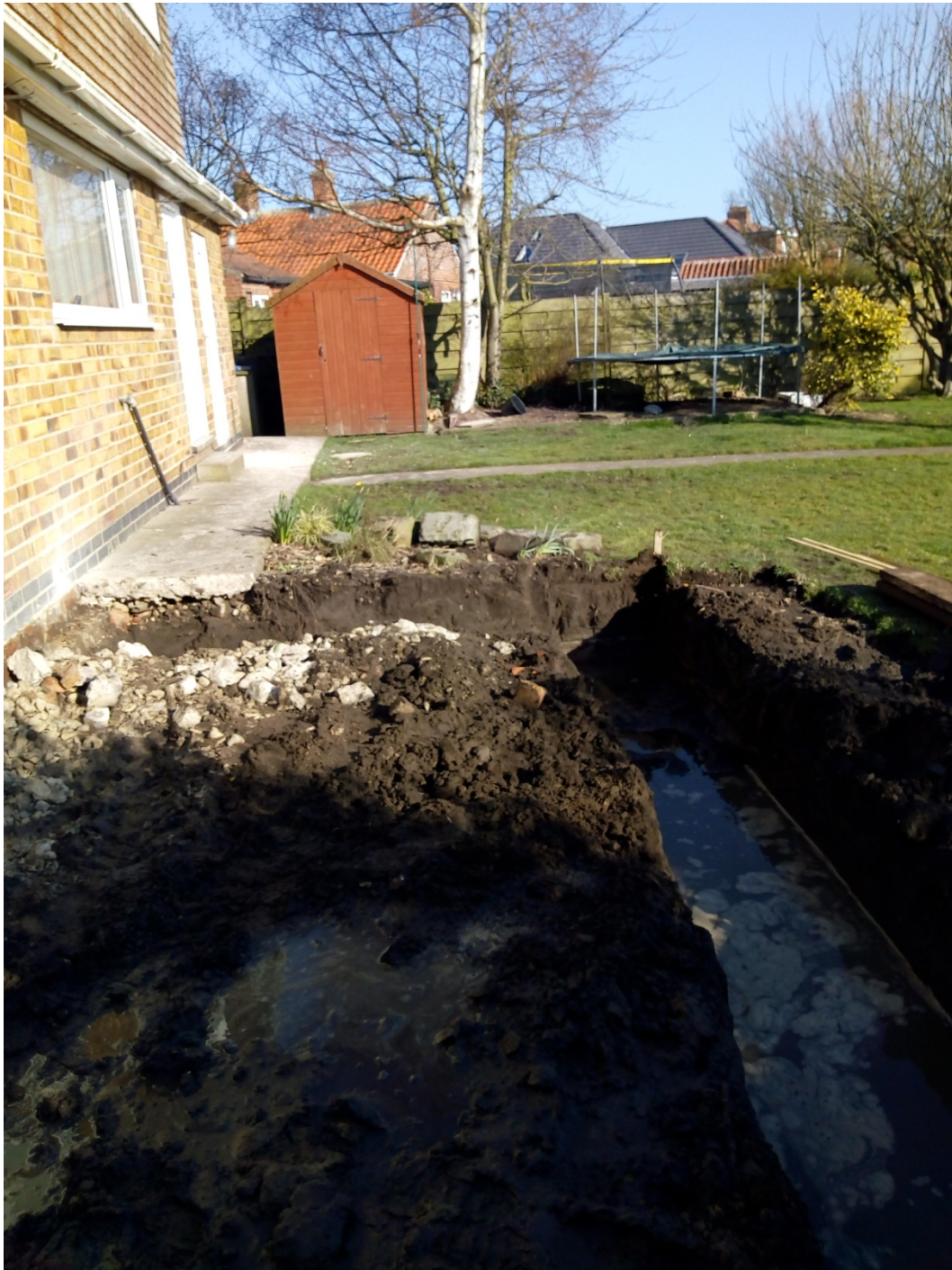
Plate 1 Foundation trench to rear of house, water table reached. View north.
