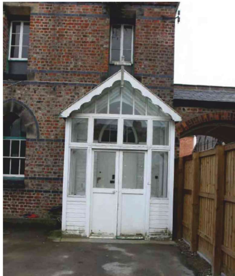
Plate 29 View of the timber and PVC porch entrance of the Extern, looking east. The porch appears on early 20th century maps but has been repaired and altered with plastic since.
