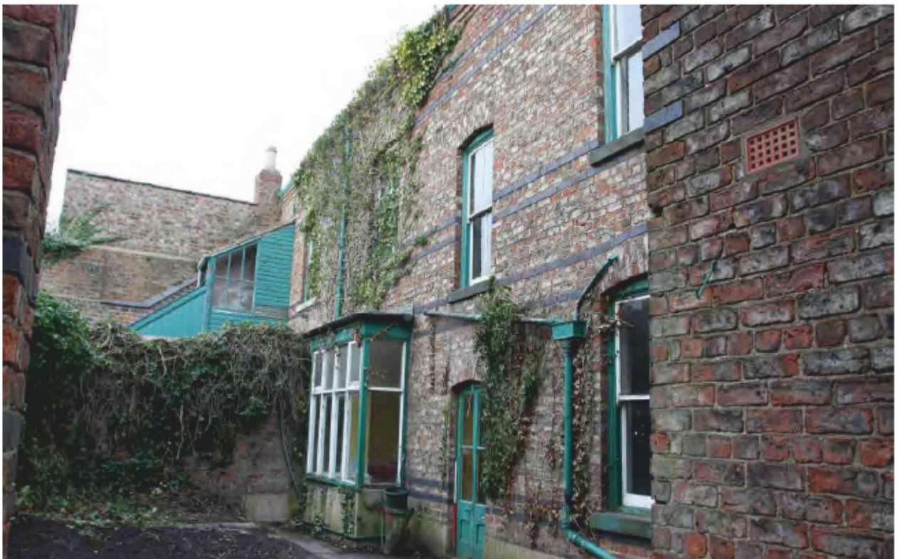
Plate 4 Alternate view of the southern elevation from within the walled garden area, looking northwest. Includes details of the 20 th century bay window addition.
