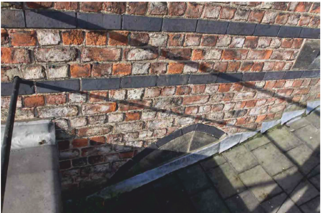
Plate 34 Detailed external view of the blocked up window, looking northwest.
