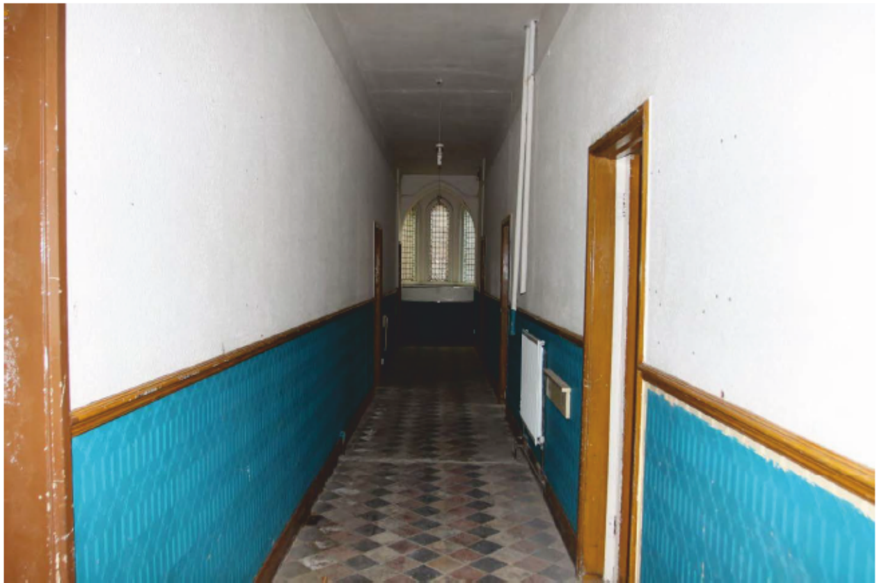
Plate 37 Central passageway on the ground floor of the Extern, looking north.
