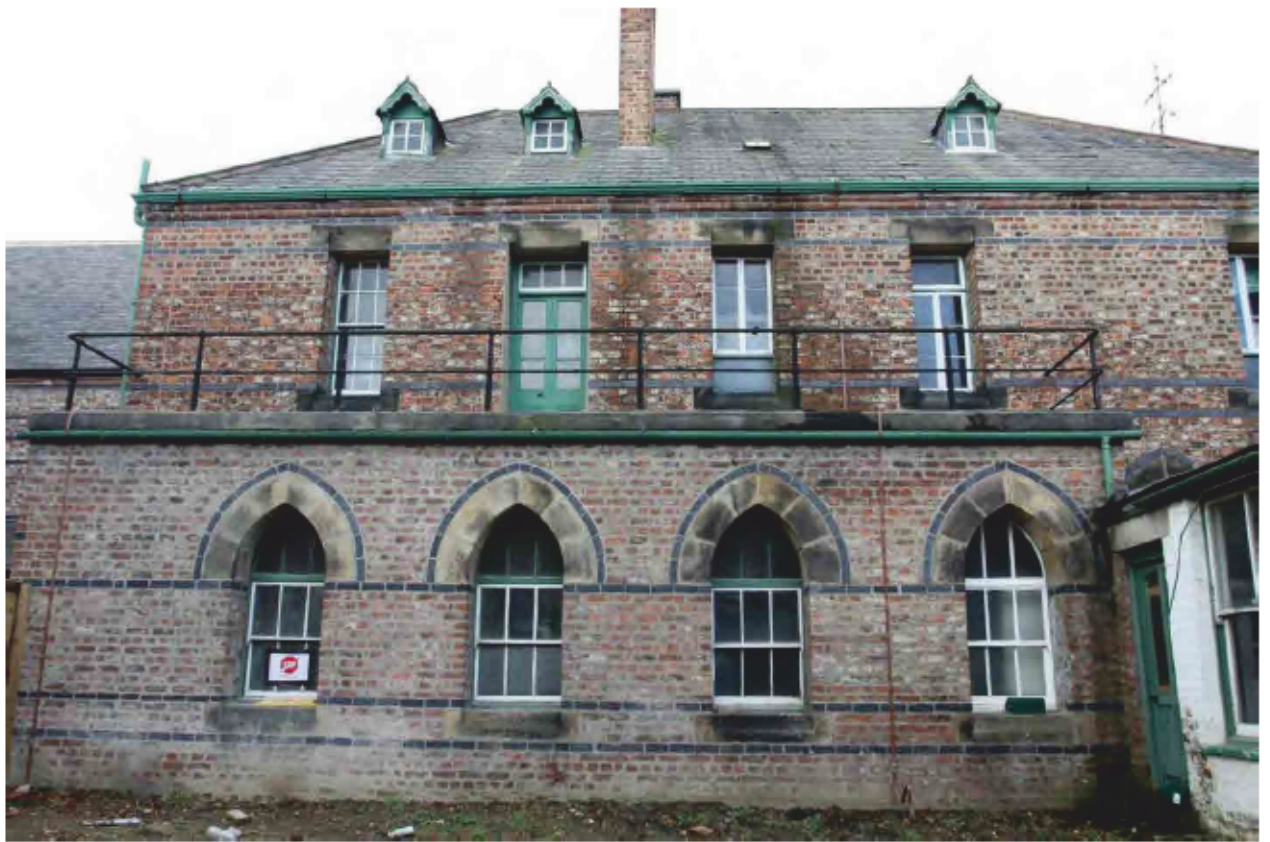
Plate 27 View of the eastern elevation of the Extern, looking west.
