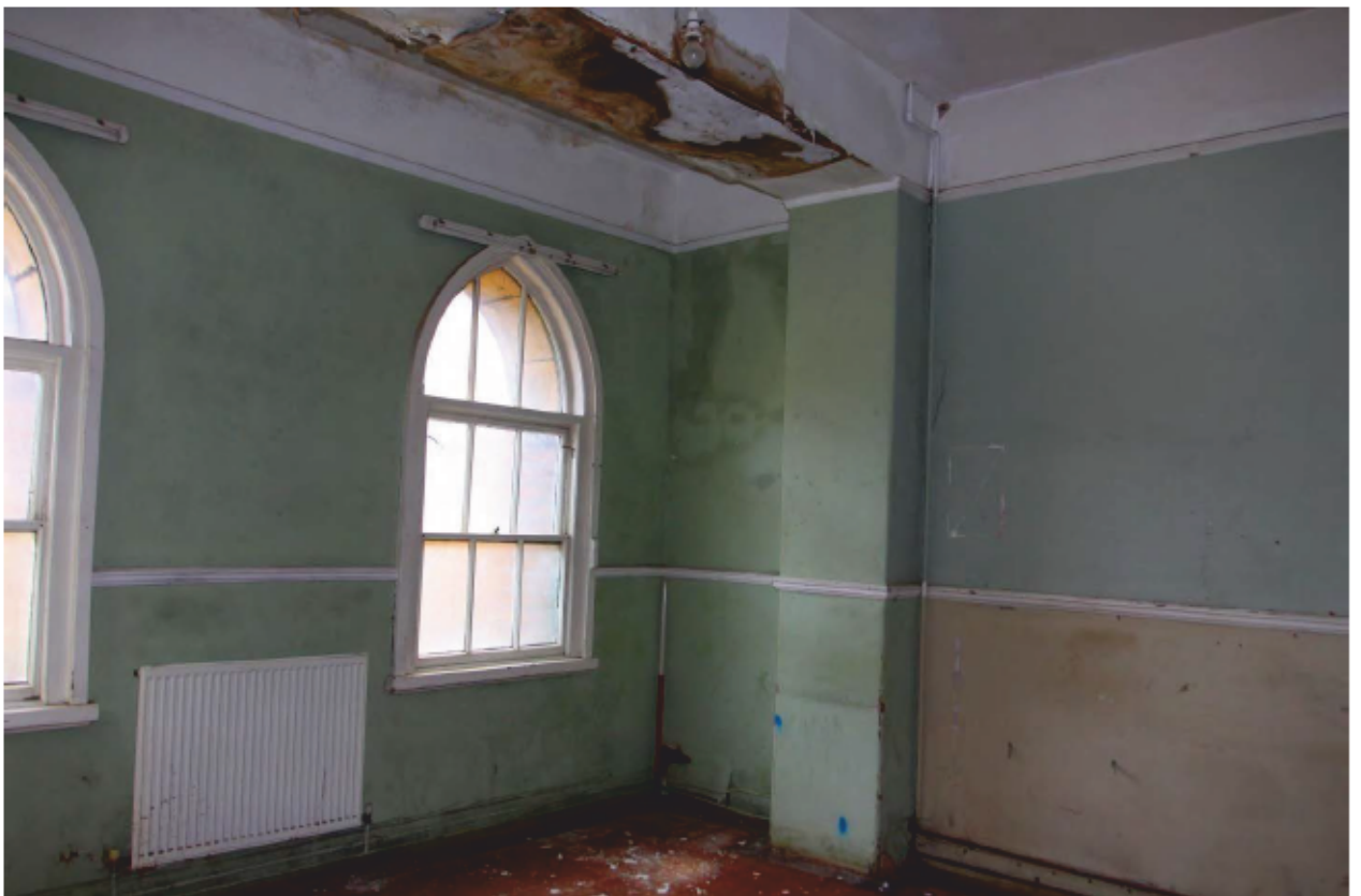
Plate 40 Ground floor parlour room with balcony extension visible, looking southeast.
