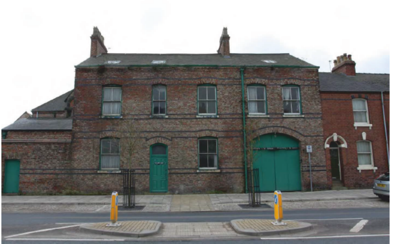
Plate 1 View of the north facing elevation of the Lodge from Lawrence Street, looking south.
