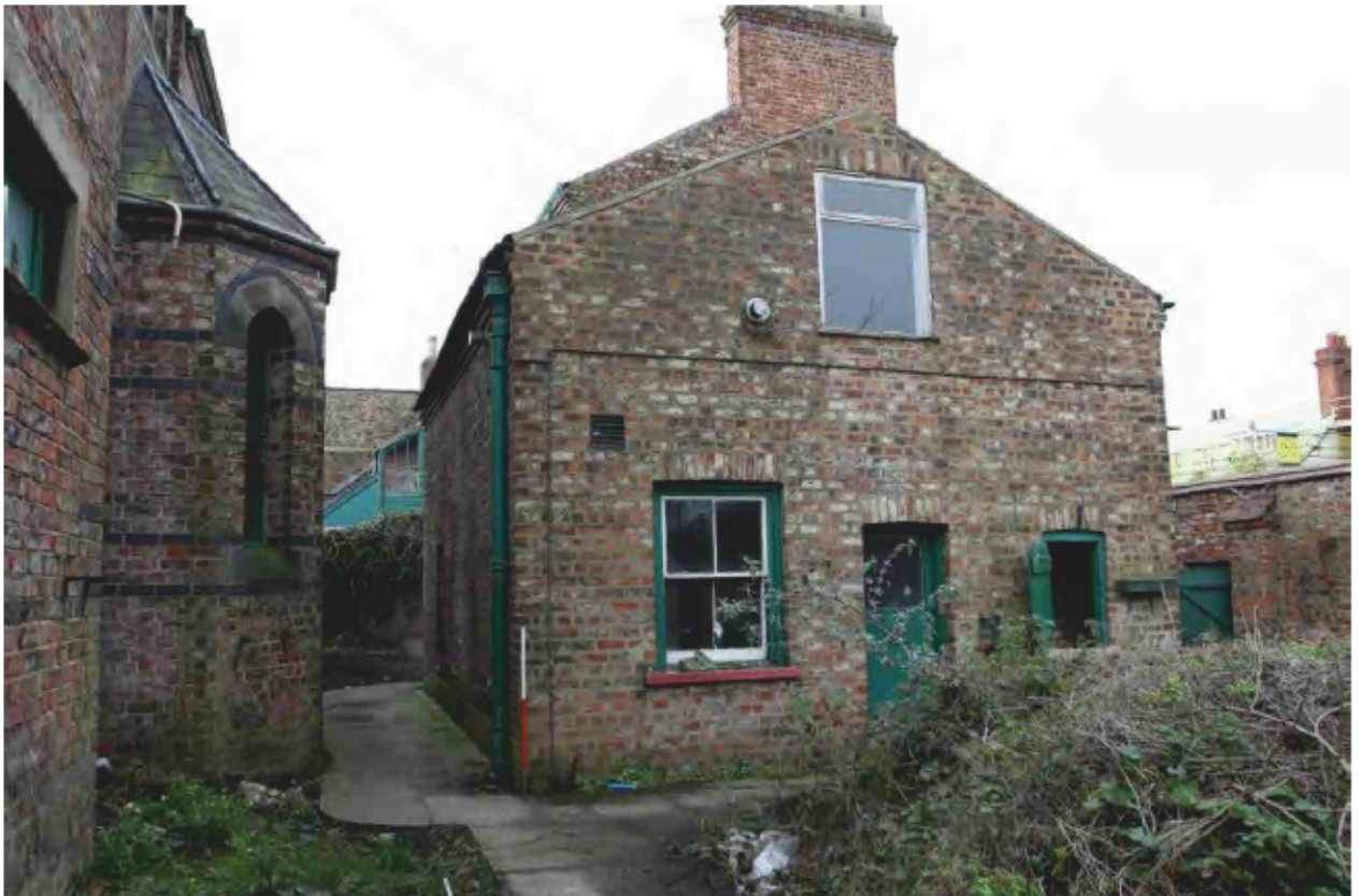
Plate 6 View of the eastern elevation of the Lodge's extension, looking northwest.
