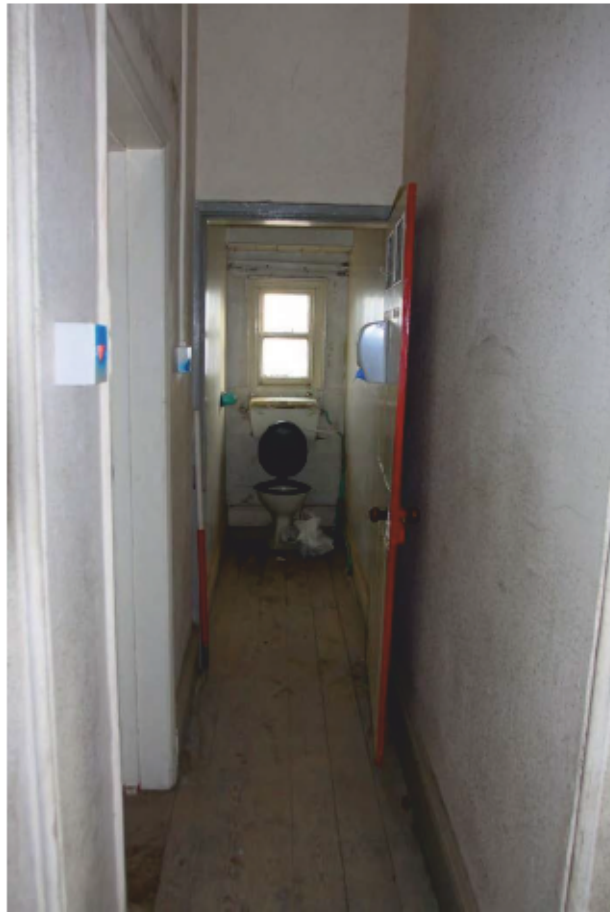
Plate 19 Narrow toilet on the first floor of the Lodge, looking east. Most of the toilet rooms within the two buildings are narrow.
