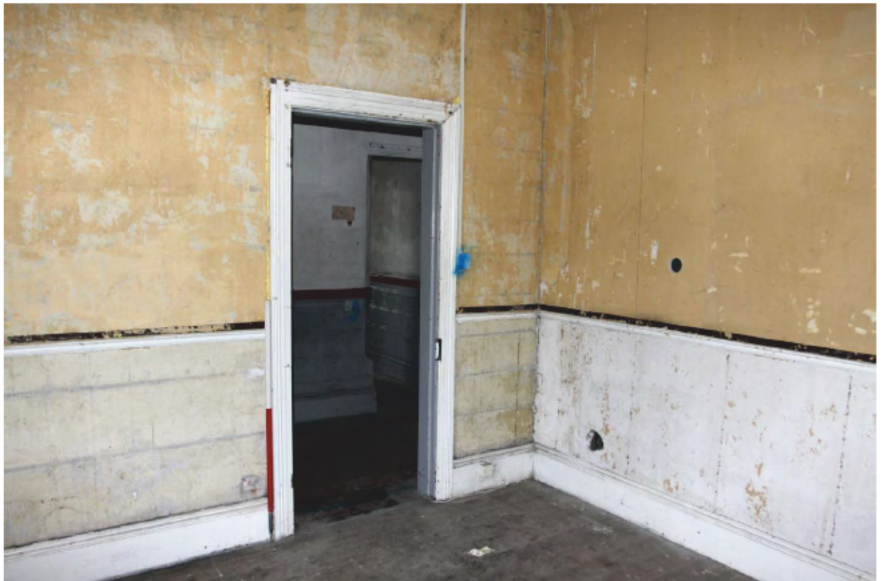
Plate 11 Detail of the entrance, door architrave and dado rail in the front parlour of the Lodge, looking southeast.
