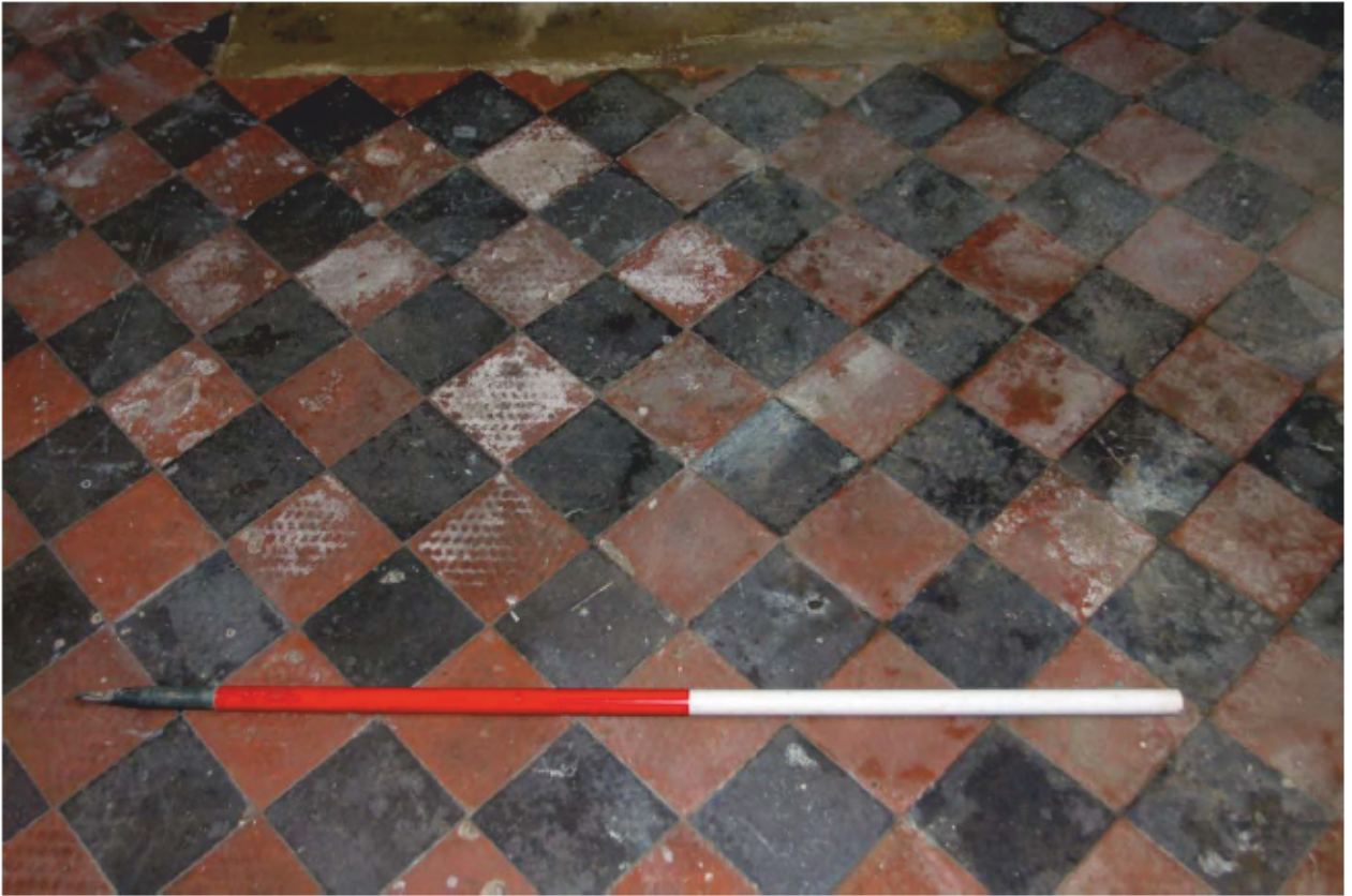
Plate 15 Detail of the original 19th century ceramic tiled floor of the Lodge.
