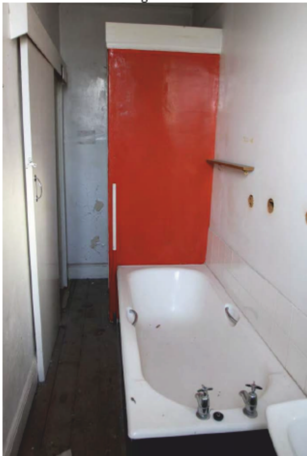
Plate 20 Bathroom on the first floor of the Lodge, looking west.
