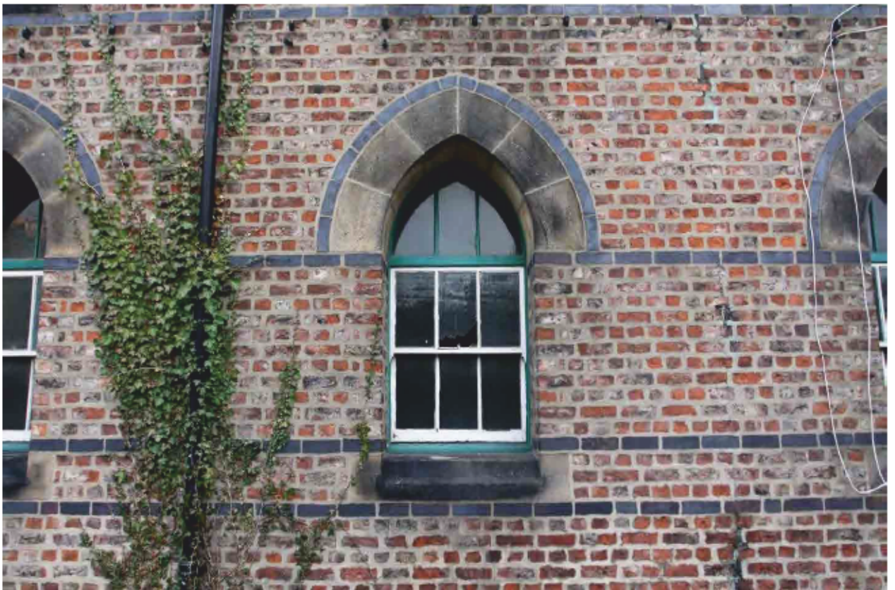
Plate 32 Ground floor window of the Extern detailing the blue brick string courses, stone sills, overlights and arched heads of ashlar voussoirs, looking east.
