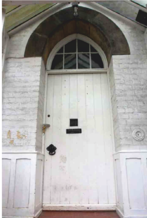
Plate 29 View of the timber and PVC porch entrance of the Extern, looking east. The porch appears on early 20th century maps but has been repaired and altered with plastic since.
