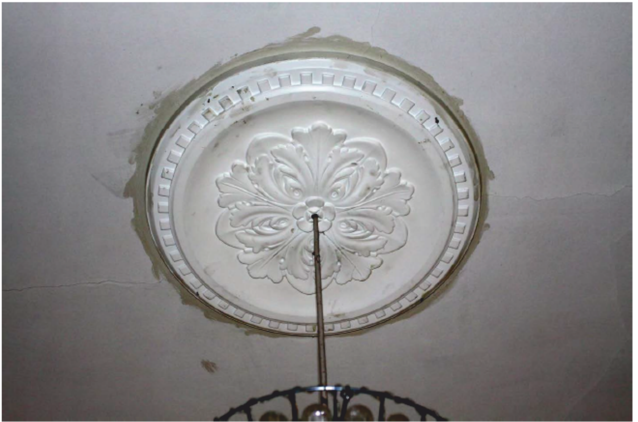
Plate 13 Detail of an original plaster moulded ceiling rose in the rear parlour of the Lodge
