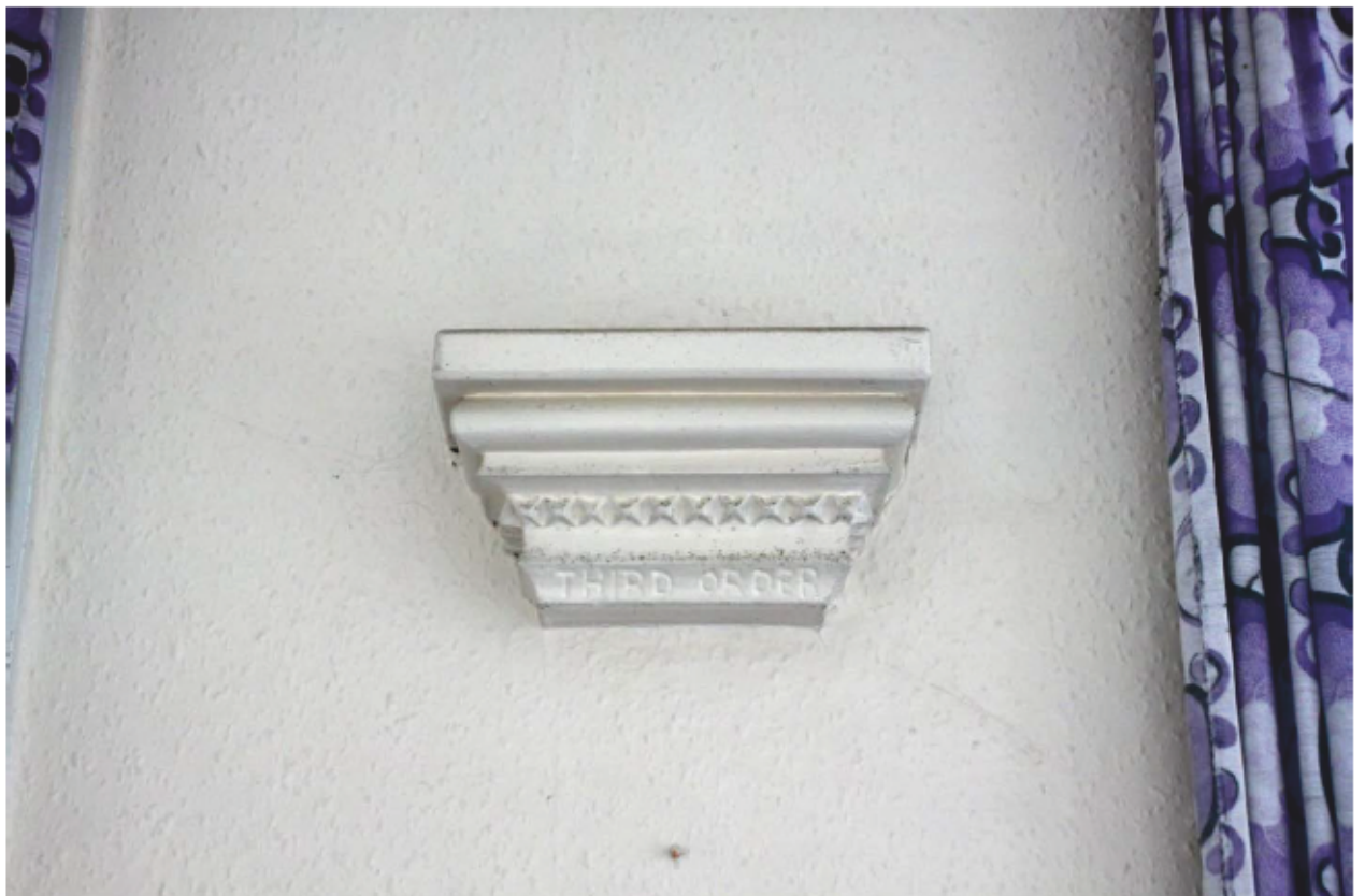
Plate 22 Detail of a moulded plaster corbel within a bedroom of the first floor of the Lodge.
