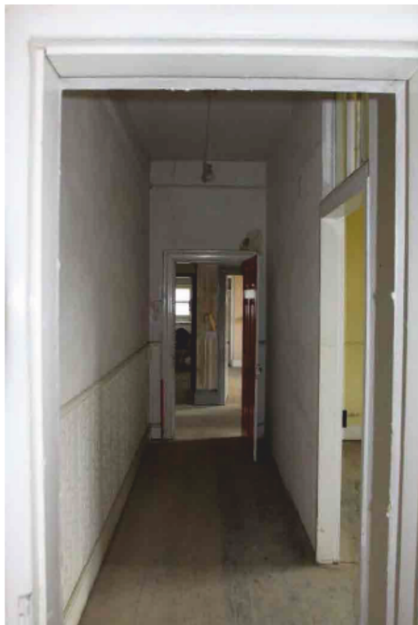
Plate 16 Central passageway on the first floor of the Lodge, looking west.
