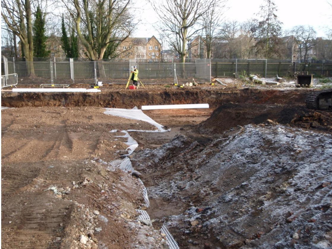
Plate 3. North-east facing view of site strip and laying of piling mat.
