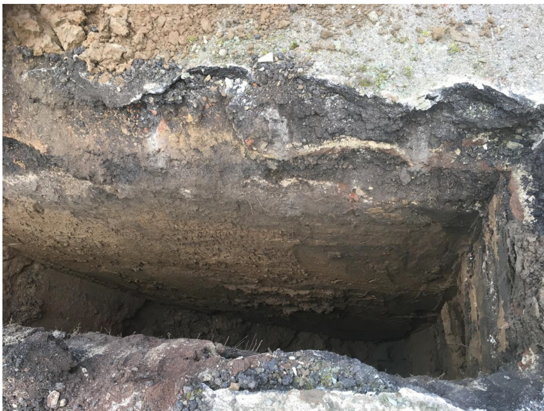
Plate 2. North facing view of Trial Pit 6.
