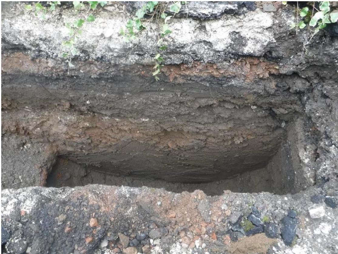
Plate 1. North-west facing view of Trial Pit 1.
