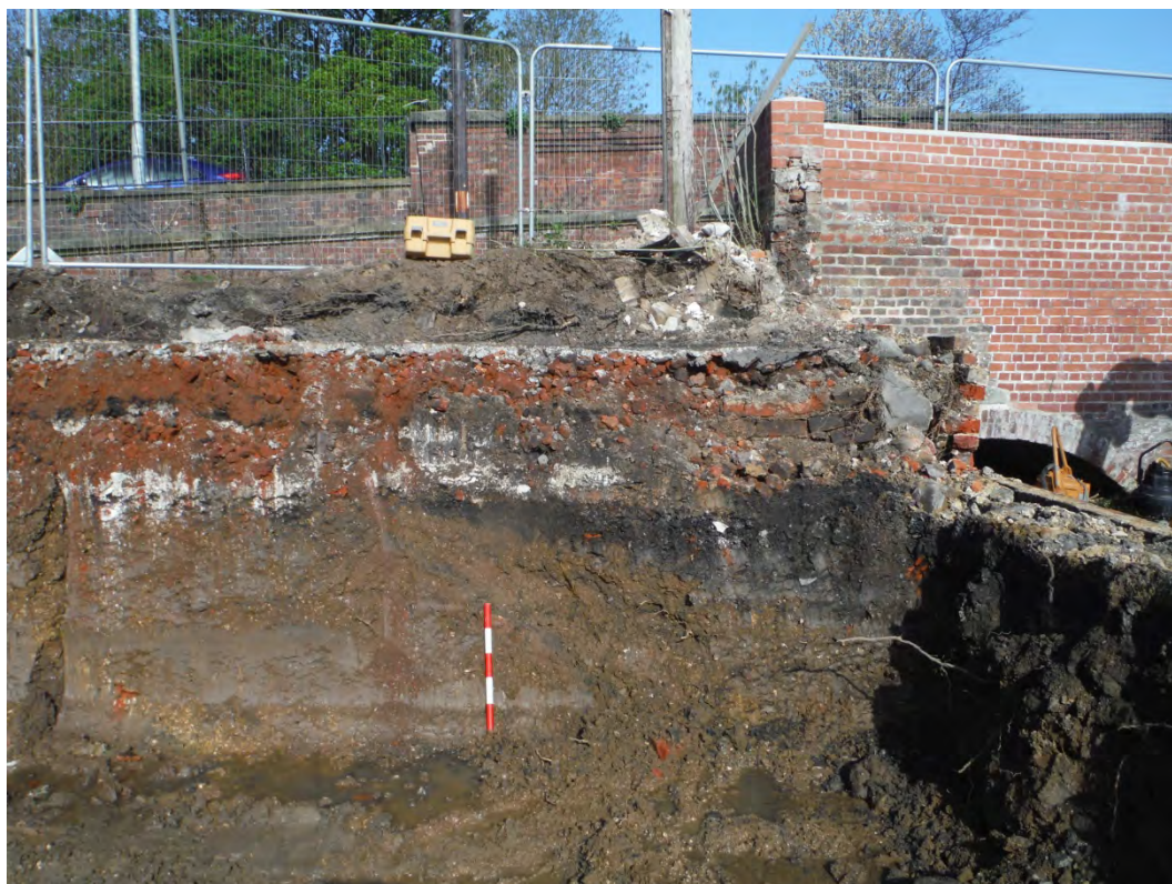
Plate 3 Construction cut 1008 of revetment wall (facing north west 0.5m scale)
