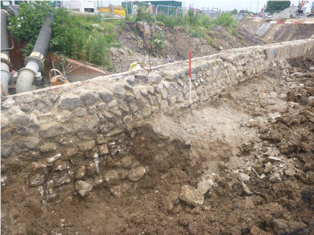
Plate 11 revetment wall 1005 and concrete wall 1015 (facing north east 1.0m scale)
