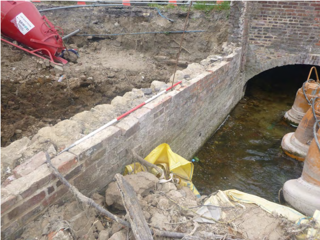
Plate 9 Northern face of Retaining wall 1014 (facing south west 1.0m scale)
