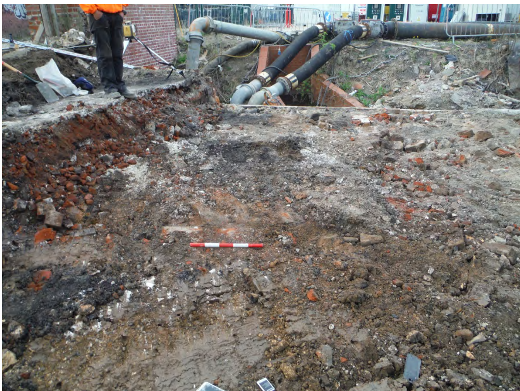
Plate 2 Context 1001 (facing north 0.5m scale)
