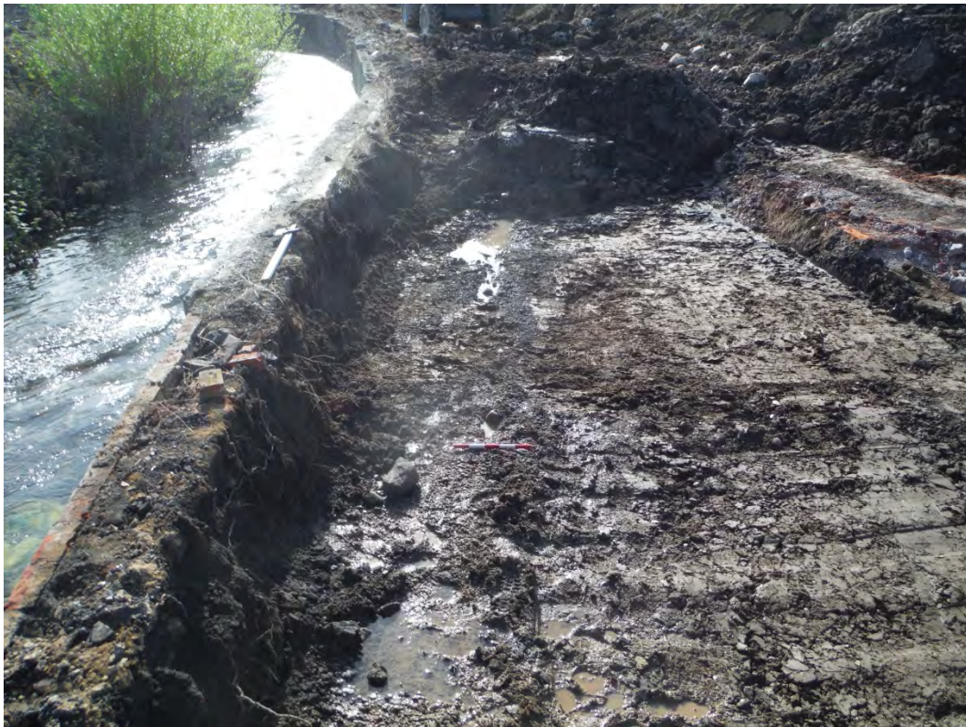
Plate 1 Construction cut 1008 and natural 1010 (facing east 0.5m scale)
