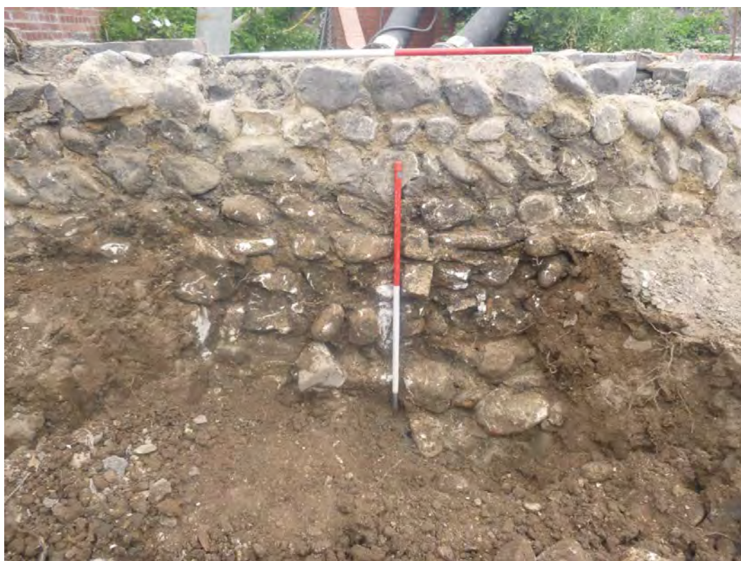
Plate 8 Retaining wall 1005 (facing north 1.0m scale).
