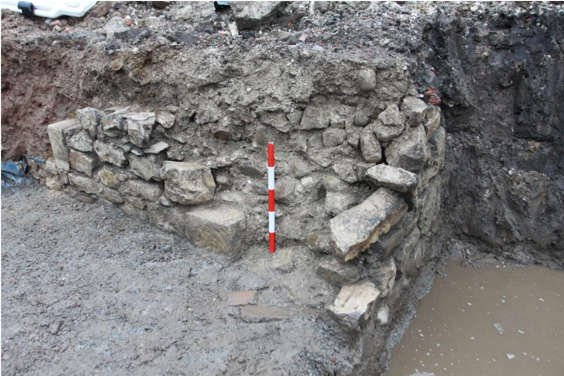
Plate 1 Medieval wall; part of the 13 th –14 th century extension, Building 2.
