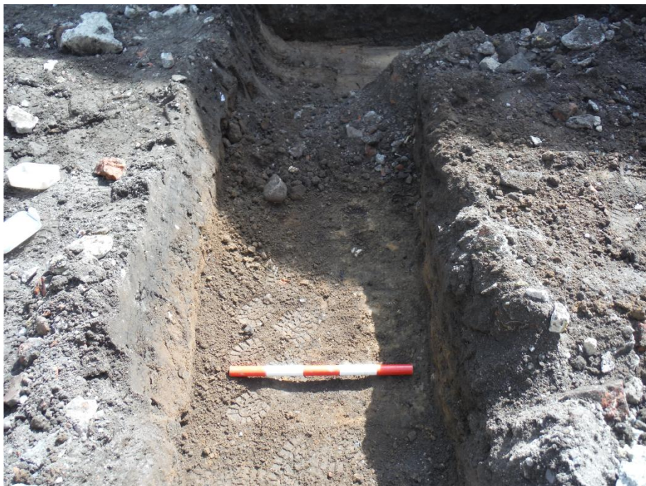
Plate 4 Strip foundation at southern end of site, looking east
