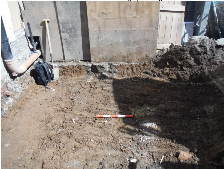
Plate 2 Area strip at northern end of site, looking east
