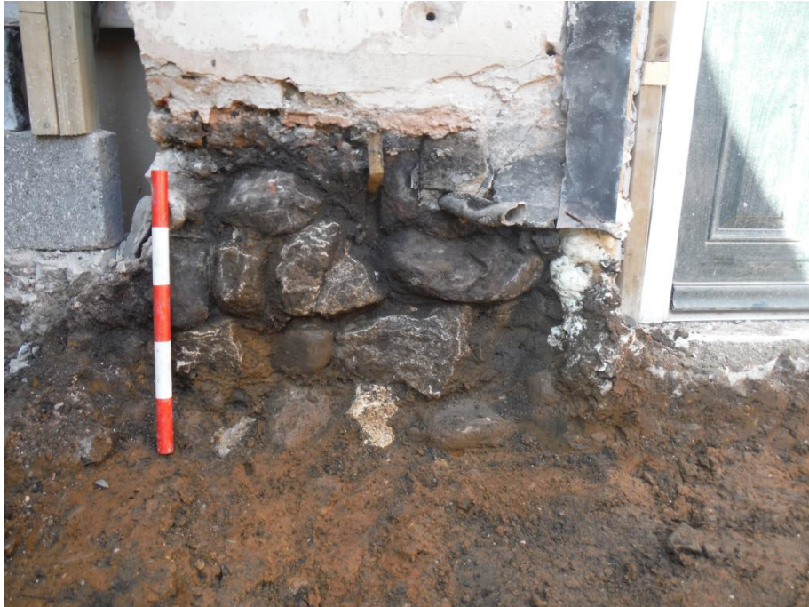
Plate 5 Foundation of standing building, section 1, looking north
