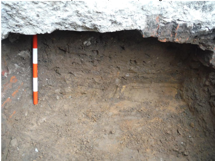
Plate 8 Underpinning pit, section 4, looking east
