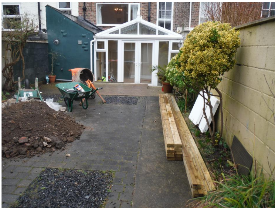
Plate 1 Before works begin, looking north
