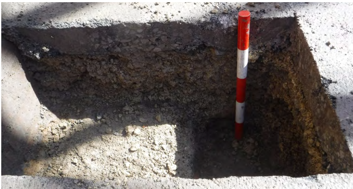
Plate 15 TP01, view northeast, scale 0.5m
