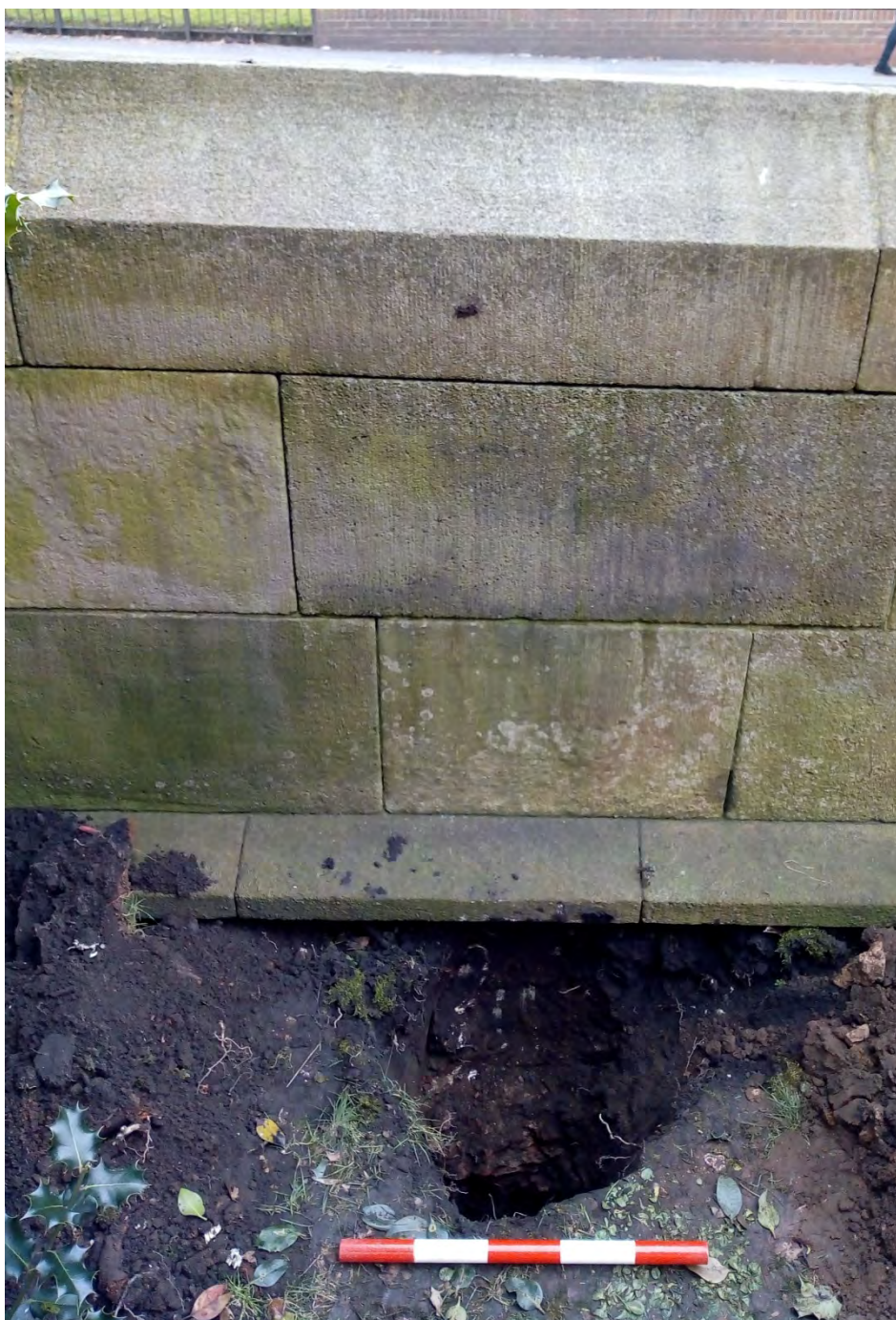
Plate 17 TP10, view west, scale 0.5m
