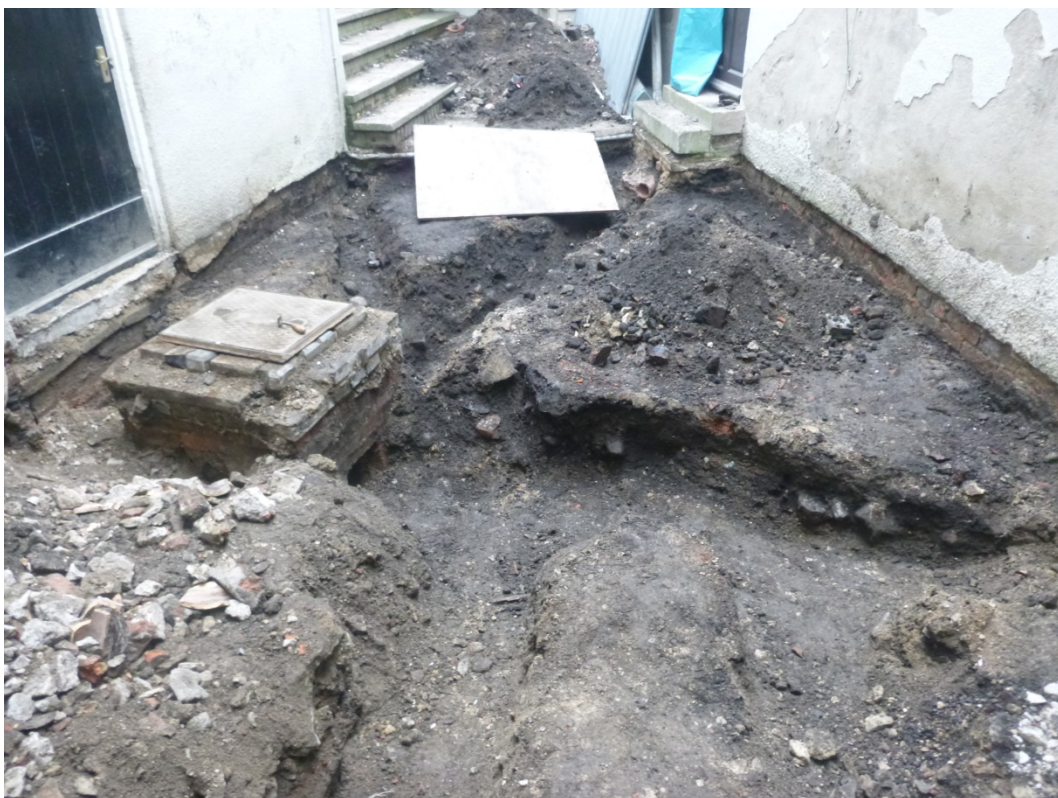
Plate 4 Lower yard after the removal of ceramic drains, facing north-west
