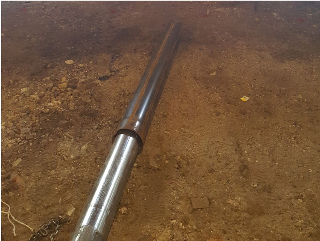
Plate 9 Shot of displacement pile prior to ground penetration
