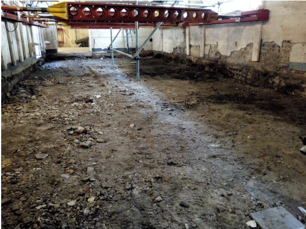
Plate 7 Main basement after ground reduction, facing east
