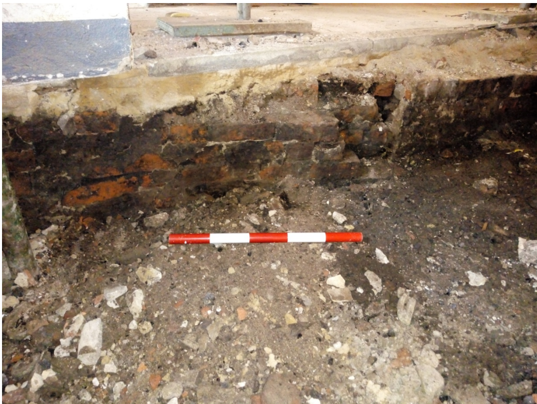
Plate 8 Shot of curved wall featured in 1852 OS map at south-west end of main basement, facing south-west, scale unit 100mm
