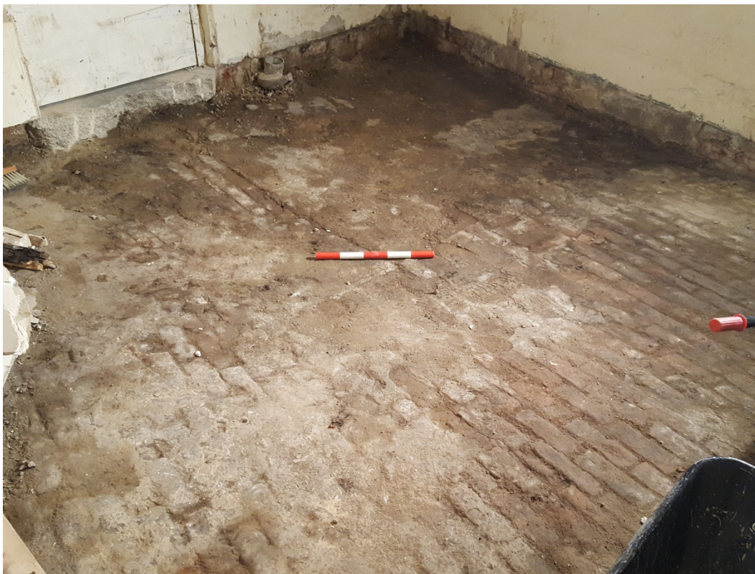
Plate 6 Rear basement revealing in-situ brick floor, facing east, scale unit 100mm
