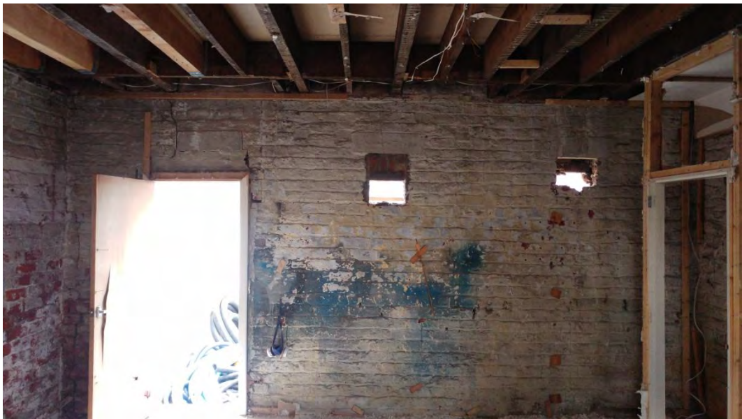
Plate 21 Ventilation openings in west wall of west coach house, looking west
