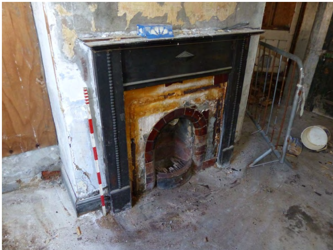
Plate 39 Fireplace in parlour of cottage, looking north-east
