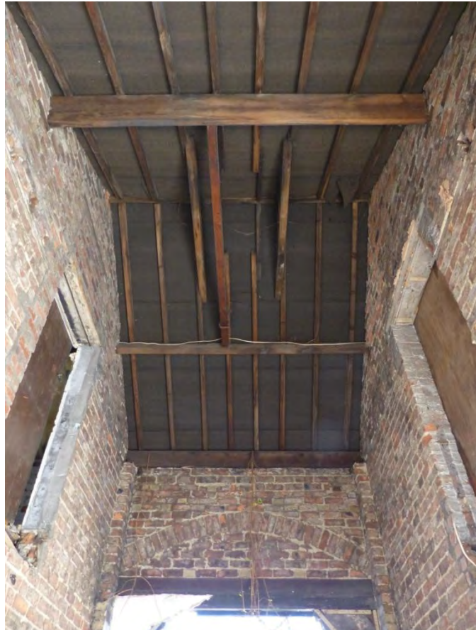
Plate 18 Interior of carriageway roof, looking west
