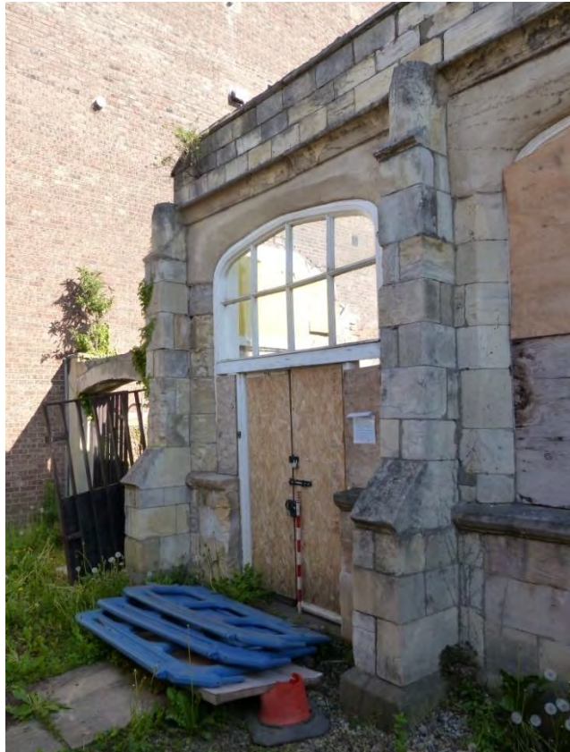
Plate 8 Detail of north arch, looking north-east
