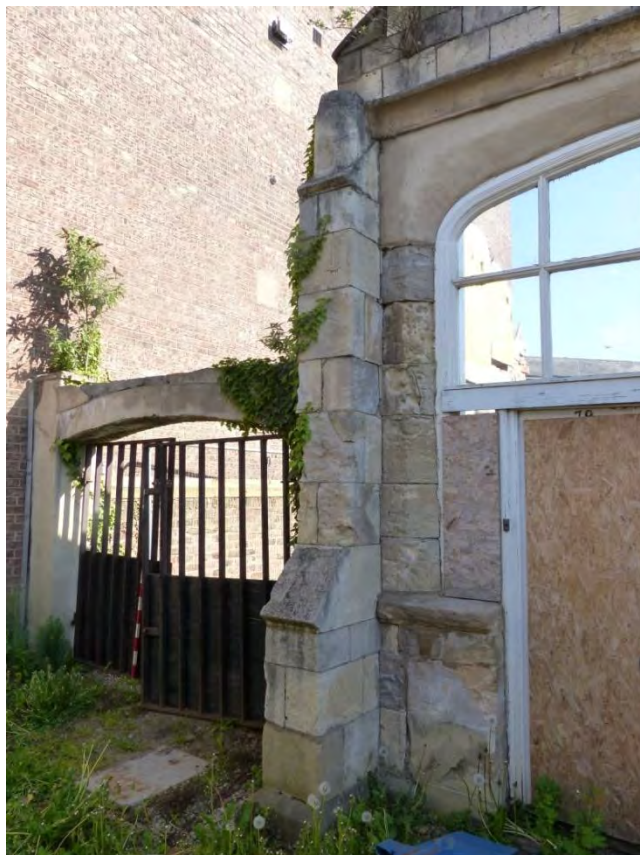
Plate 9 Detail of buttress and later arch opening, looking north-east
