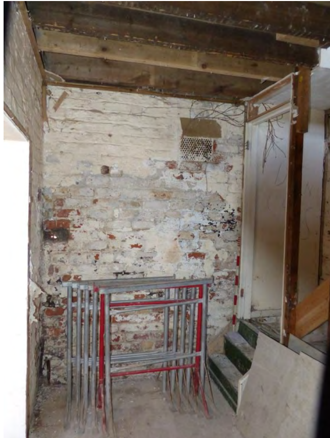
Plate 26 Ground floor of north room in west coach house, looking north
