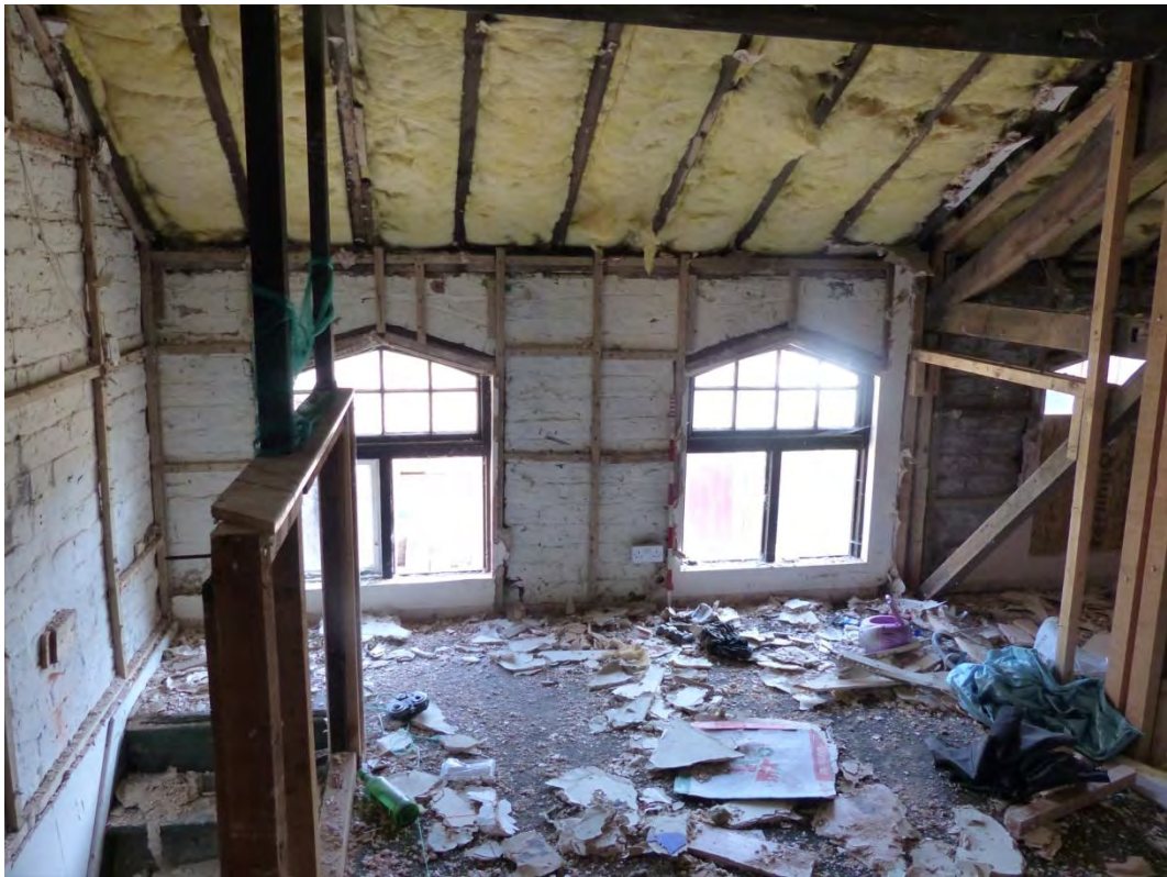
Plate 23 First floor east wall of west coach house, looking east
