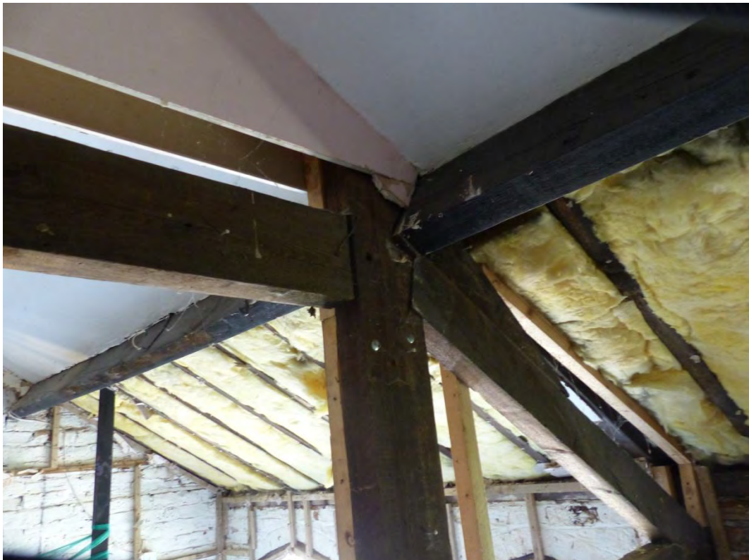
Plate 25 Detail of roof truss in west coach house, looking south-west
