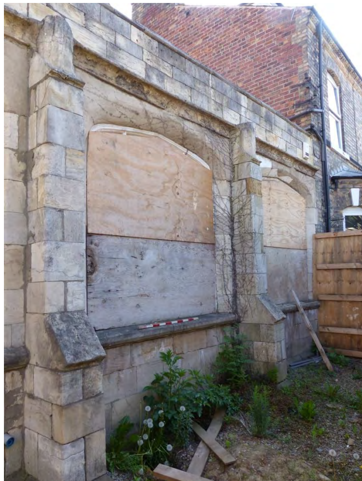
Plate 7 Detail of the arches, looking south-east
