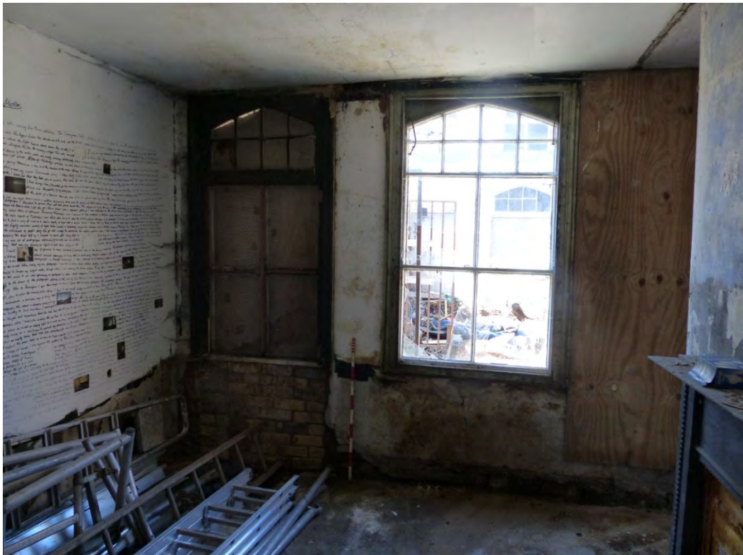
Plate 37 West wall in parlour of cottage, looking west
