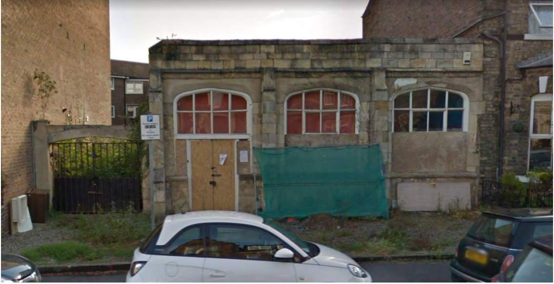
Plate 6 General view of the York Theatre Royal arcade, looking east (2017)
