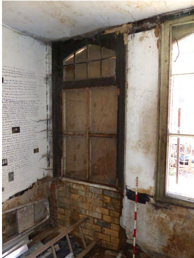
Plate 38 Former door opening in parlour of cottage, looking south-east
