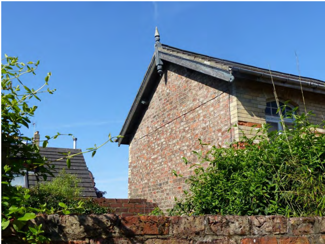
Plate 17 General view of the roof, looking north-west
