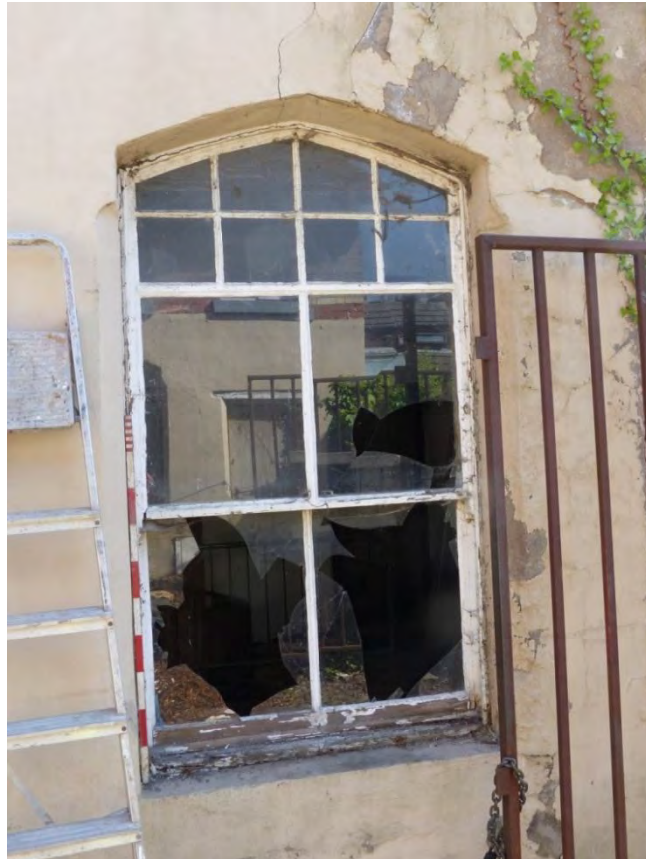
Plate 28 Detail of window to west elevation of cottage, looking east
