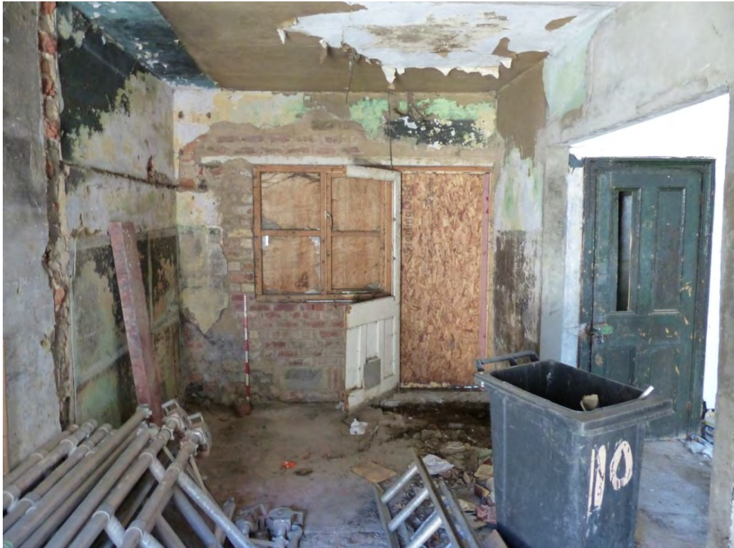
Plate 34 Ground floor north room of cottage, looking east
