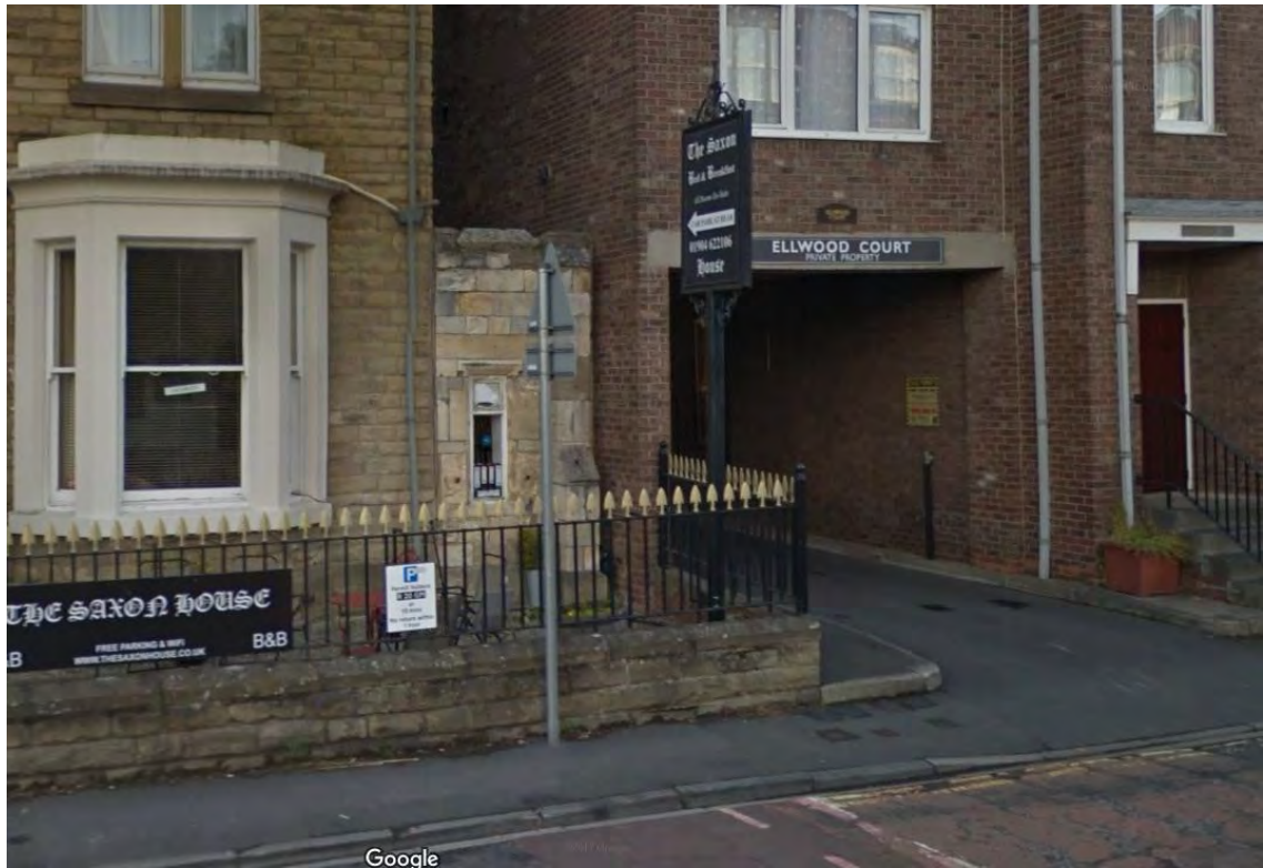
Plate 5 Street image of the remaining portion of the arcade between Ellwood Court and the Manor House B&B
