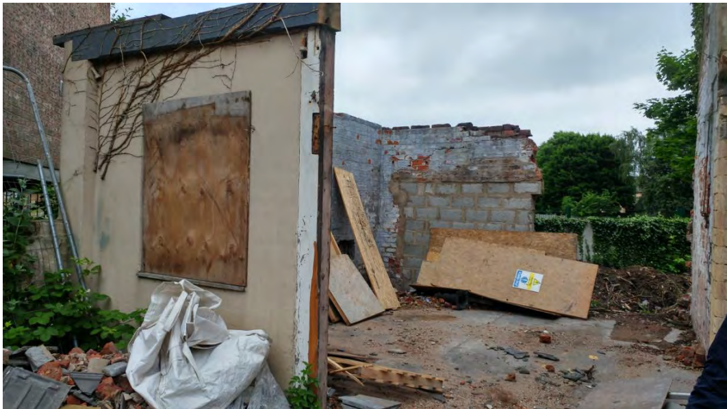
Plate 33 Partially demolished remains of carriage house, looking east
