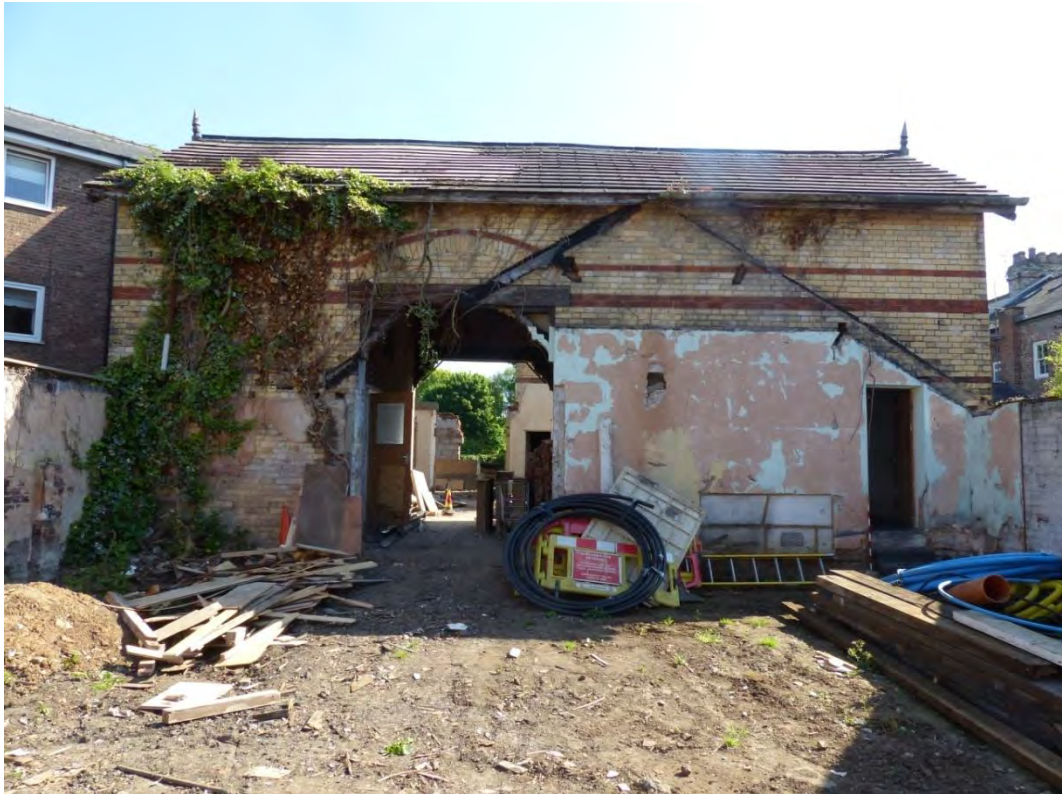
Plate 12 West elevation of the west coach house, looking east
