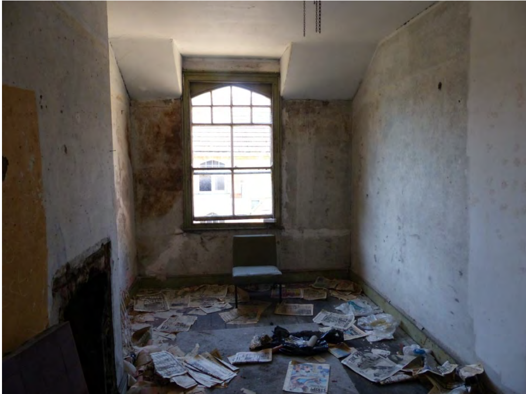
Plate 45 First floor north bedroom in the cottage, looking west
