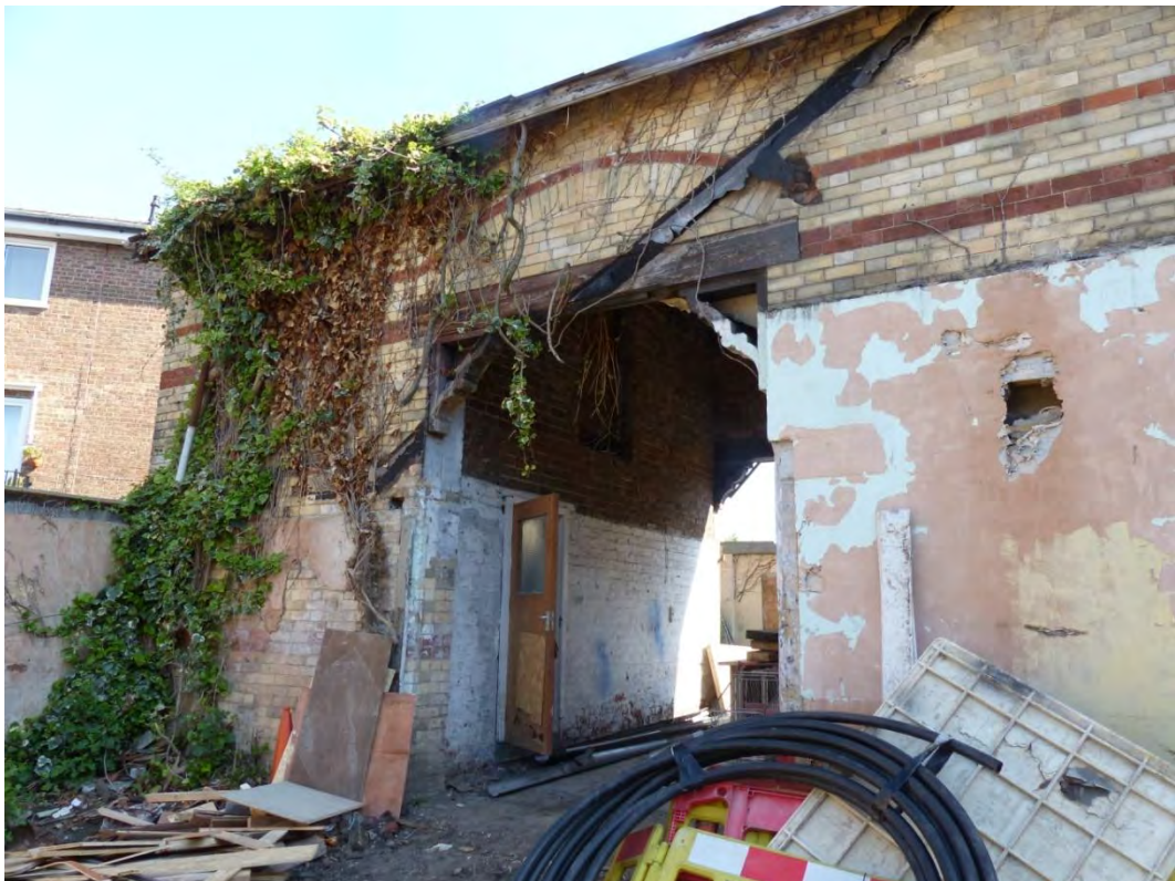
Plate 13 Detail of carriageway from west elevation, looking north-east
