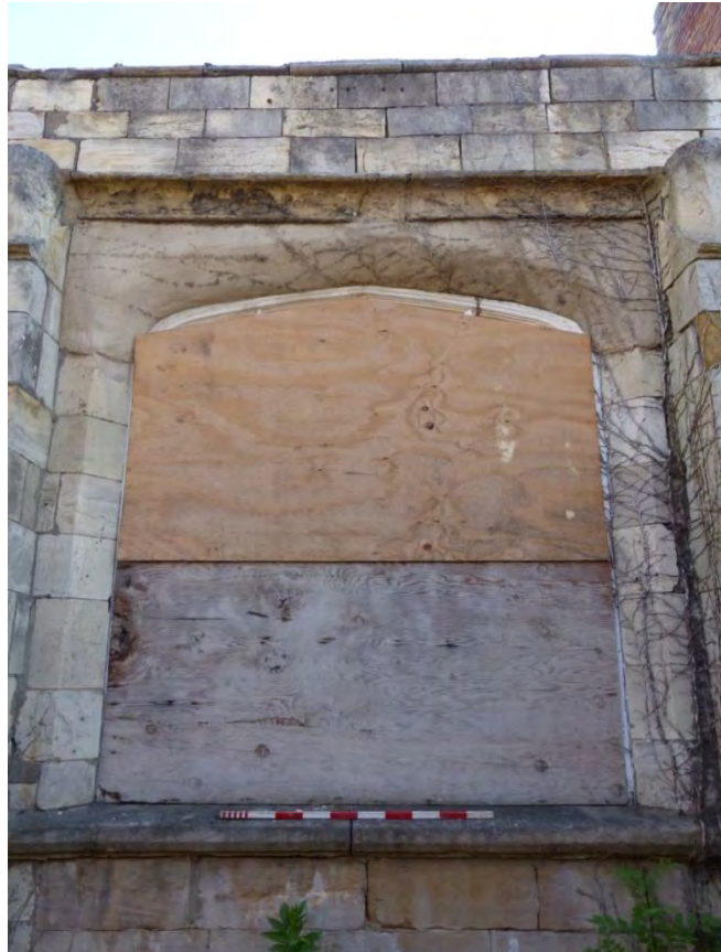
Plate 10 Detail of arch opening, looking east
