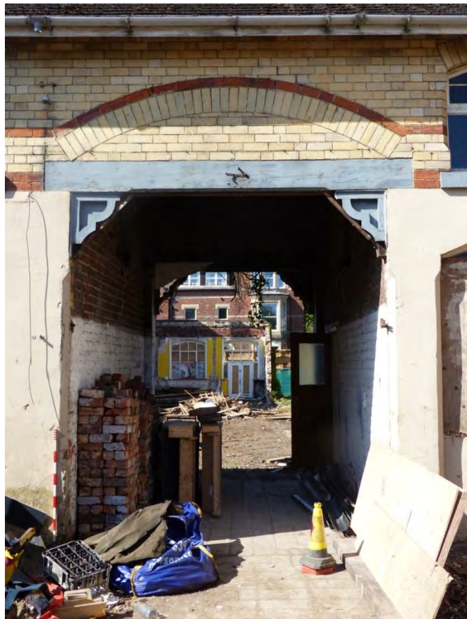
Plate 15 Carriageway through west coach house, looking west
