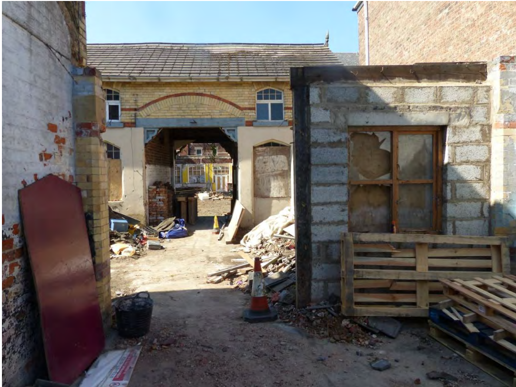
Plate 32 Partially demolished interior of carriage house, looking east
