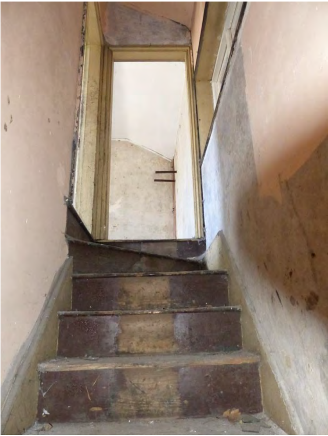
Plate 41 Detail up the stairs in the cottage, looking north
