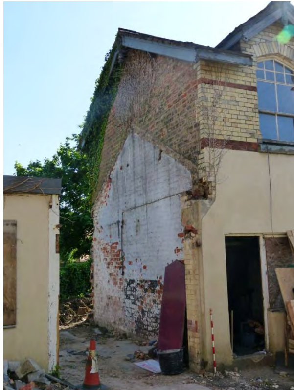
Plate 31 Side (north) elevation of coachman's cottage, looking south-east
