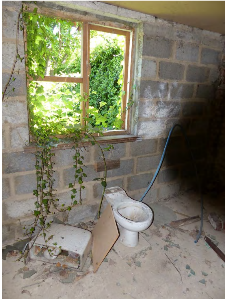
Plate 46 The interior of the lean-to addition of the cottage, looking south-east
