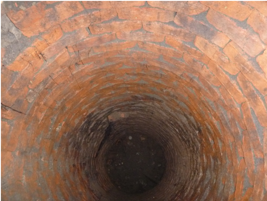
Plate 10 Well interior, note soil at base of well c.3.5m below well capping.
