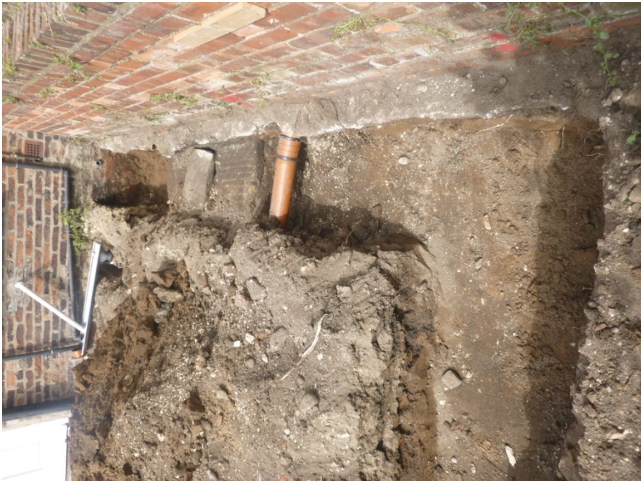
Plate 8 Foundation trench at north end of site, looking west.
