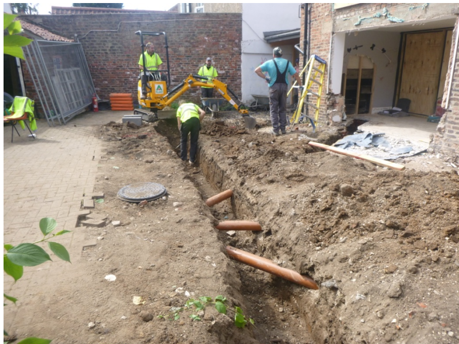
Plate 2 foundation trench excavation in progress.
