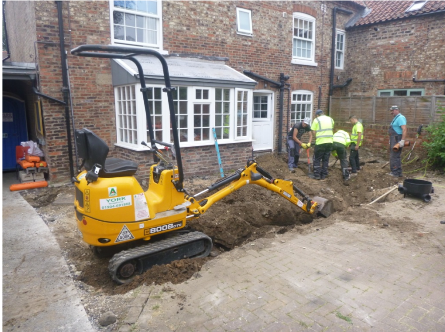
Plate 1 Drainage excavation in progress.
