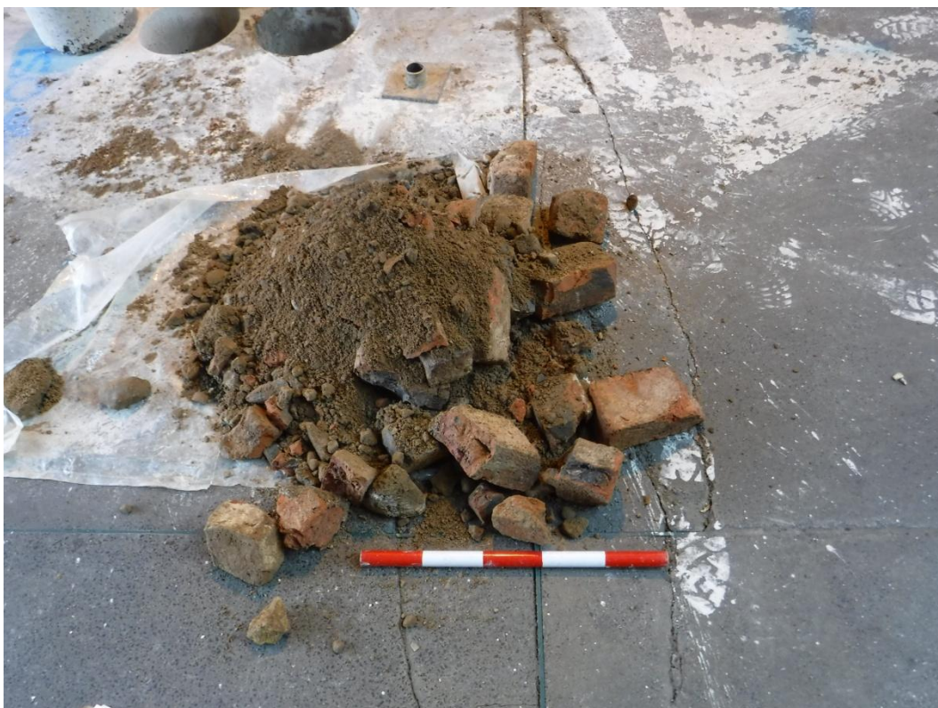
Plate 10 WS202, loose rubble from immediately below the car park floor to 1.2m BPGL, possibly deriving from the demolition of earlier structure on the car park site, 0.1m scale units.
