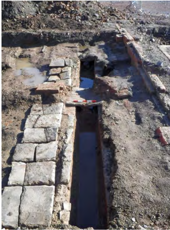
Plate 9 Culvert (c3011) in the yard area of Trench 3
