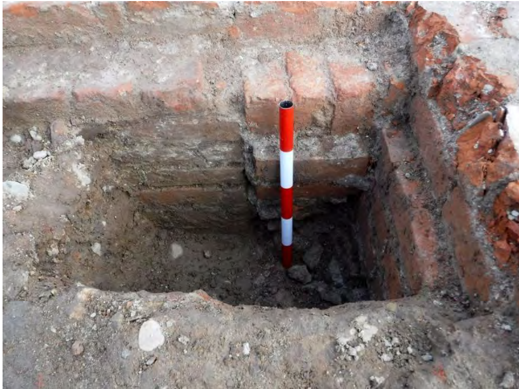
Plate 3 Section where the Early Quadrangle Wall (c1013), on the left, joins the prison wing wall (c1015), on the right, characterised by a change in brick thickness and mortar. Trench 1.
