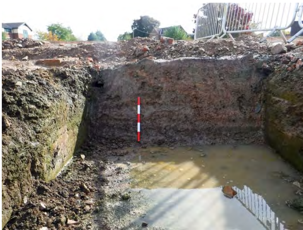
Plate 11 Section in Trench 4 sondage showing the layers of pre-prison landscaping (c4005) and the buried soil (c4006)
