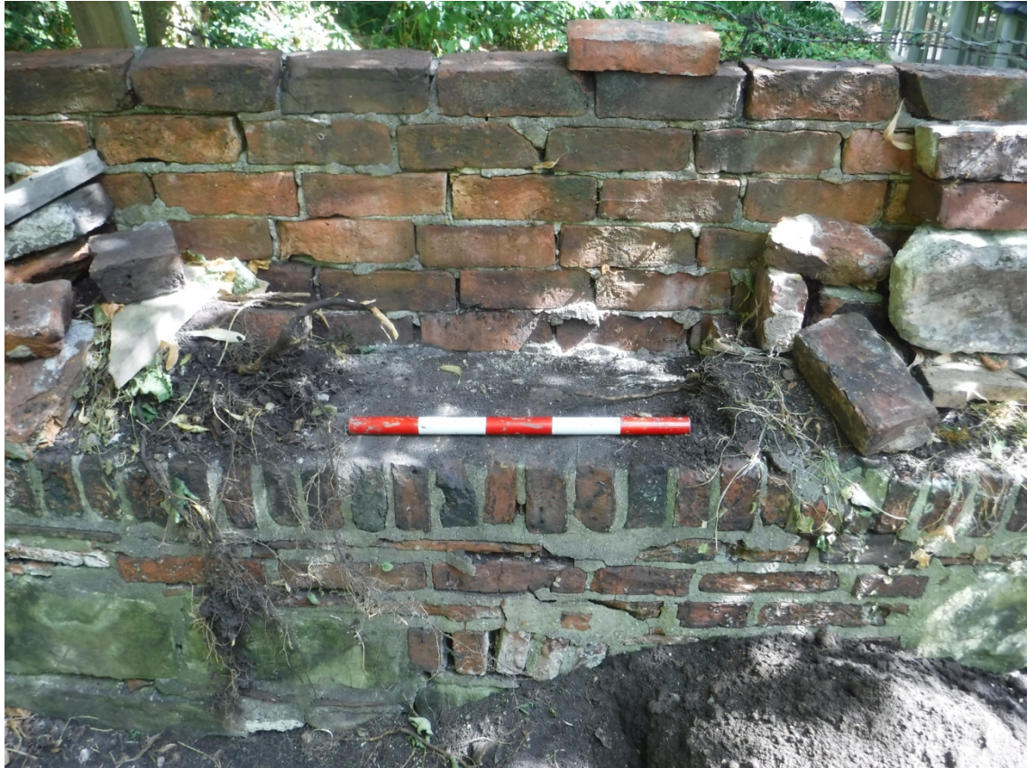
Plate 2 view northeast of later additions to the wall.
