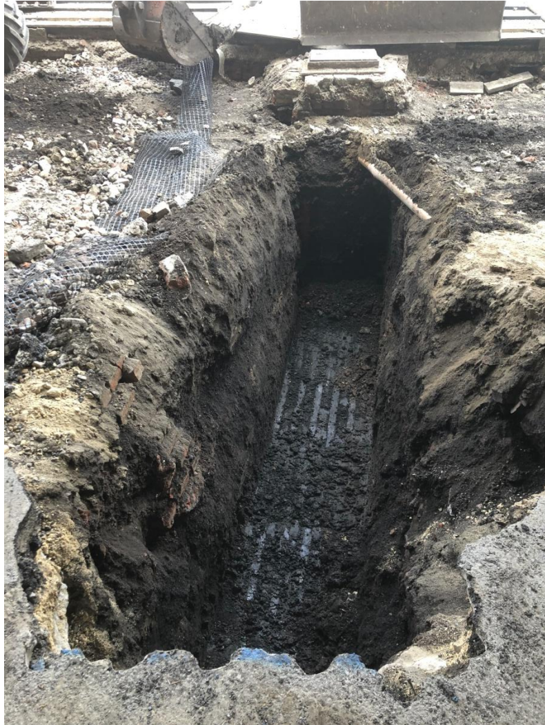
Plate 2 North-east facing view of the machine-excavated drain trench
