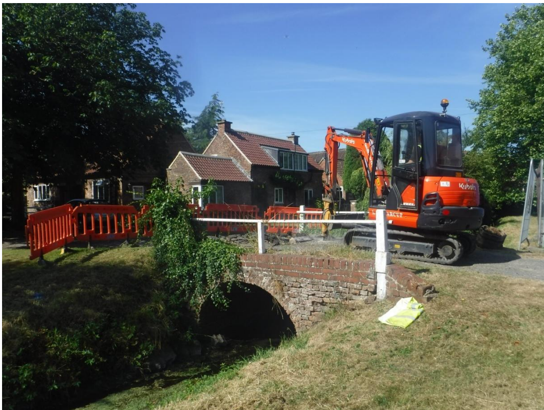
Plate 1. South-west facing view of demolition in progress.
