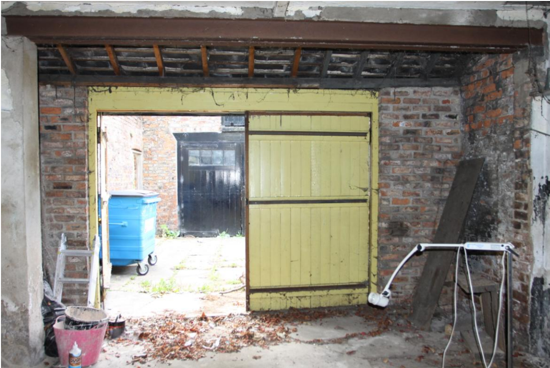
Plate 9 The later porch addition to Building 1, view south.
