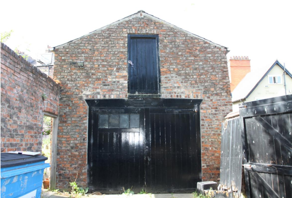
Plate 8 Northern elevation of Building 2, view south.
