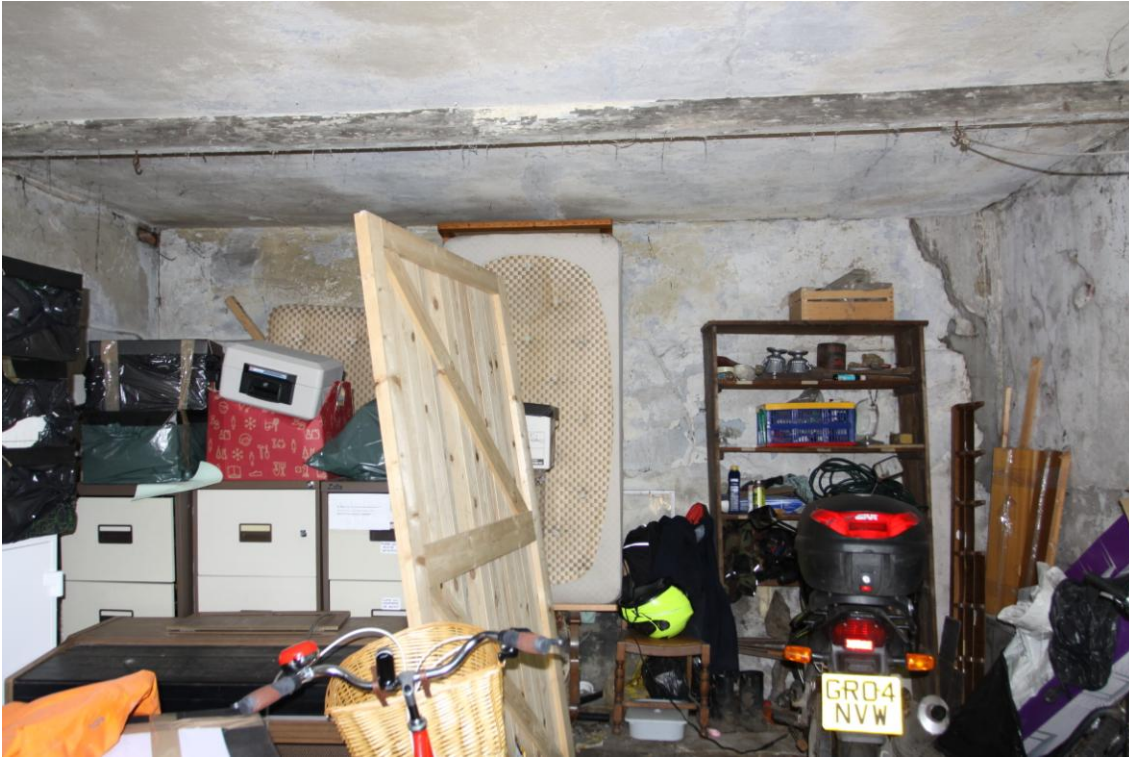
Plate 13 The interior of Building 2, view south.
