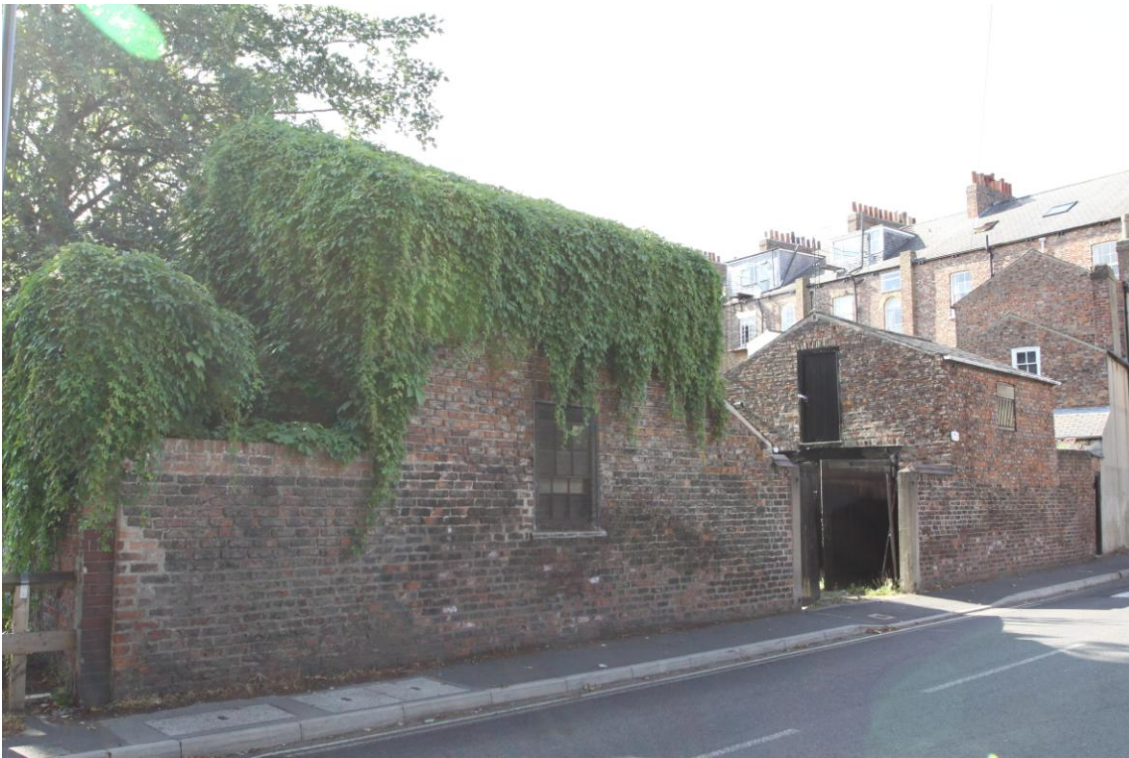
Plate 1 View of Buildings 1 and 2, view south-east.
