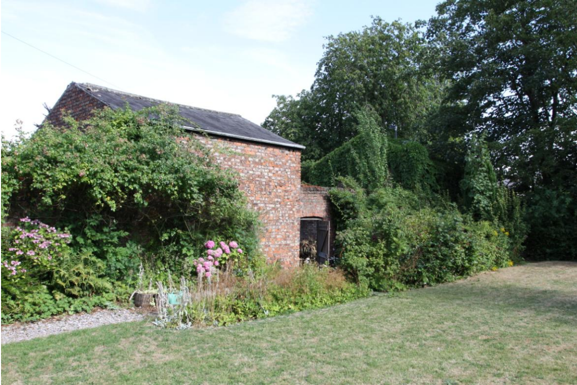
Plate 7 View of the southern and eastern elevations of Building 2, view north-west.
