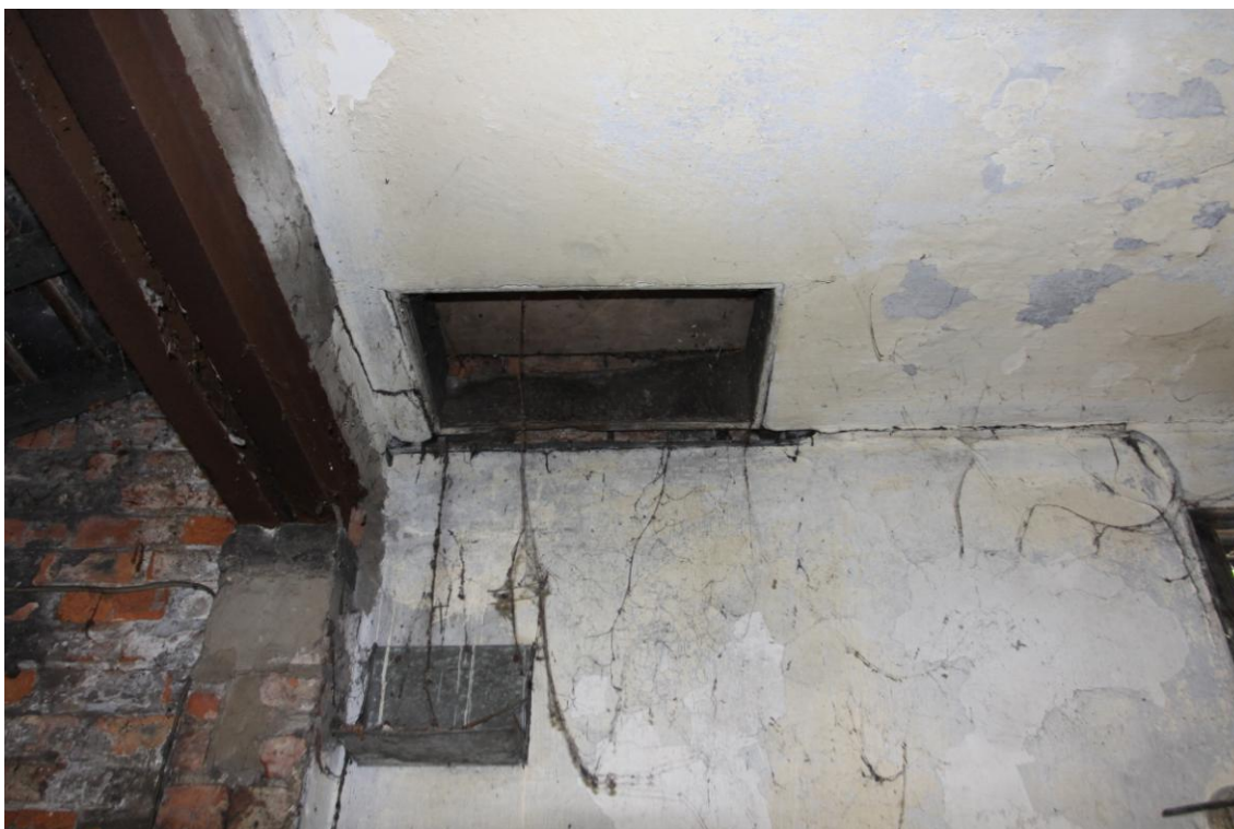
Plate 11 Access to upper storey of Building 1, view west.
