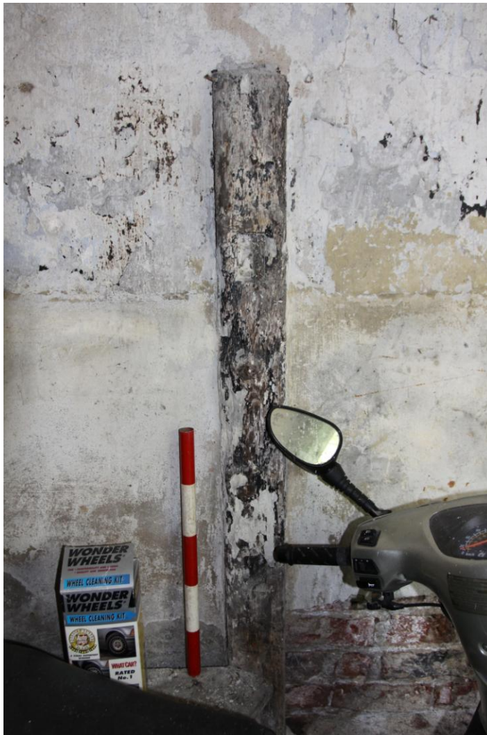
Plate 14 Wooden post and exposed brick wall in Building 2, view west
