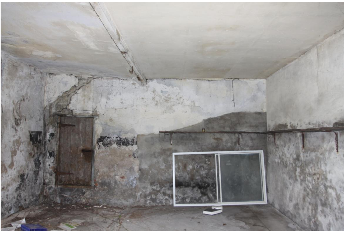
Plate 10 The interior of Building 1, view north.
