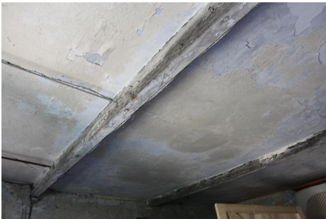
Plate 16 Beams within Building 2, view south-east.
