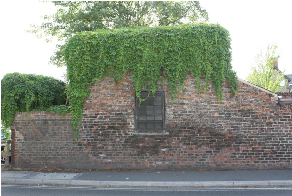
Plate 3 Northern elevation of Building 1, view south.
