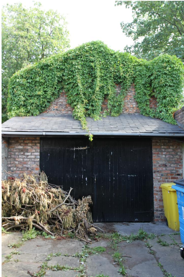
Plate 5 Southern elevation of Building 1, view north.
