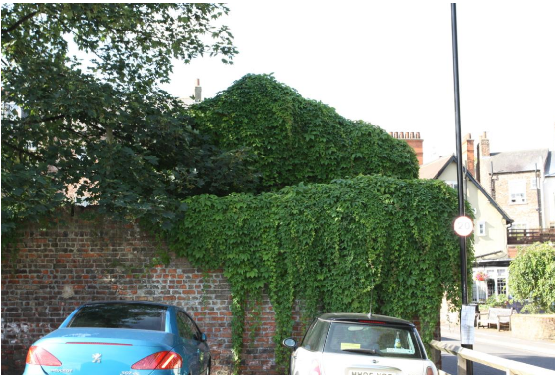
Plate 2 Western elevation of Building 1, view east
