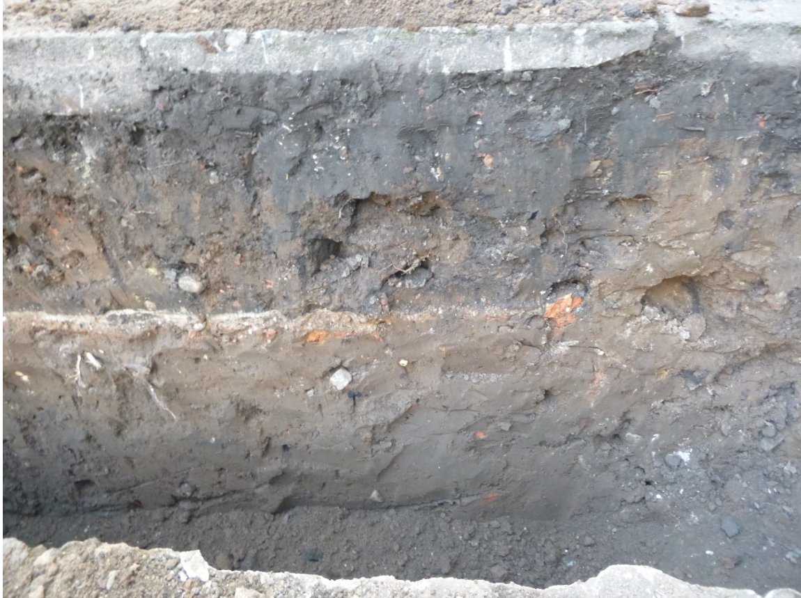
Plate 1 Section of trench behind removed retaining wall. To depth of c.800mm BGL.
