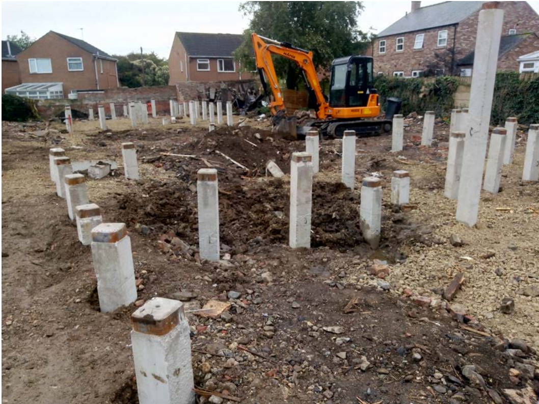
Plate 1 The site after piling, looking east
