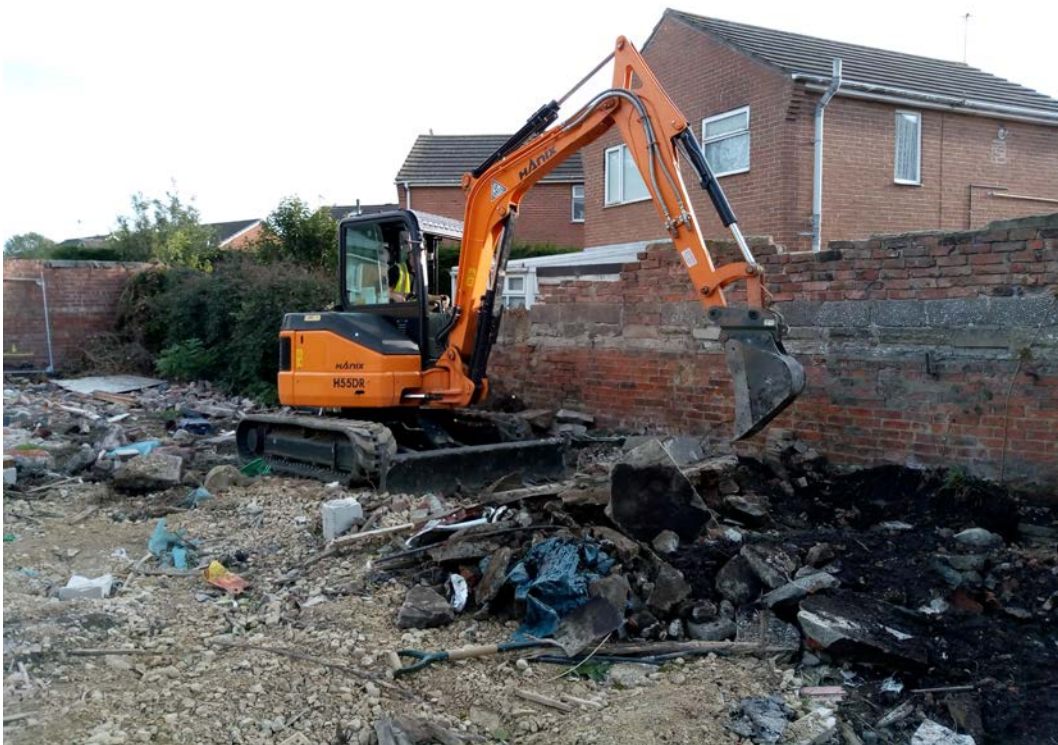
Plate 2 Excavation of eastern footings, looking north-east
