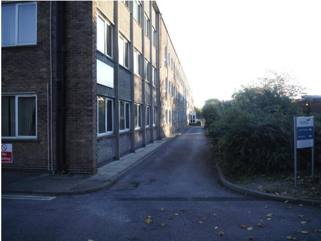
Plate 7 View of the Office building on the Frederick House site, facing east
