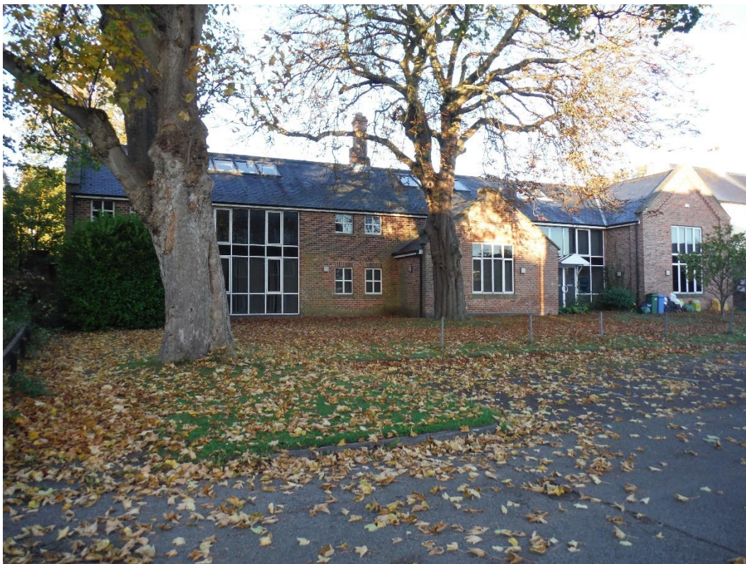
Plate 1 Rear view of Frederick House, facing west
