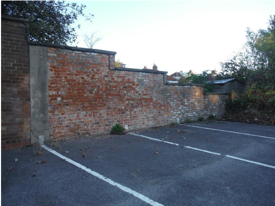
Plate 5 Older boundary wall section, possibly 19th century or earlier, facing north-east.
