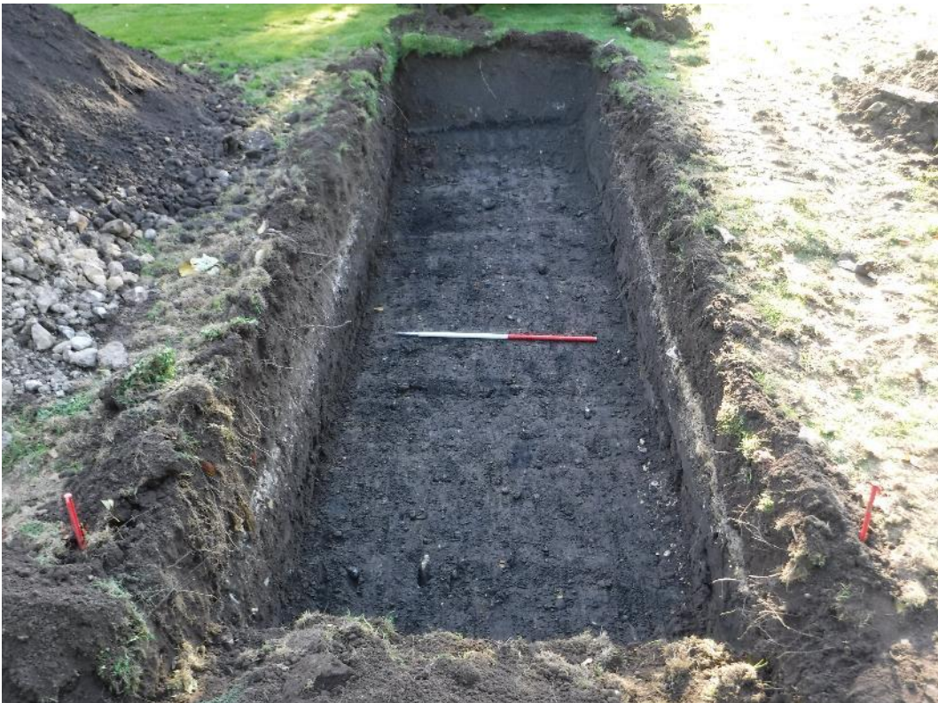
Plate 5 Trench 2 (south), looking south-west
