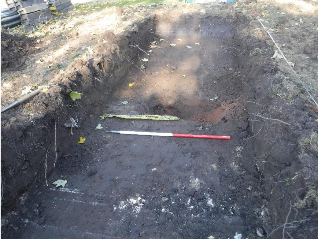
Plate 4 Trench 2 (north) showing low-pressure gas pipe
