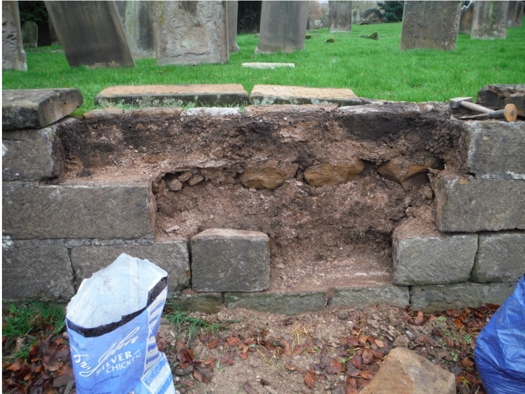
Plate 2. East facing view of the partially dismantled boundary wall.
