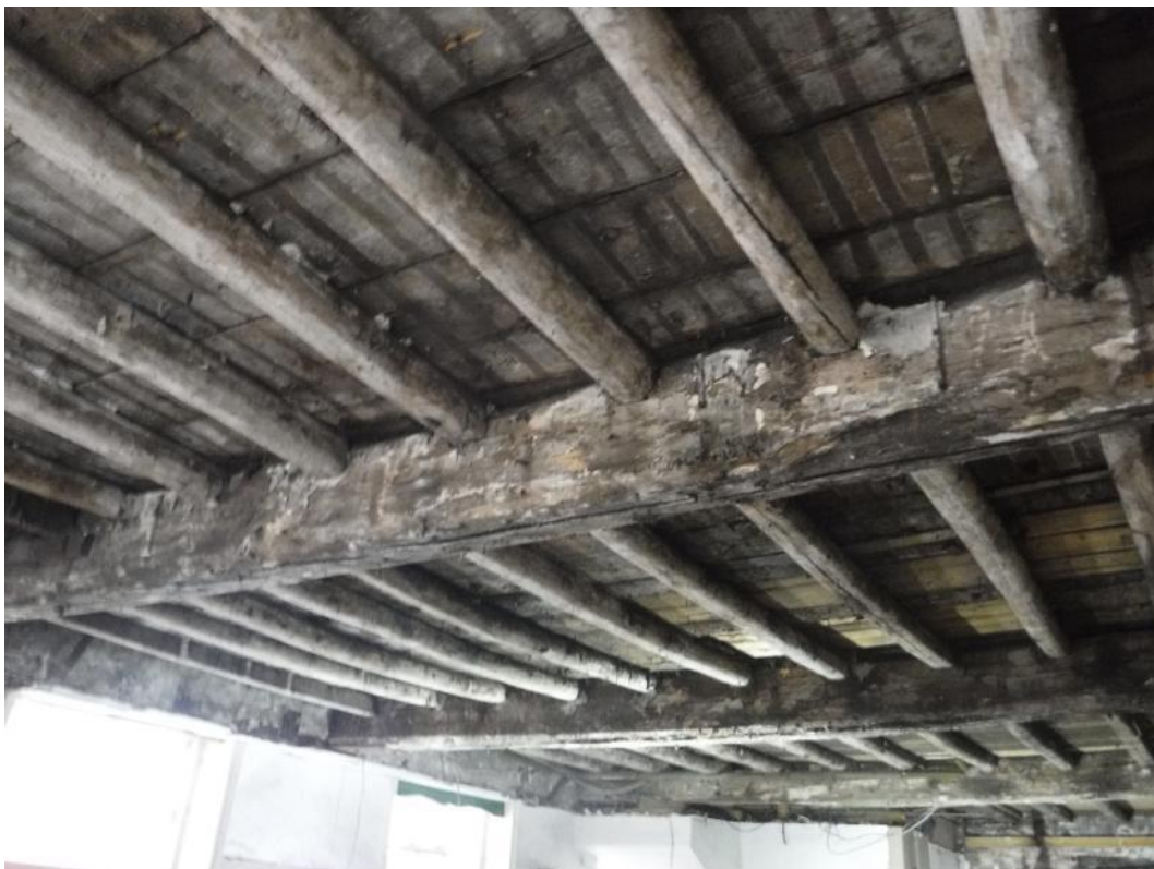
Plate 10 Exposed 17th/18th century beams and joists with floor boards of the first floor above, facing east
