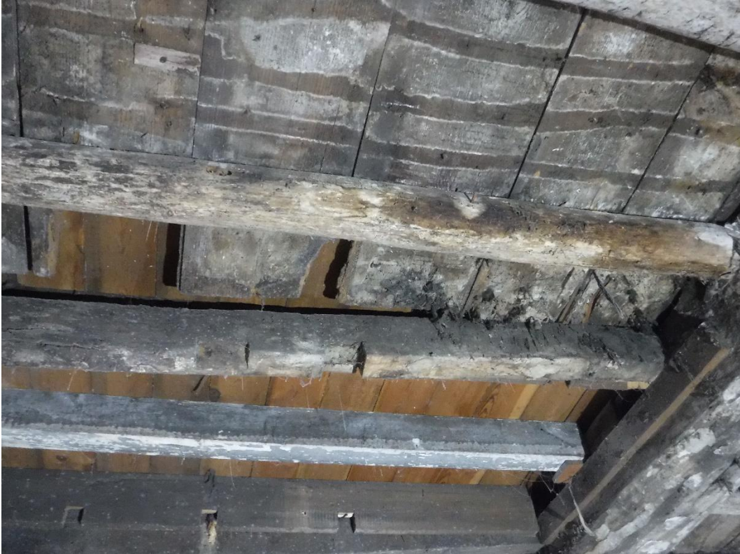
Plate 7 Deteriorated north-eastern ends of early floor boards at northern of the ground floor, note the reused timbers used as joists, looking north-east
