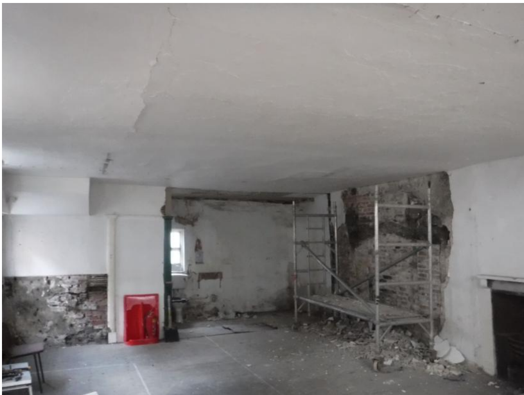
Plate 2 Ground floor 19th century ceiling, facing south
