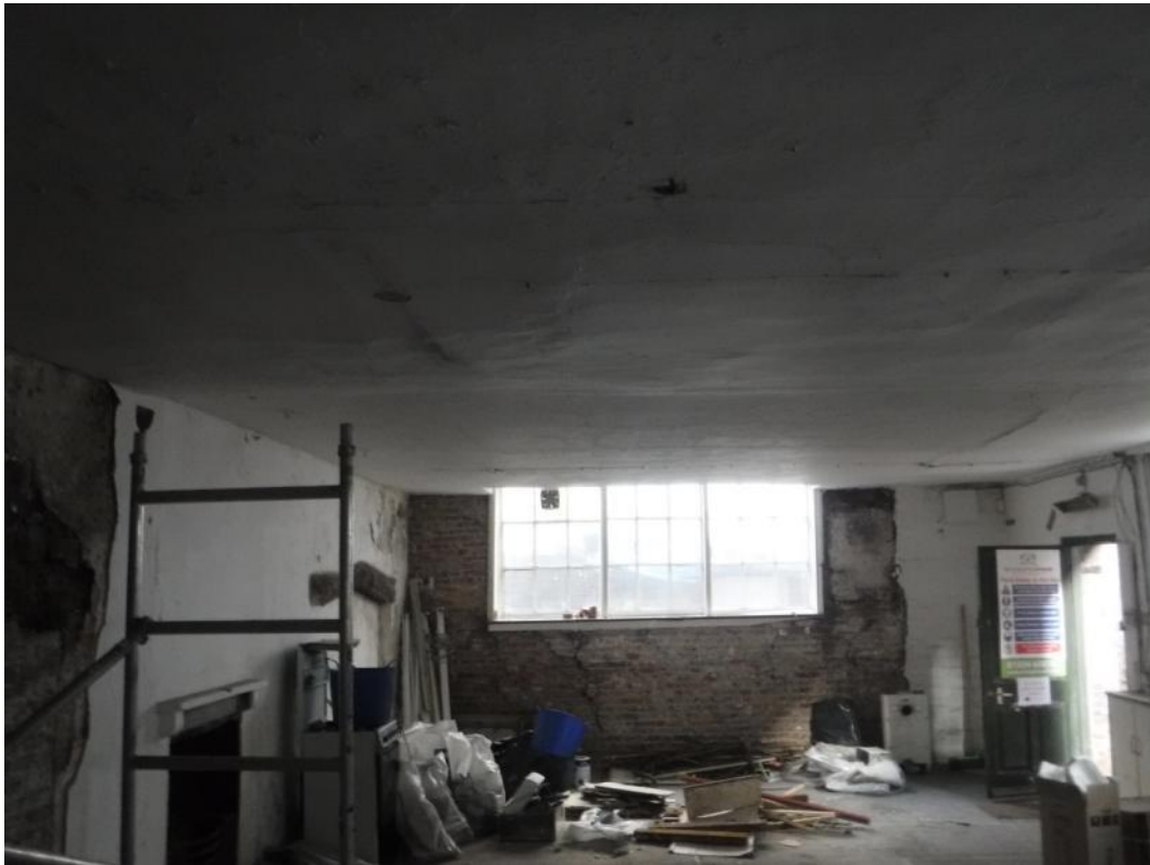
Plate 1 Ground floor 19th century ceiling, facing north-west
