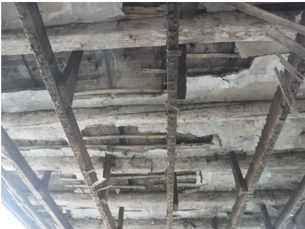
Plate 16 Fragmentary remains of an early lath and plaster ceiling present towards the northern end of the ground floor ceiling, facing north-east
