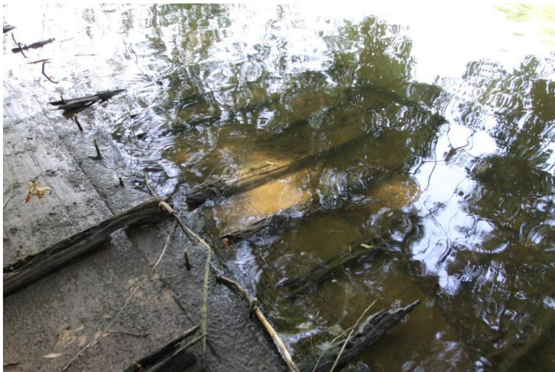
Plate 2. Submerged in situ frame elements. The row of nails are in the keel plank. Looking south west.
