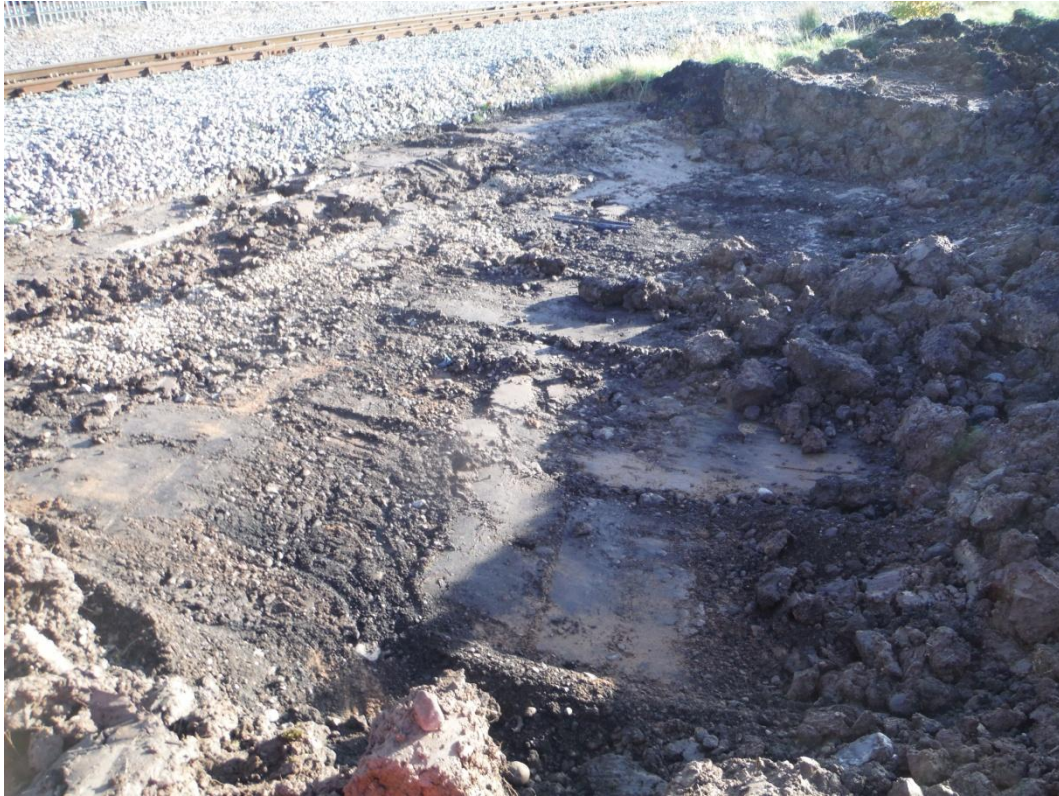
Plate 2 View of ground reduction at the north of development looking east
