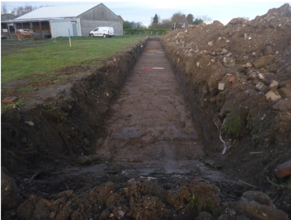
Plate 4 Trench 2, looking NE
