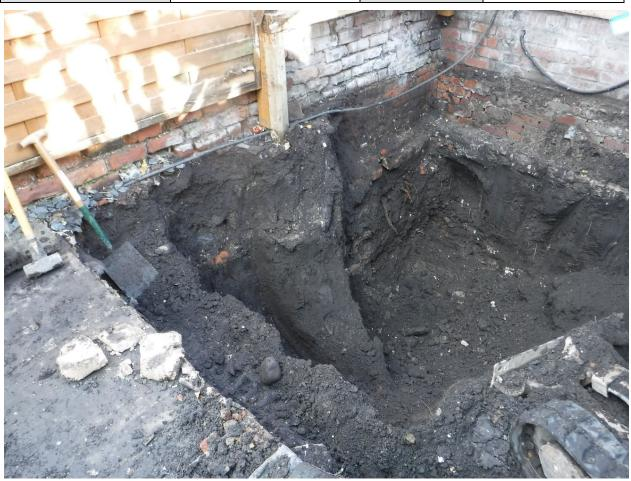
Plate 3 Area stripped to maximum depth of 2.45m below ground level, view east
