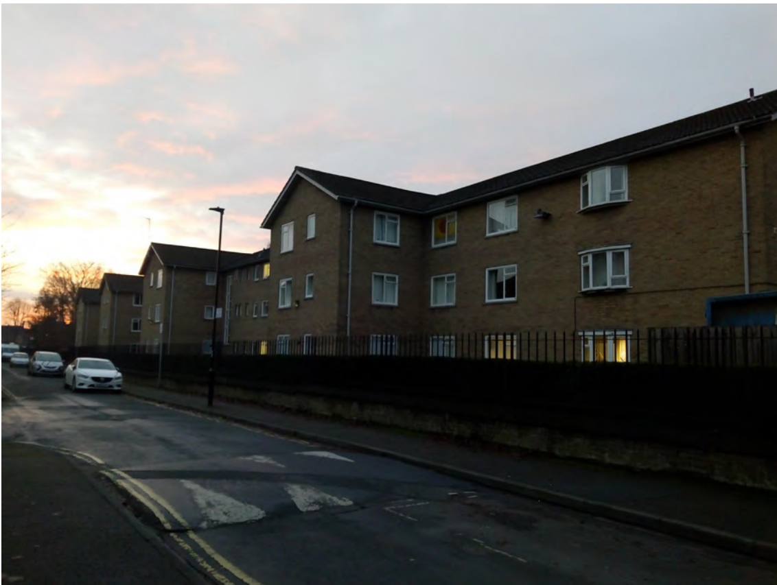
Plate 2 Residences A-G on Garden Street, view south-east
