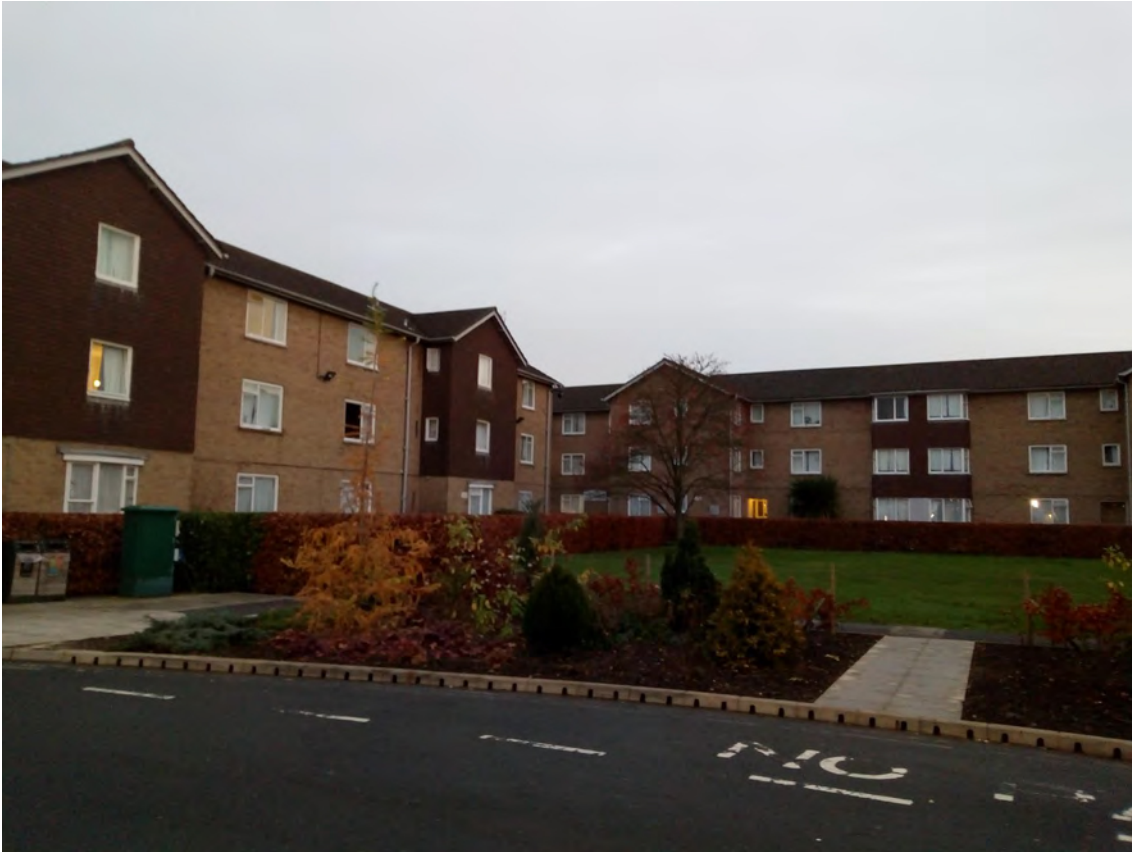
Plate 1 View of the proposed development area, view north-west
