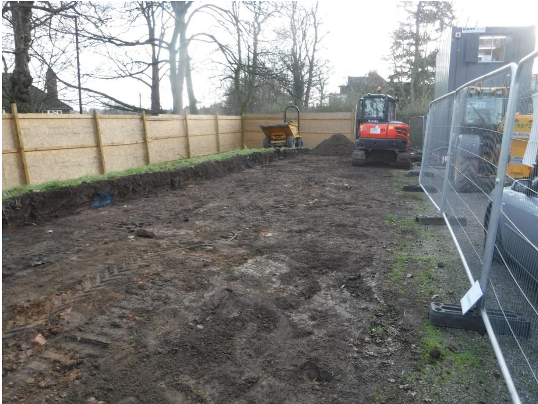
Plate 1 Car park area after topsoil strip
