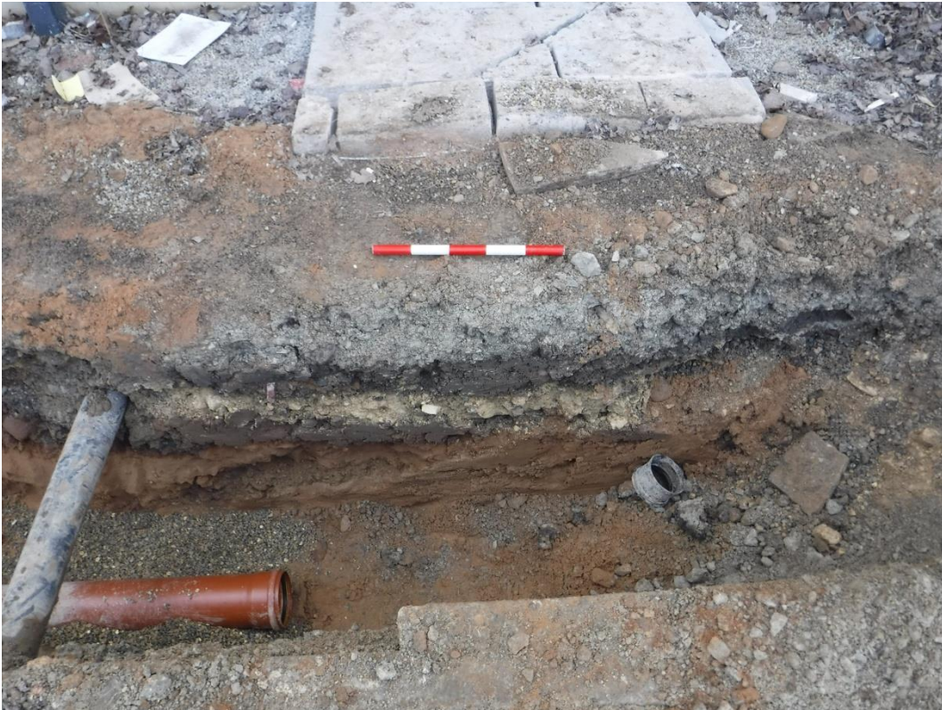
Plate 5 Service trench looking south-west, 0.5m scale
