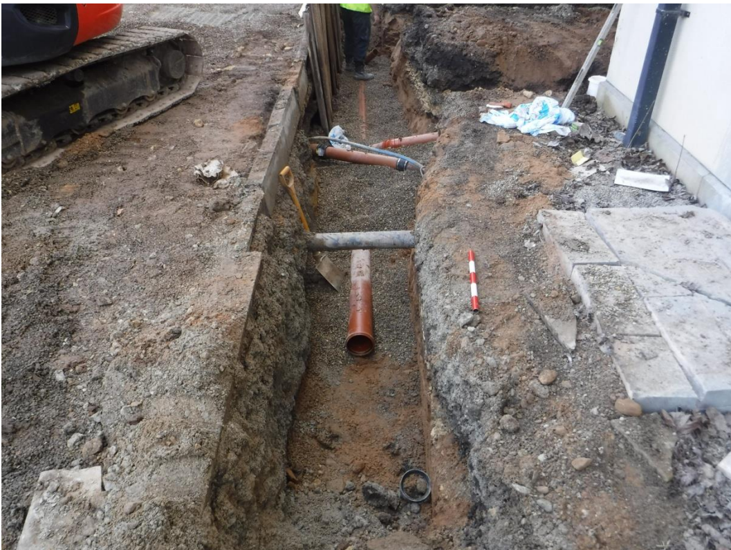
Plate 4 Service trench looking south-east, 0.5m scale
