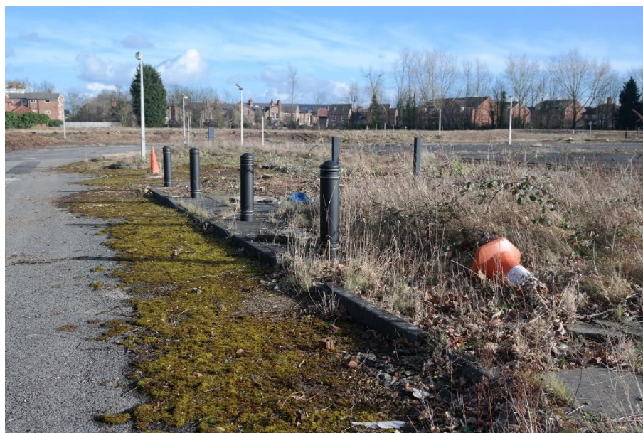
Plate 31 Metal bollards at the edge of the northernmost roadway of Zone D facing east
