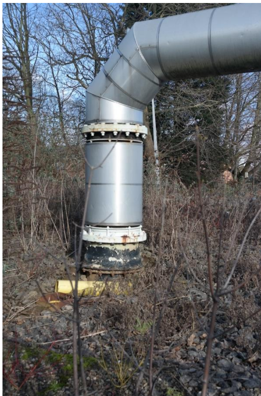
Plate 15 The northern end of the major pipeline in Zone B facing east
