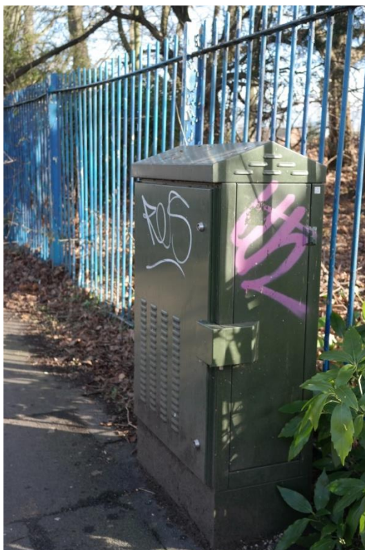
Plate 19 Zone C street frontage facing south-east
