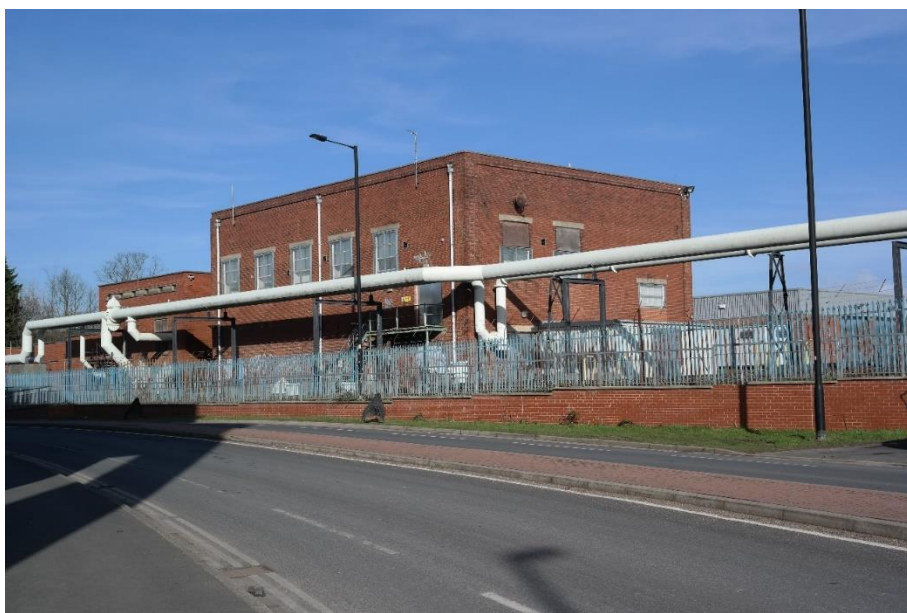
Plate 9 Zone B facing north-east
