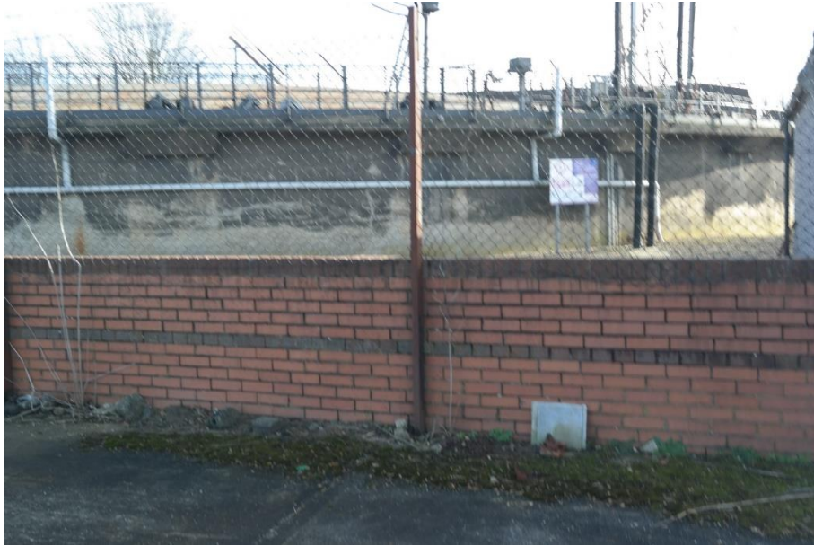
Plate 38 Zone F the gas storage tank facing west
