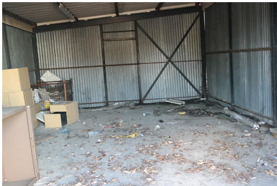
Plate 44 An open metal shed to the west of the gas storage tank facing east
