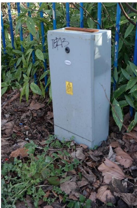
Plate 20 Zone C street frontage facing south-east
