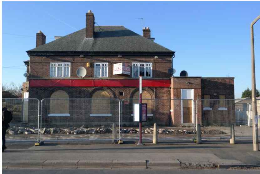
Plate 7 General view of the site facing north-west
