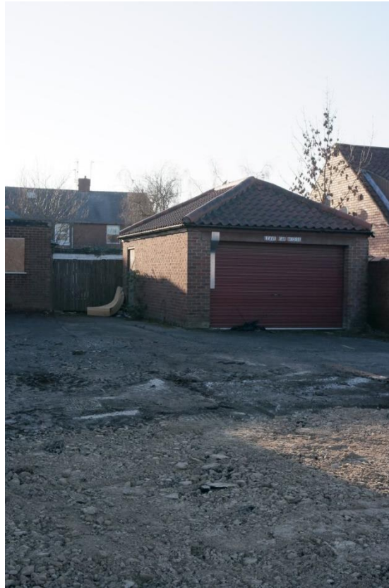
Plate 10 The garage building facing west
