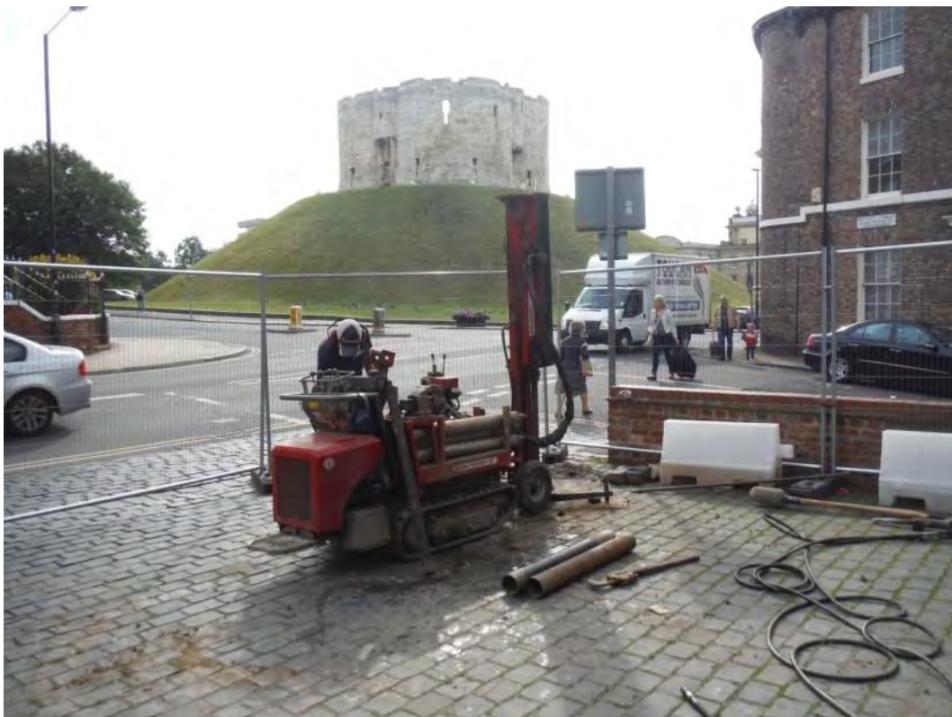
Plate 10 Borehole 1 during drilling
