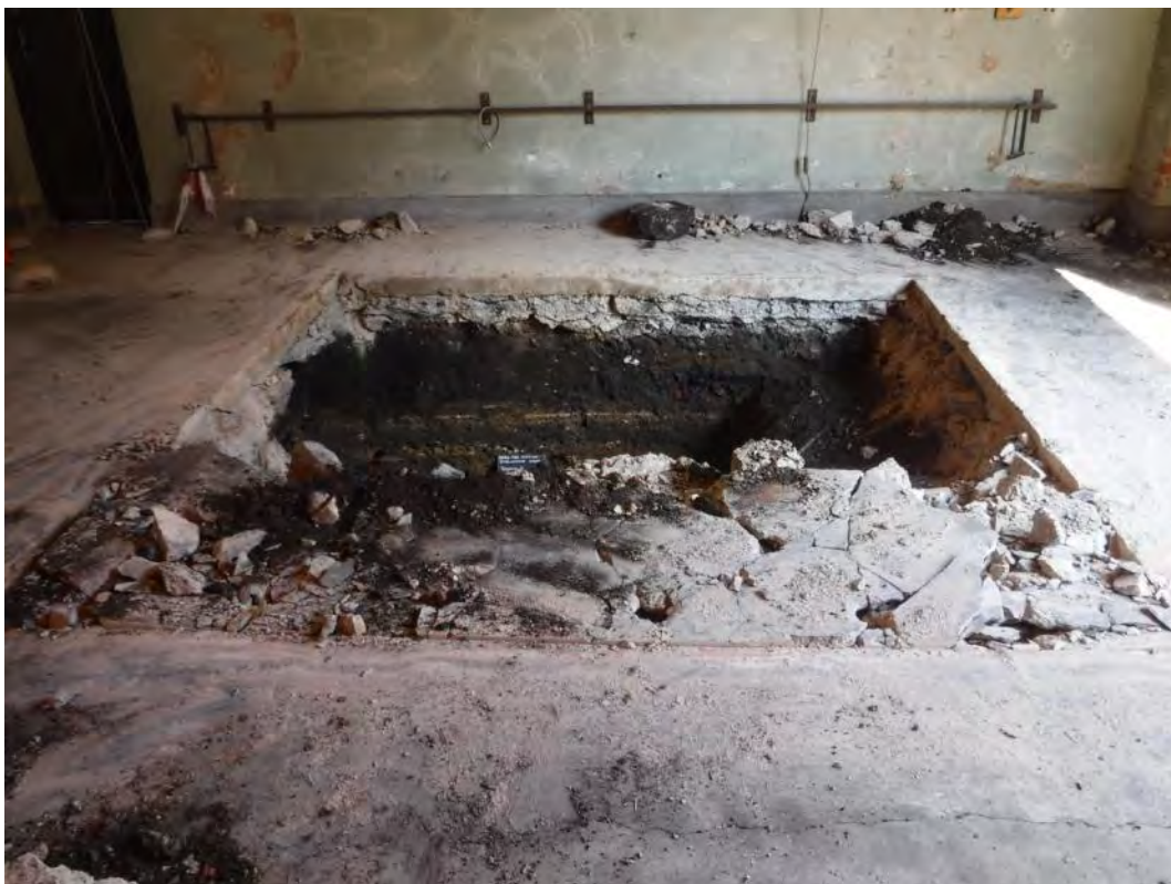
Plate 8 Trench 4 general view looking NE
