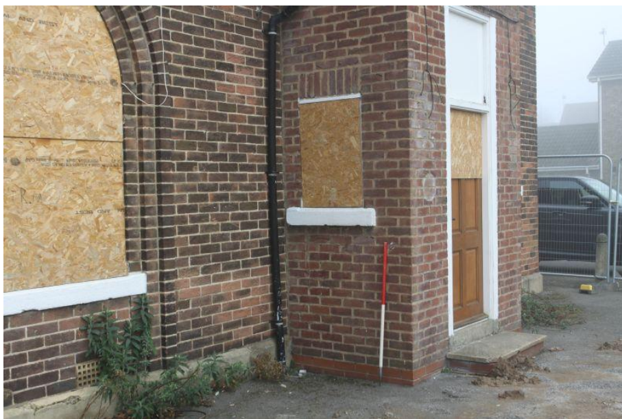
Plate 7 The porch, facing north-east
