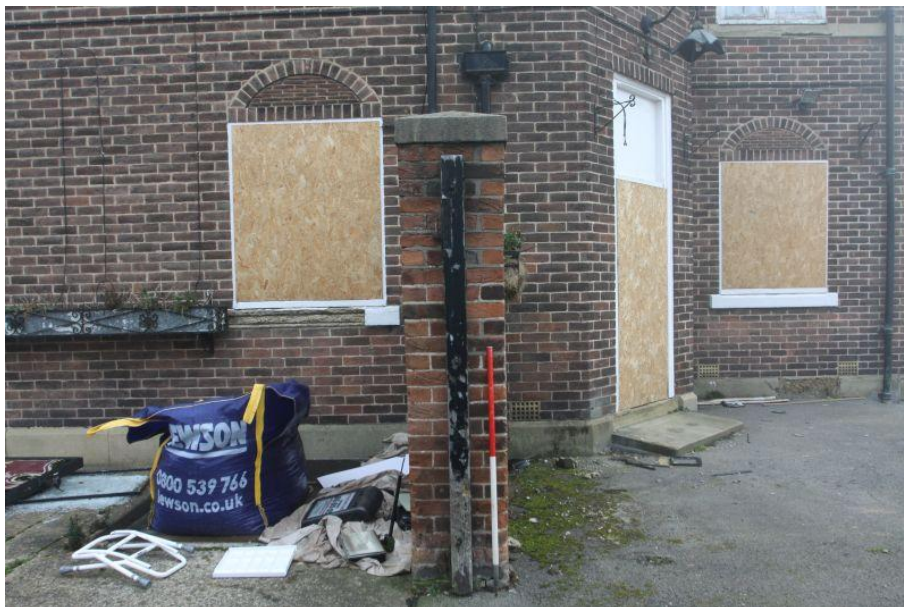
Plate 30 The easternmost gate-post, facing north-east
