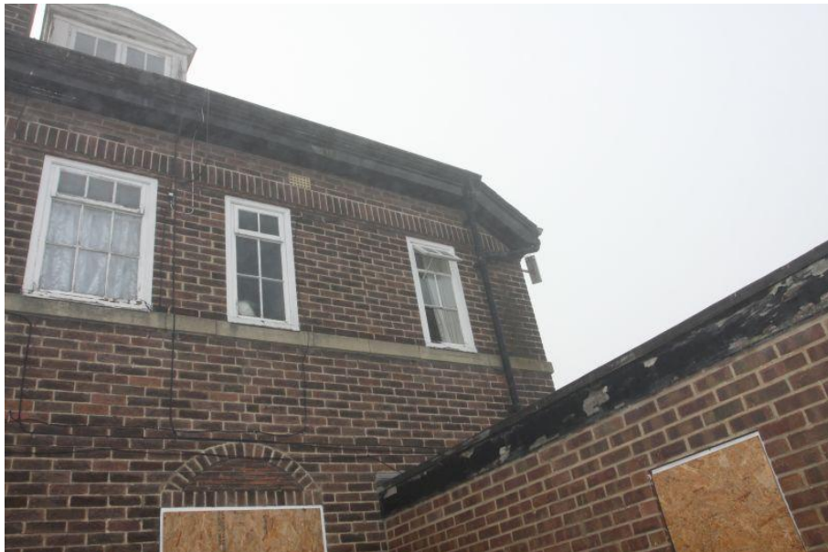
Plate 15 Windows of Design G (left) and H (right), facing south-west
