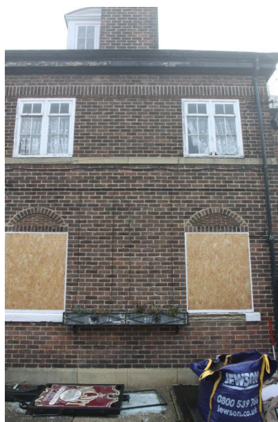
Plate 19 The central portion of the south-western elevation, facing north-east
