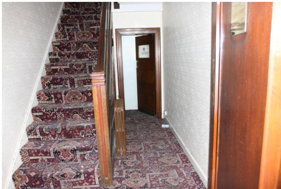
Plate 80 Room I, facing north-west
