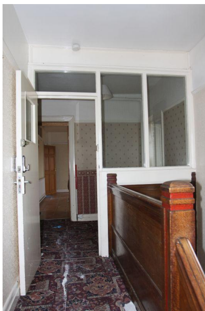
Plate 82 the partition wall at the top of the stairs, facing south-east
