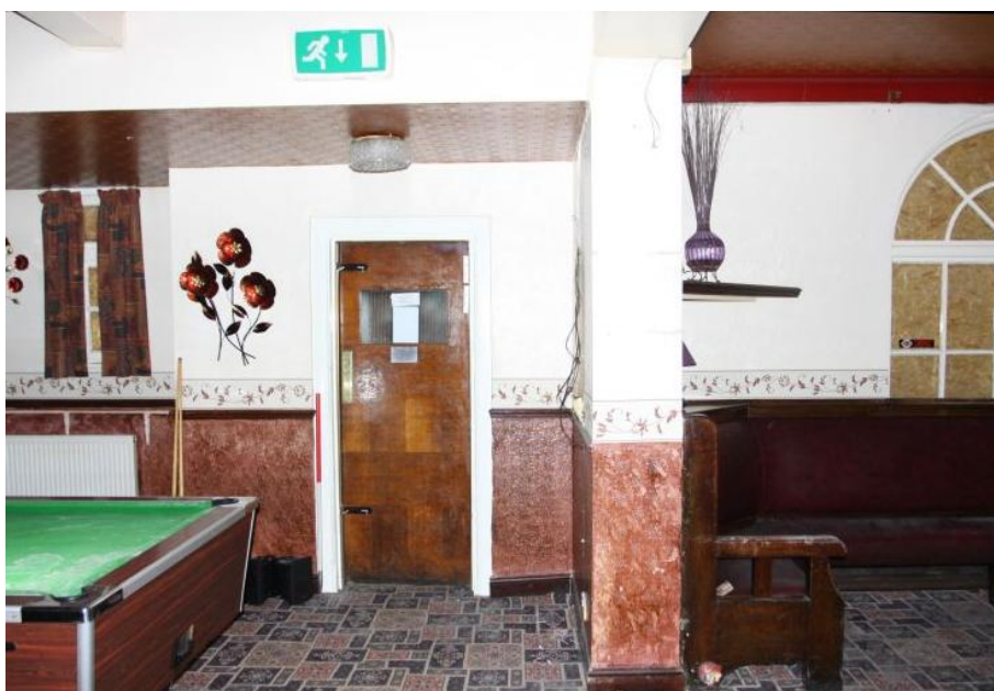
Plate 60 The doorway to the porch in Room C, facing south-east
