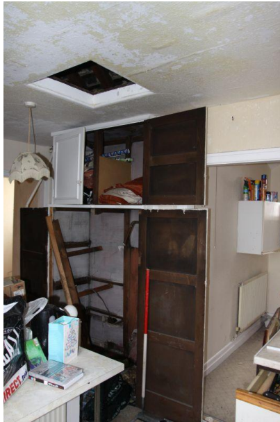
Plate 127 Room X the access hatch for the roof space, facing south-west
