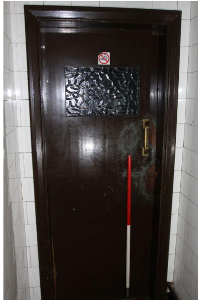
Plate 64 The door between the gents' toilet and Room J, facing south-west
