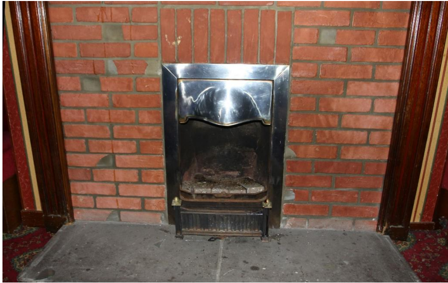
Plate 73 The Room G fireplace hood, facing north-west
