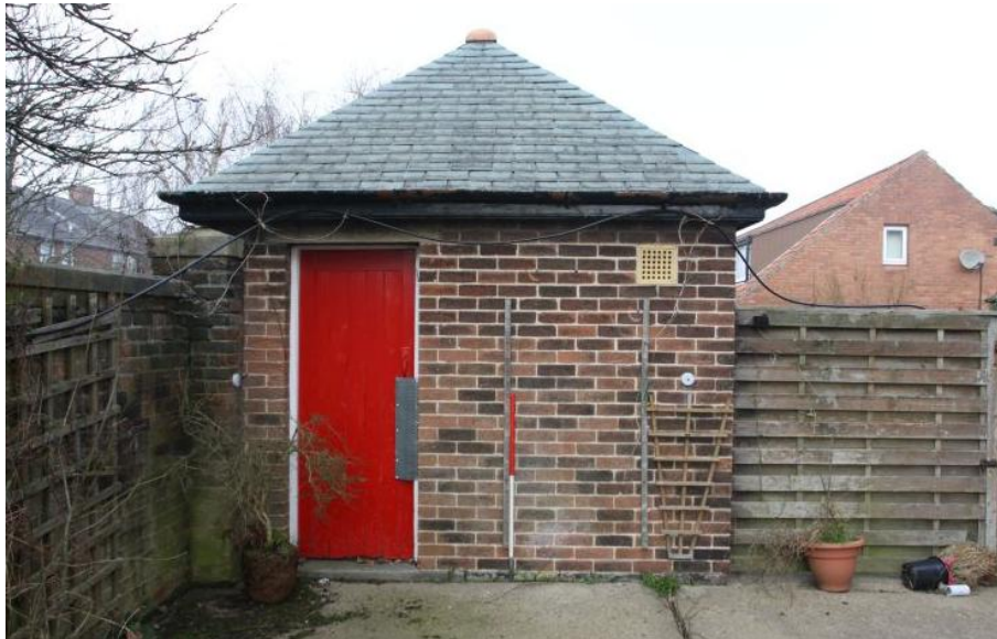
Plate 26 The south-eastern elevation of the outbuilding, facing north-west
