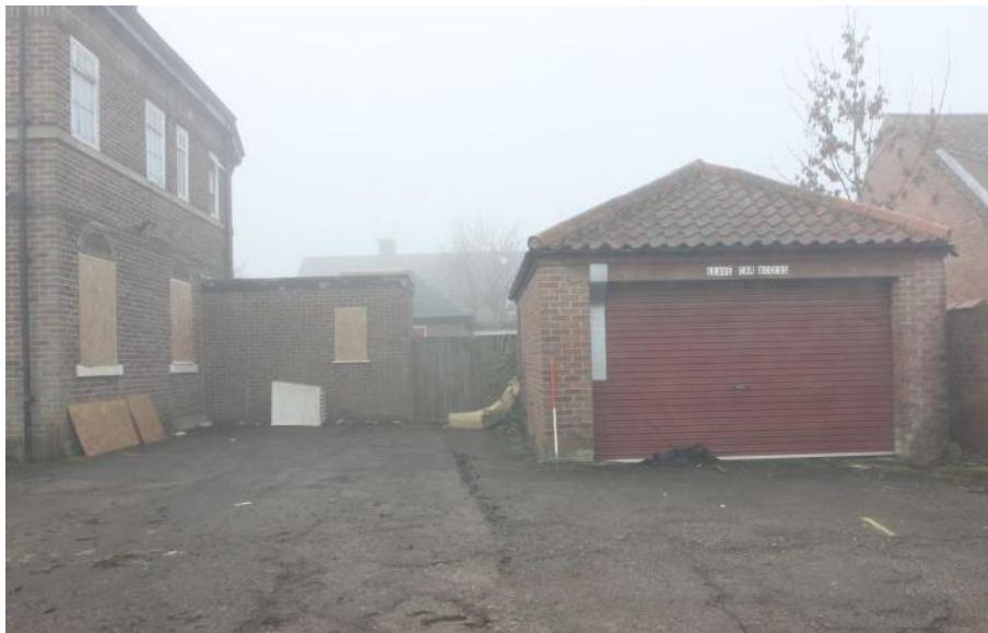
Plate 13 The rear of the public house, facing west
