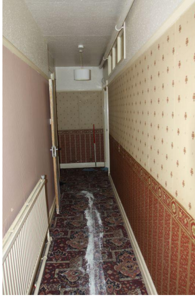
Plate 97 Room M the central portion of the corridor, facing south-east
