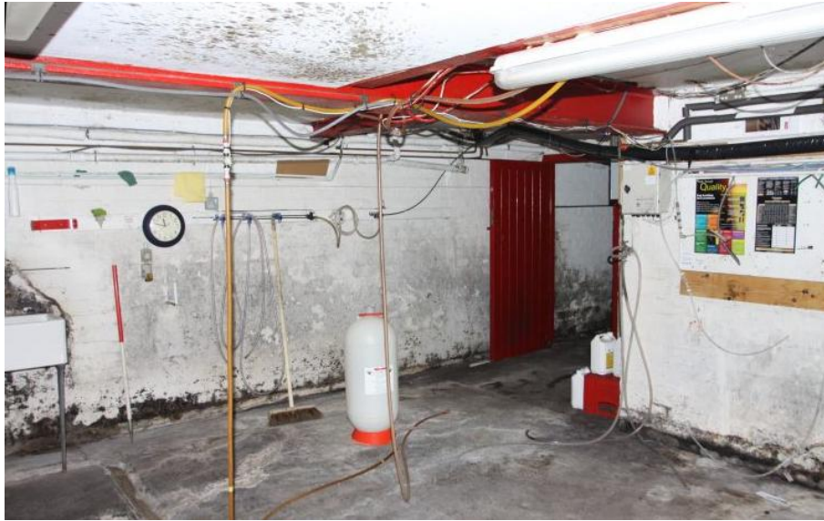
Plate 40 Room C2, facing north-east
