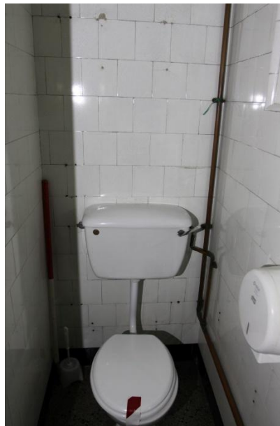
Plate 67 the gents' toilet facing north-west
