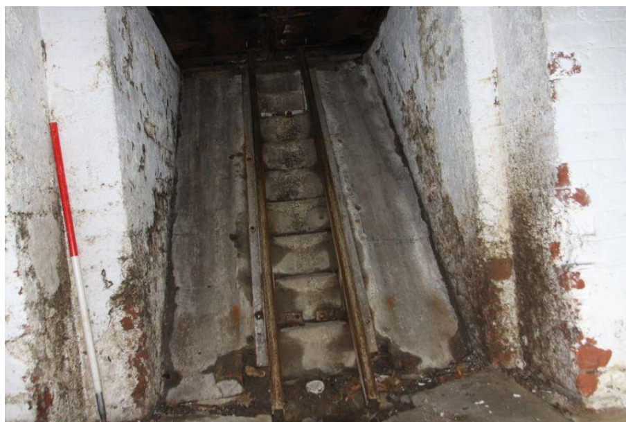
Plate 35 Room C1 barrel chute, facing south-west
