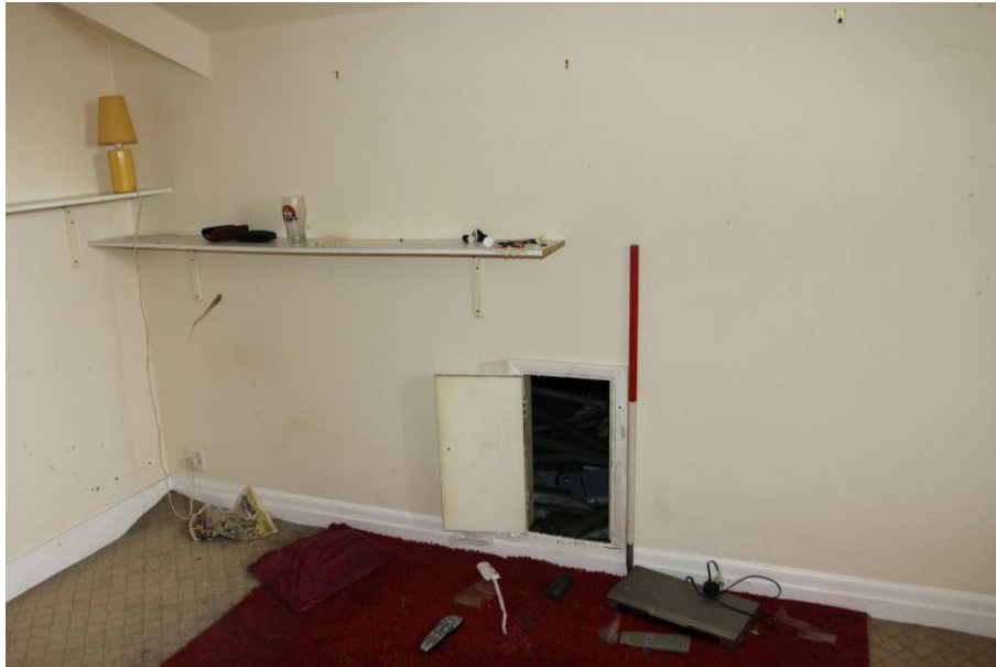
Plate 131 Room Y, facing south-west
