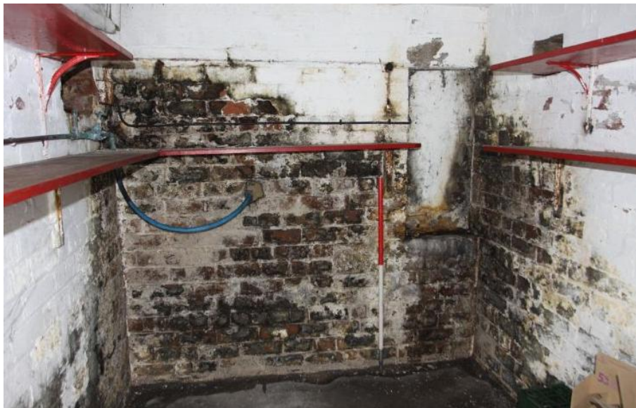
Plate 37 Room C2 facing south-east
