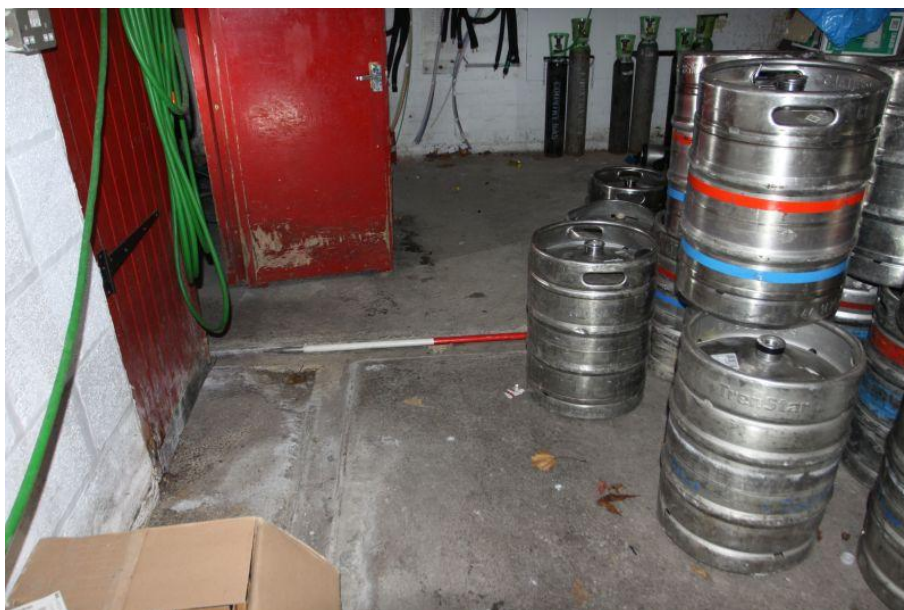
Plate 33 Room C1 floor drainage channels, facing south-east
