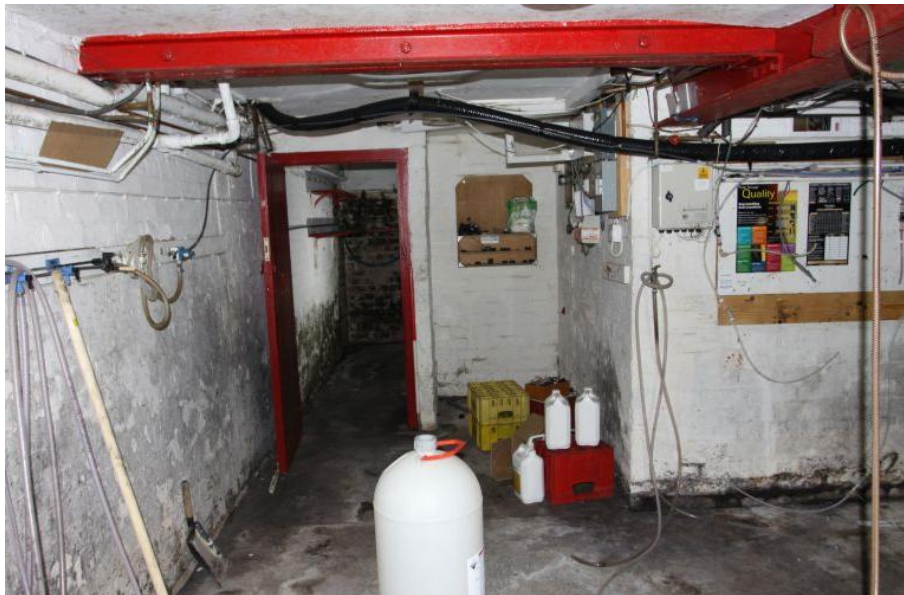
Plate 41 Room C2, facing south-east
