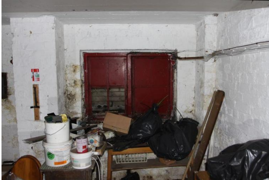
Plate 36 Room C1 window, facing south-west
