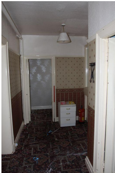
Plate 100 The northern end of Room M, facing south-west
