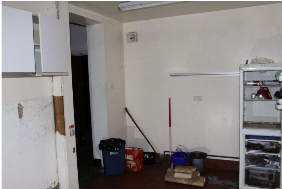
Plate 70 the south-western end of Room E, facing south-west
