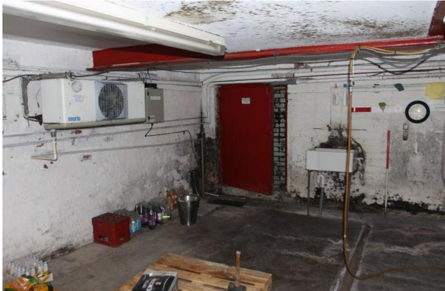
Plate 38 Room C2, facing north
