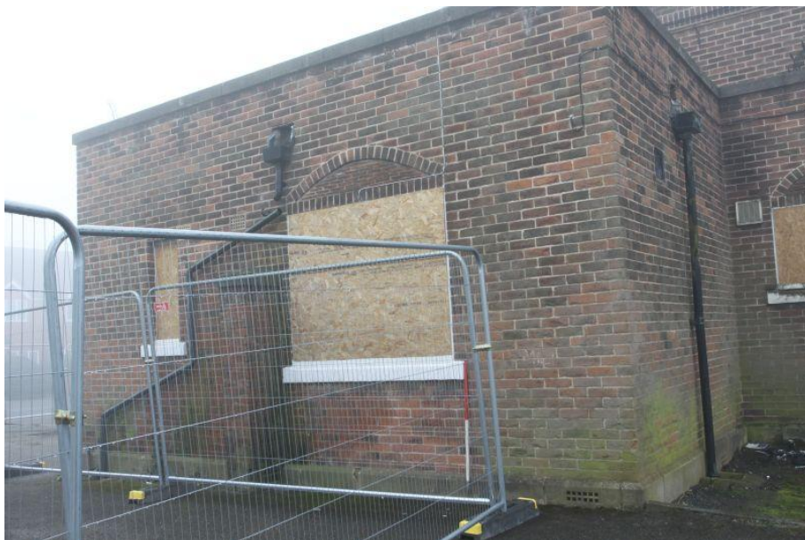
Plate 10 The north-eastern elevation of the southernmost single-storey building, facing south-west
