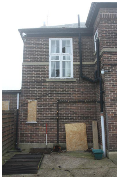
Plate 17 The northern portion of the south-western elevation, facing north-east
