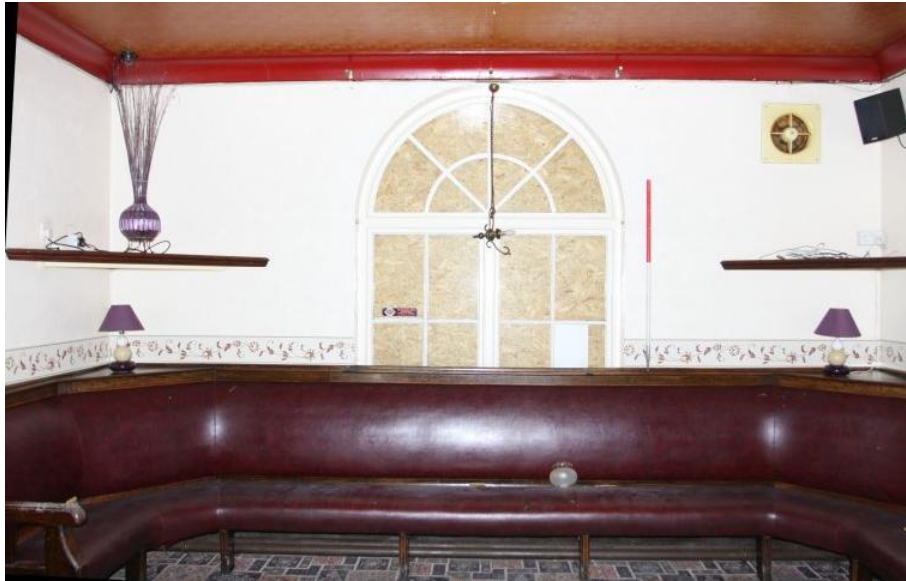
Plate 59 The arched window in Room C, facing south-east
