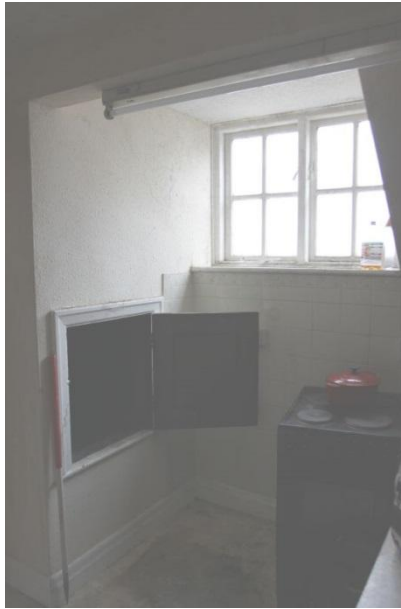
Plate 123 Room X the dormer window and cubby hole, facing north
