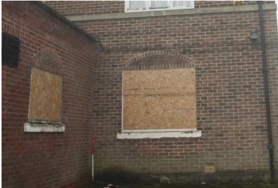
Plate 9 Window Design D, facing south-west
