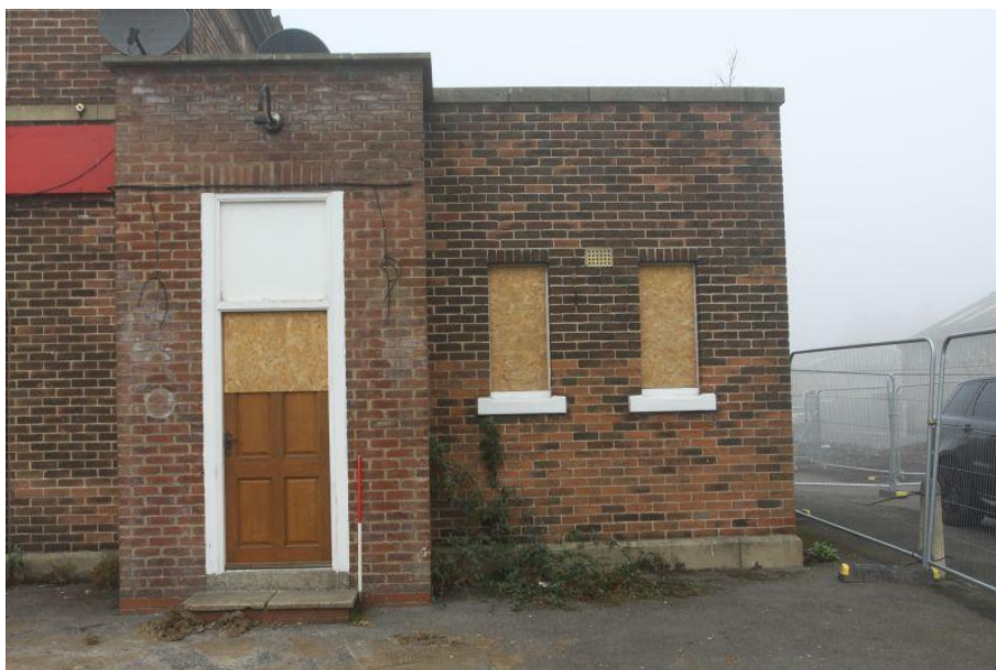
Plate 5 The single storey portion of the street frontage, facing north-west
