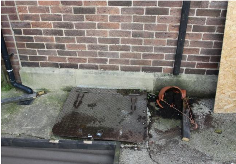
Plate 18 The hatch above the coal-cellar chute facing north-east
