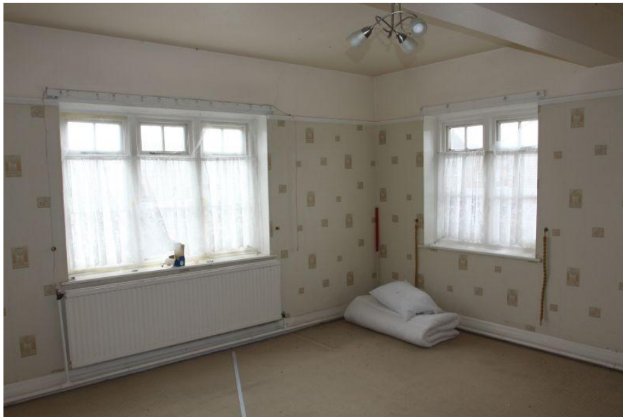
Plate 92 Room L, facing south
