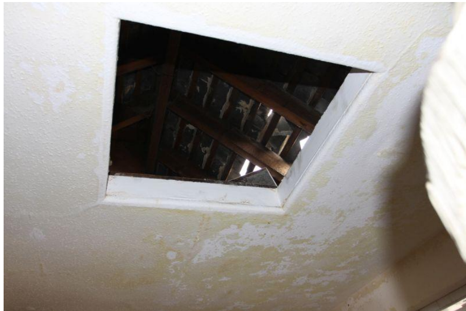
Plate 128 Room X the access hatch for the roof space facing north
