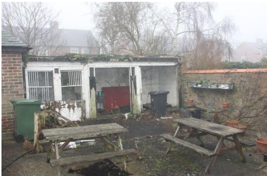
Plate 27 The yard, facing west
