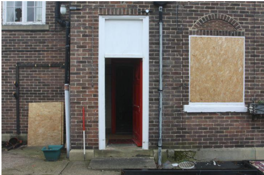
Plate 23 The door on the central portion of the south-western elevation, facing north-east
