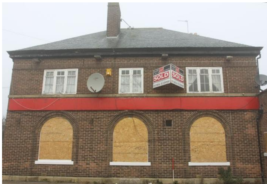
Plate 1 The front elevation facing, north-west
