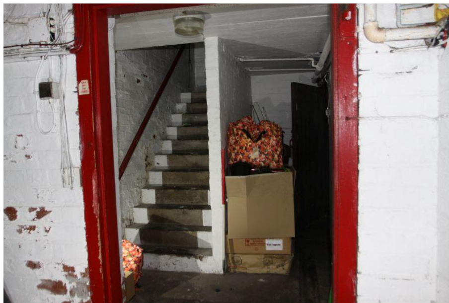
Plate 34 Room C1 entry, facing north-west
