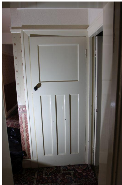
Plate 96 Room M the cubby-hole door, facing south-west
