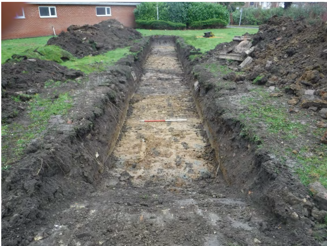
Plate 11 Trench 3 looking west. Scale unit 1.0m
