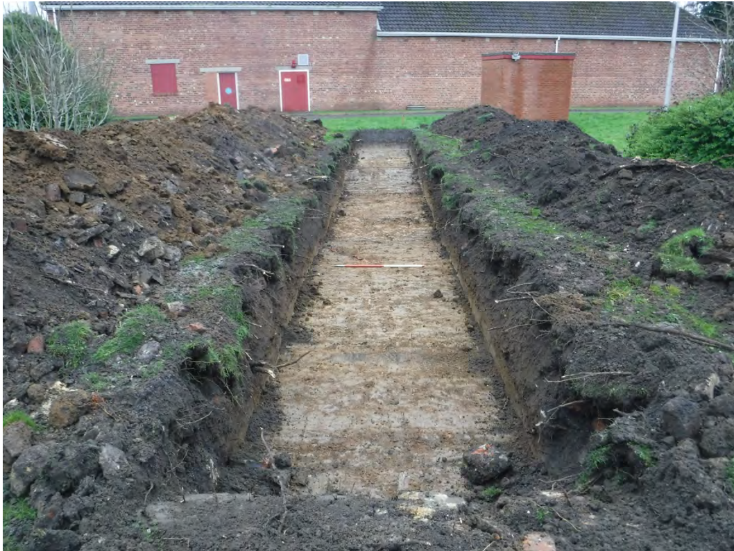
Plate 8 Trench 2 looking south-east. Scale unit 1.0m
