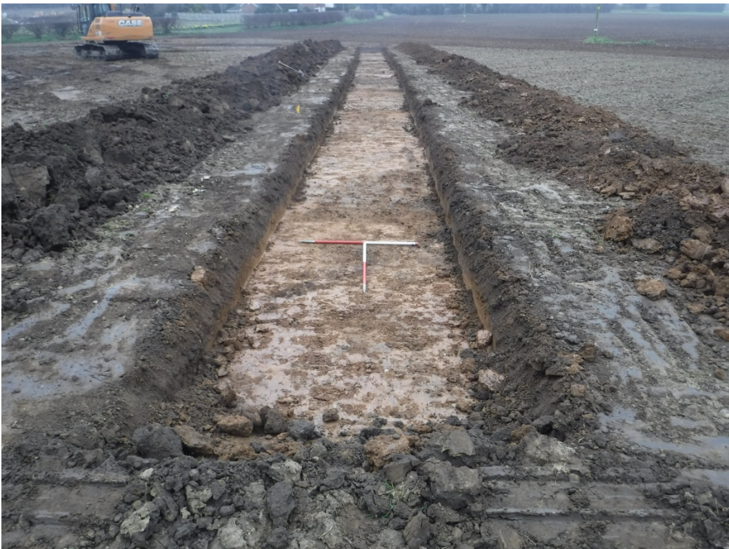
Plate 24 Trench 5, looking south-east. Scale unit 1.0m.
