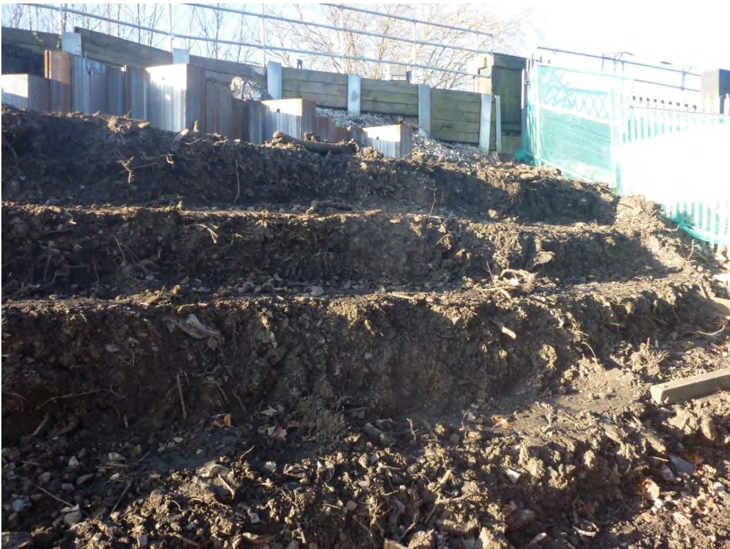
Plate 6 Stepping in the embankment post-installation of the sheet piling
