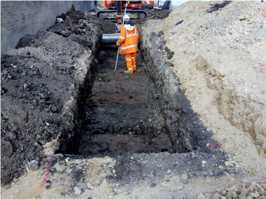
Plate 11 Excavation of foundation trench in Marygate Car Park
