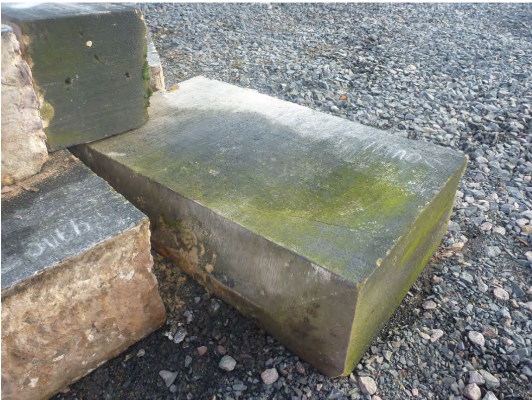
Plate 18 Example of masonry from the later phase of the abutments and pier. Features the pitched top with a hipped edge
