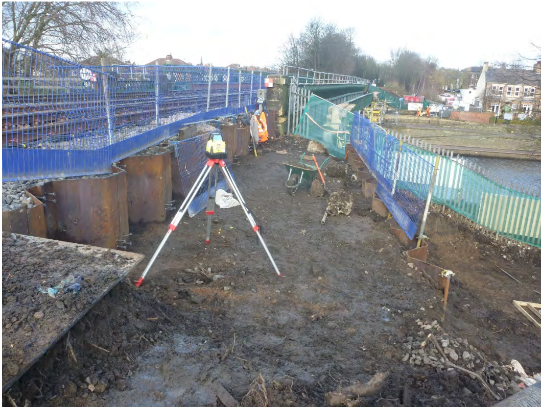
Plate 1 Overview of Sheet Piling and Scarborough Bridge
