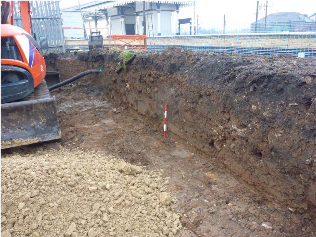
Plate 5 Depth and extent of excavations for the cycle and accessibility path
