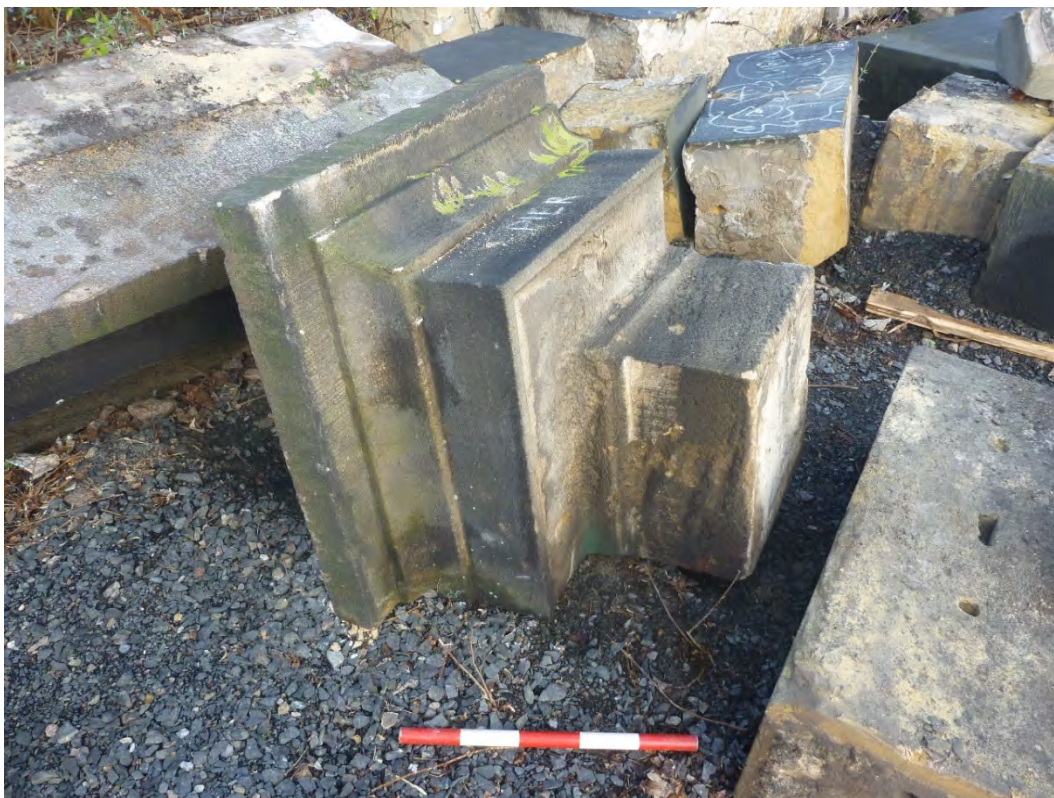
Plate 16 Example of stone from the cornice course of the original abutments and pier. Dated to 1845
