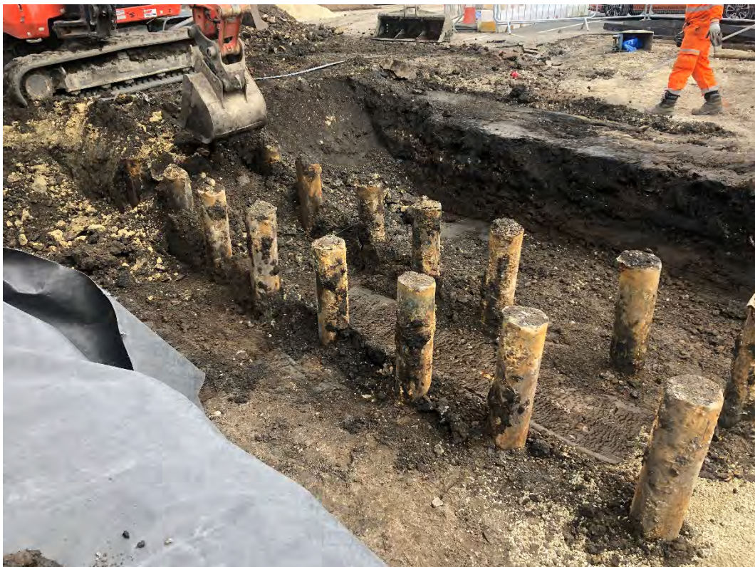
Plate 14 The two lines of lines associated with earlier bridge alterations
