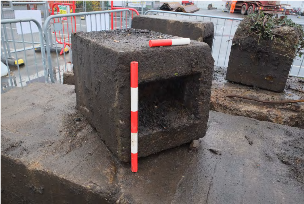
Plate 3 Notch in concrete stanchion, possibly for a timber post
