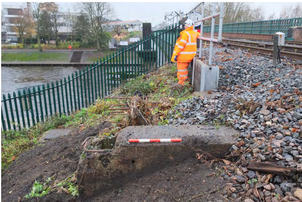
Plate 2 In-situ concrete stanchions on north bank
