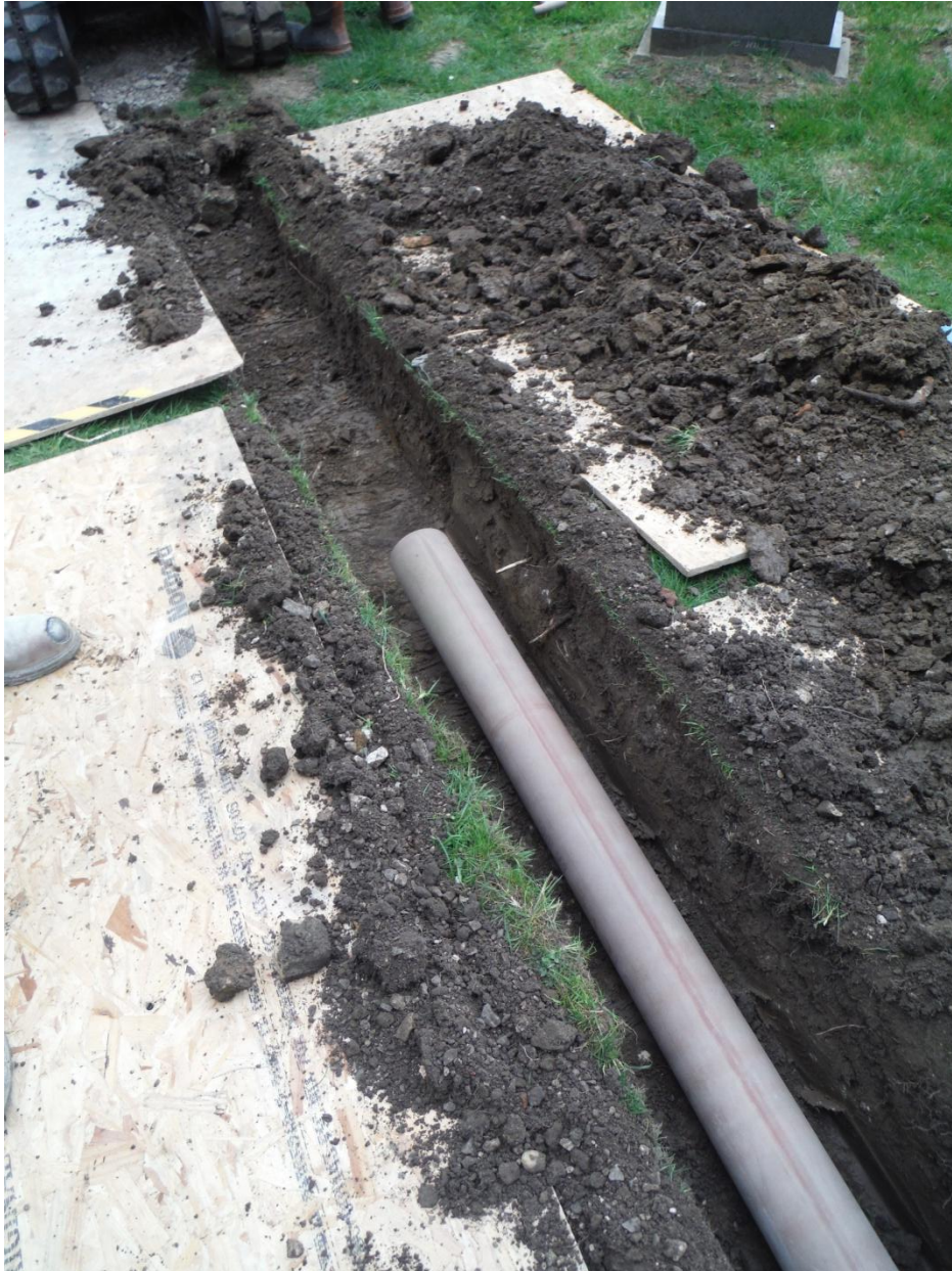
Plate 1 North-east facing view of drain trench
