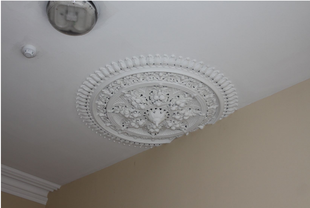
Plate 17 Bedroom 1 ceiling rose
