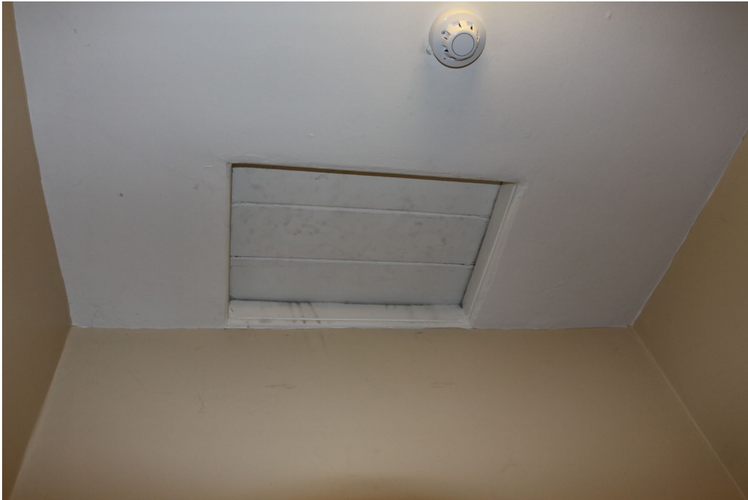
Plate 23 Attic access from second floor corridor
