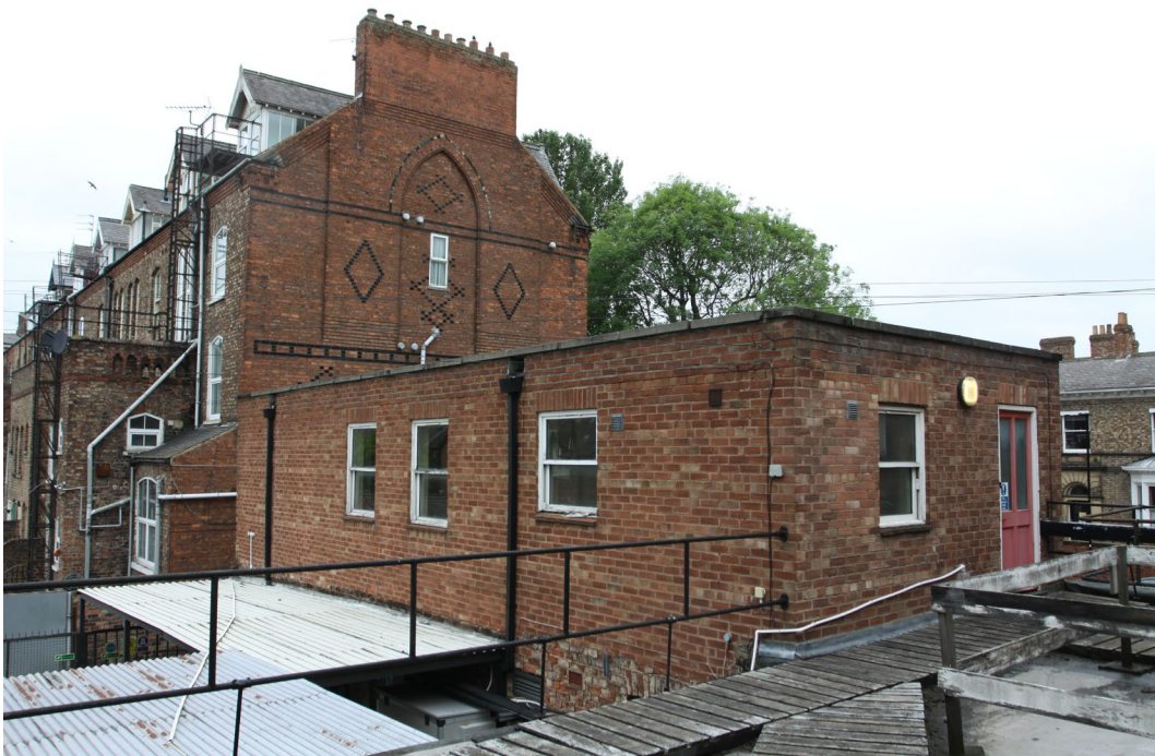
Plate 6 20 th century two-storey building to rear of 212-214 Fulford Road, view north-west
