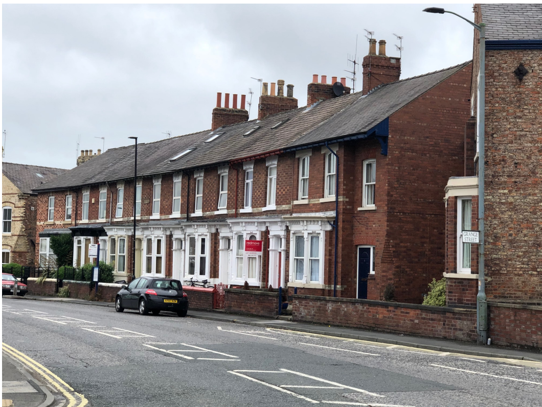
Plate 32 Terraces on Fishergate (within Fulford Road Conservation Area) with velux windows, view north
