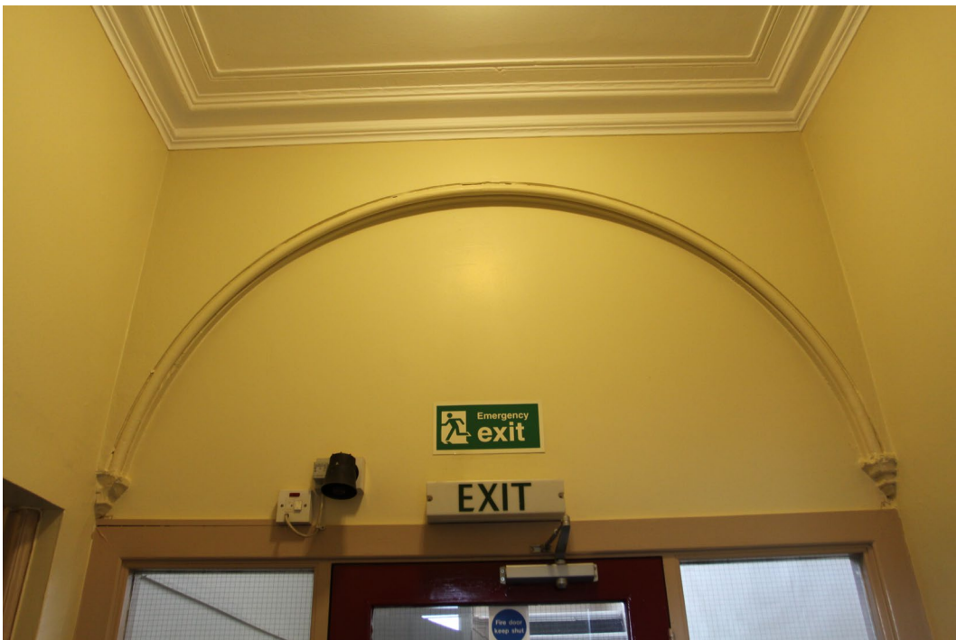
Plate 20 Stairwell leading to second floor
