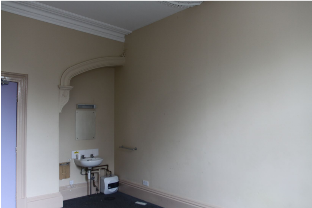
Plate 15 Bedroom 1 with dividing wall
