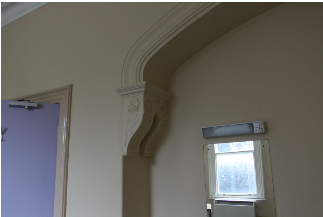
Plate 16 Bedroom 1 arch moulding
