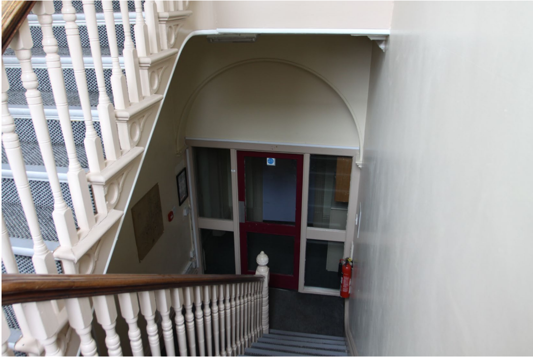
Plate 21 Staircase between first and second floors
