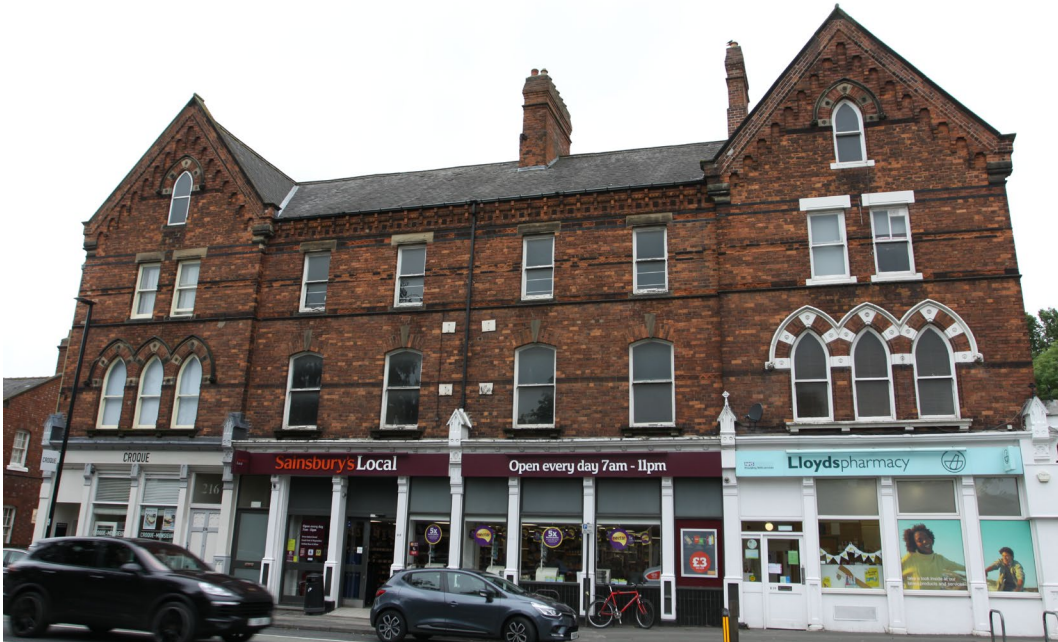
Plate 1 East facing elevation, view west
