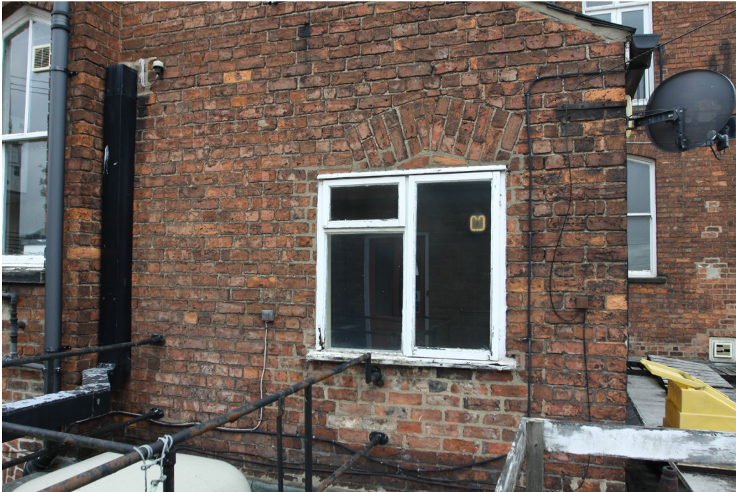
Plate 3 West elevation first floor replacement window, view east
