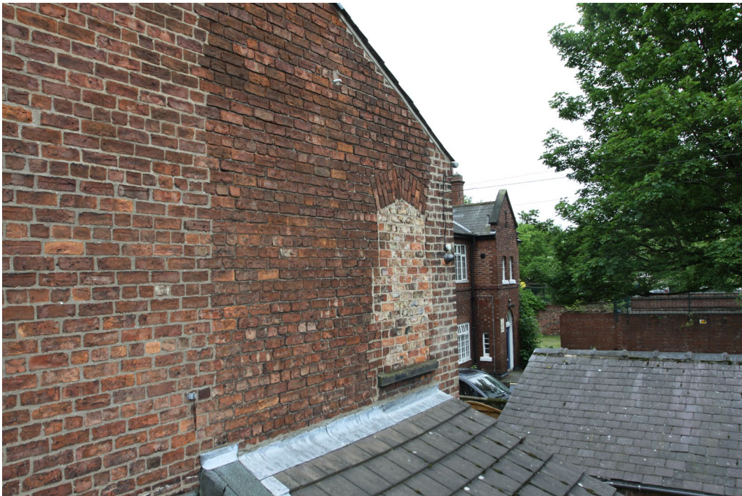
Plate 4 West elevation first floor bricked up window, view south-east
