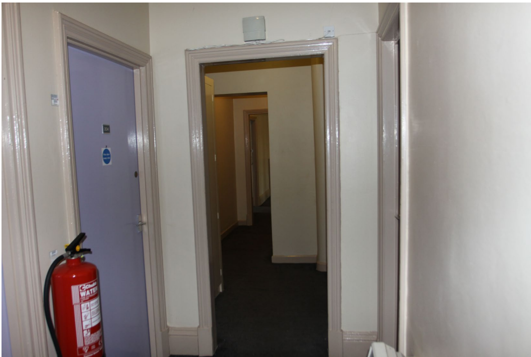
Plate 22 Second floor corridor across 212 and 214 Fulford Road
