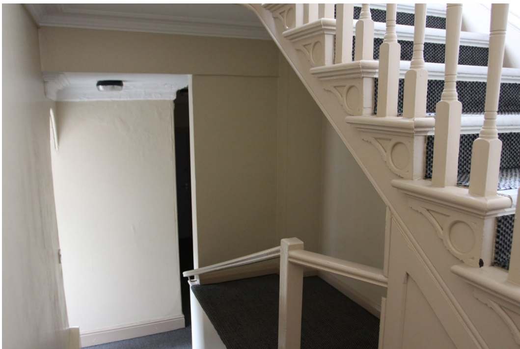
Plate 10 Stairwell in 212 Fulford Road
