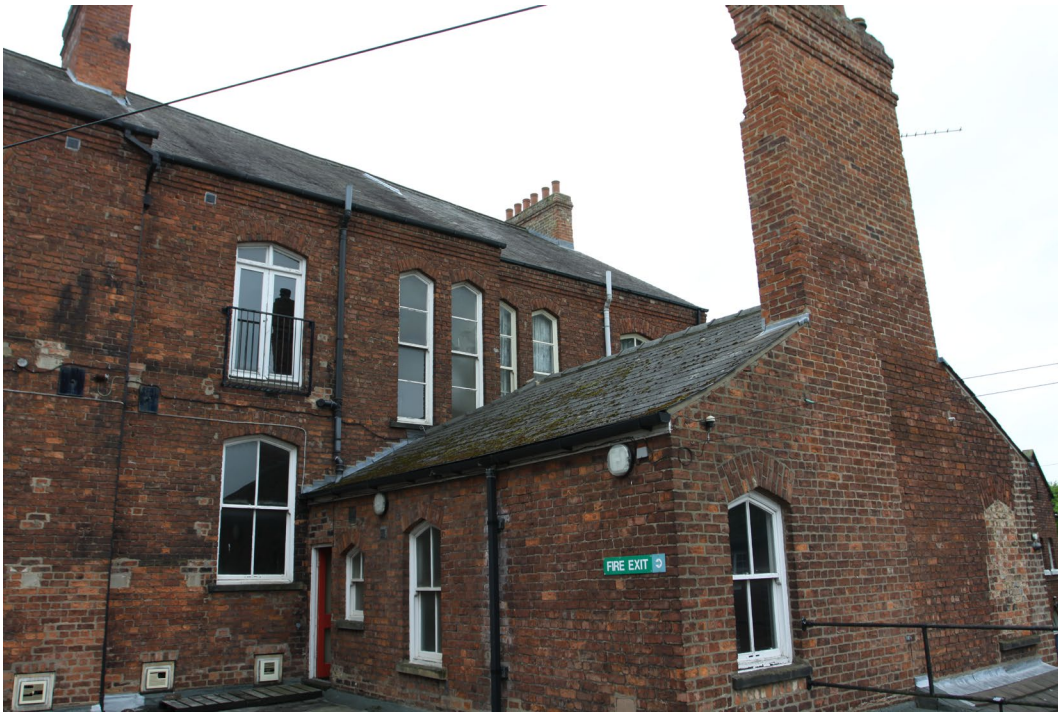
Plate 7 North facing elevation of first floor rear projection, view south-east
