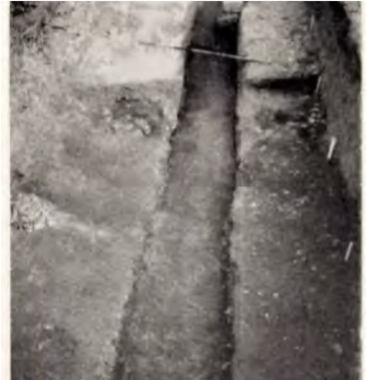
Plate 3. Wenham's Trench 14 from 1953-55 Excavation showing Roman Road 9 (B) and 10 (A).
