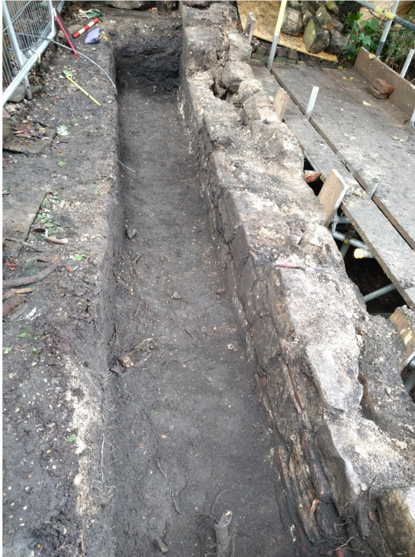
Plate 3 View looking north-east across the wall. The visible wall face is the south-west facing elevation. The CYC trench runs the length of this section of wall.
