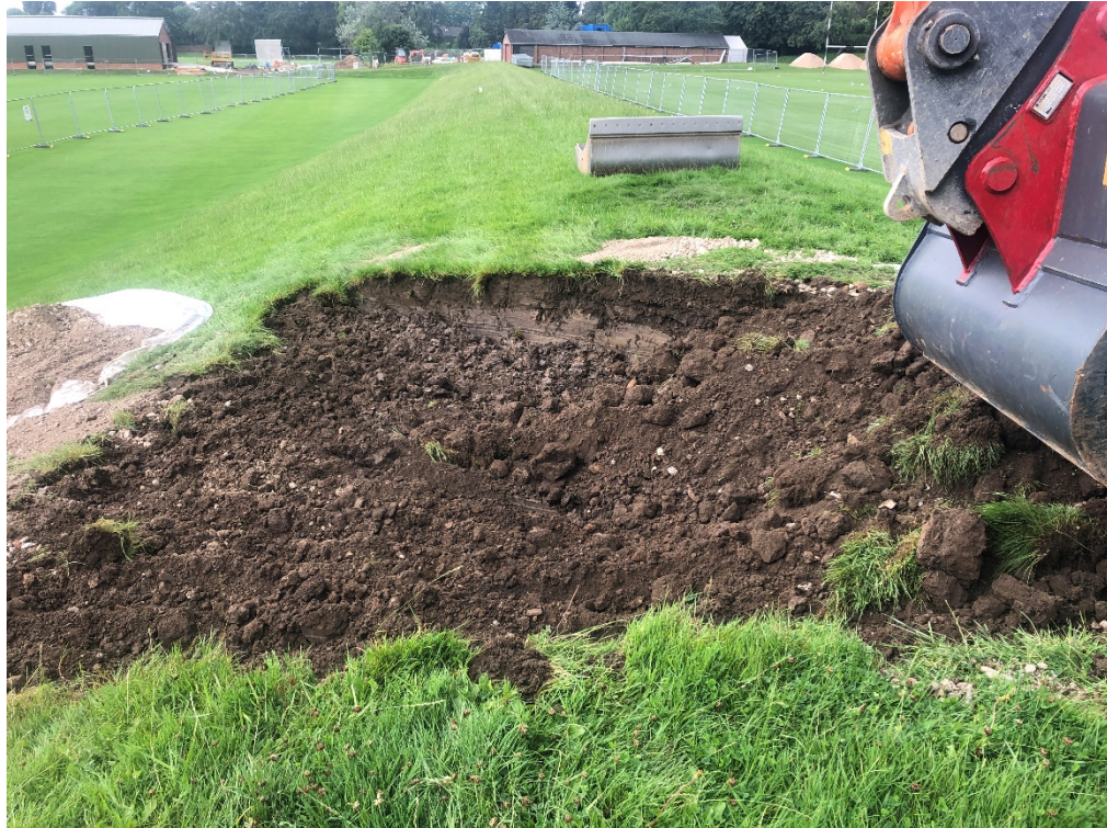
Plate 3 Excavation into the top of the flood embankment.
